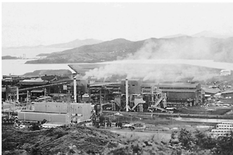
Land and water pollution caused by a nickel smelter on New Caledonia
