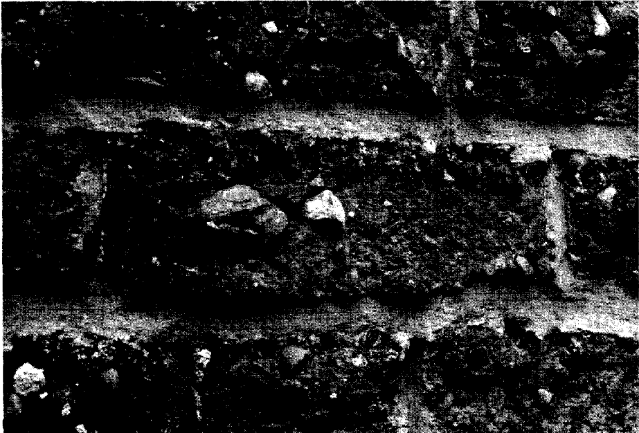
Figure 6.2 Brick ruined by sand-blasting
