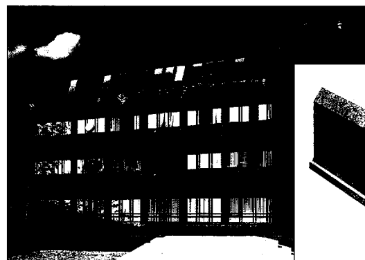
■ 3:4 Plain grey spandrel beams to support external cladding
