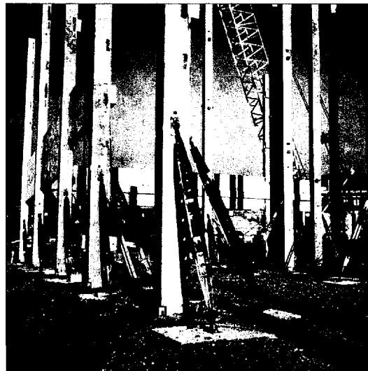
■ 7:7 Propping of frame during erection
