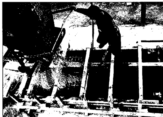
■ 5:6 Placing carefully specified concrete into mould
