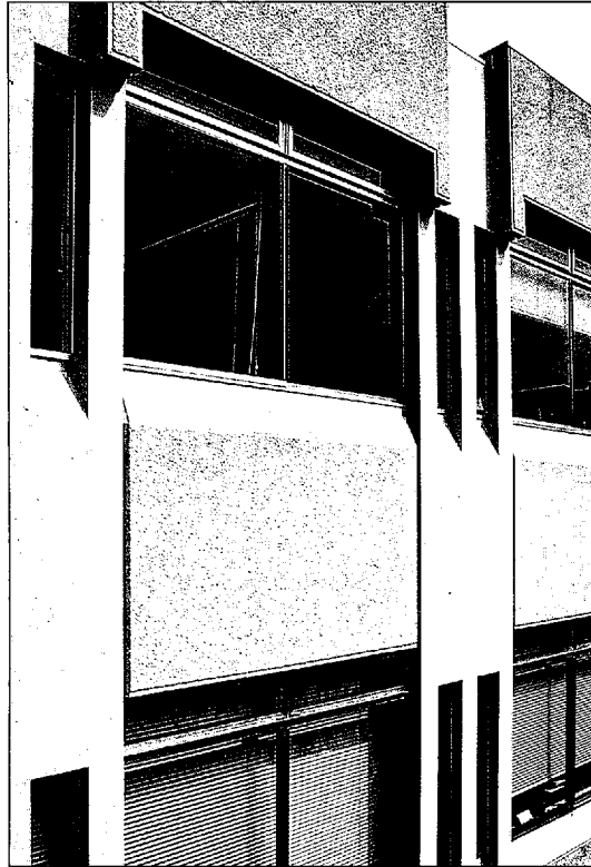
■ 3:6 External loadbearing wall panels produced in high quality visual concrete
