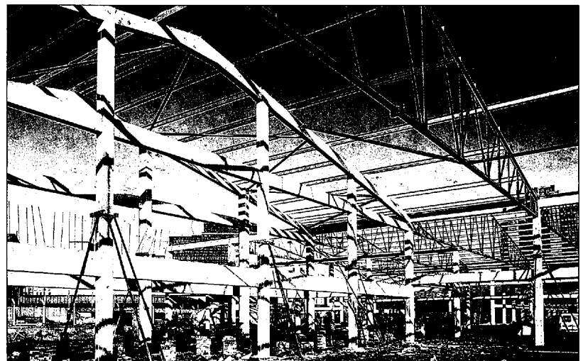
3:10 Precast concrete composite frame
