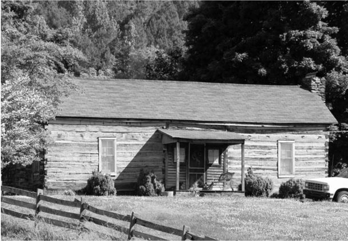
Dogtrot houses, like this one in Giles County, sometimes have the breezeway enclosed to form a central hallway.
