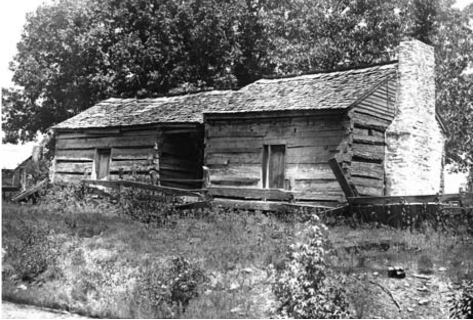
A fascinating house type, the dogtrot features an open breezeway between two pens. This site was near Hohenwald (Lewis County), 12 miles southwest of the Meriwether Lewis National Monument. (Library of Congress, Prints and Photographs Division, Historical American Buildings Survey, HABS TN-36. Photo by A. A. Gustafson, Aug. 1937.)
