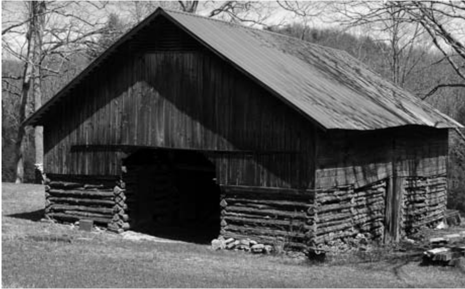
Transverse-crib barns have three or more cribs on either side of an open passageway. This one with saddle-V notches was an accidental discovery near Monterey in Putnam County.
