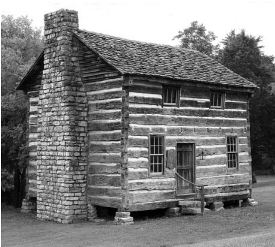
In 1988, the Walker Springs structure was moved 18 miles from its west Knox County site to the Marble Springs John Sevier historic site in south Knox County. Only the larger pen, the west elevation on the original, was reconstructed there.
