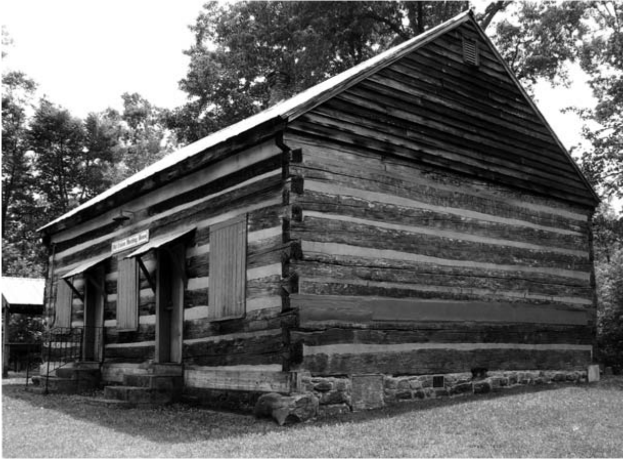
The Old Union Meeting House (c. 1880) in Overton County measures 35 feet 9 inches (east) by 25 feet 11 inches (north) by 35 feet 8.5 inches (west) by 25 feet 9.5 inches (south). The place was built with half-dovetail notches on yellow poplar logs.
