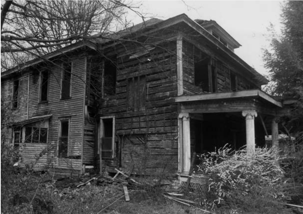
Four-pen houses with log construction are extremely rare. This once opulent home near downtown Columbia in Maury County was razed in 1983. (Courtesy of the Tennessee Historical Commission.)
