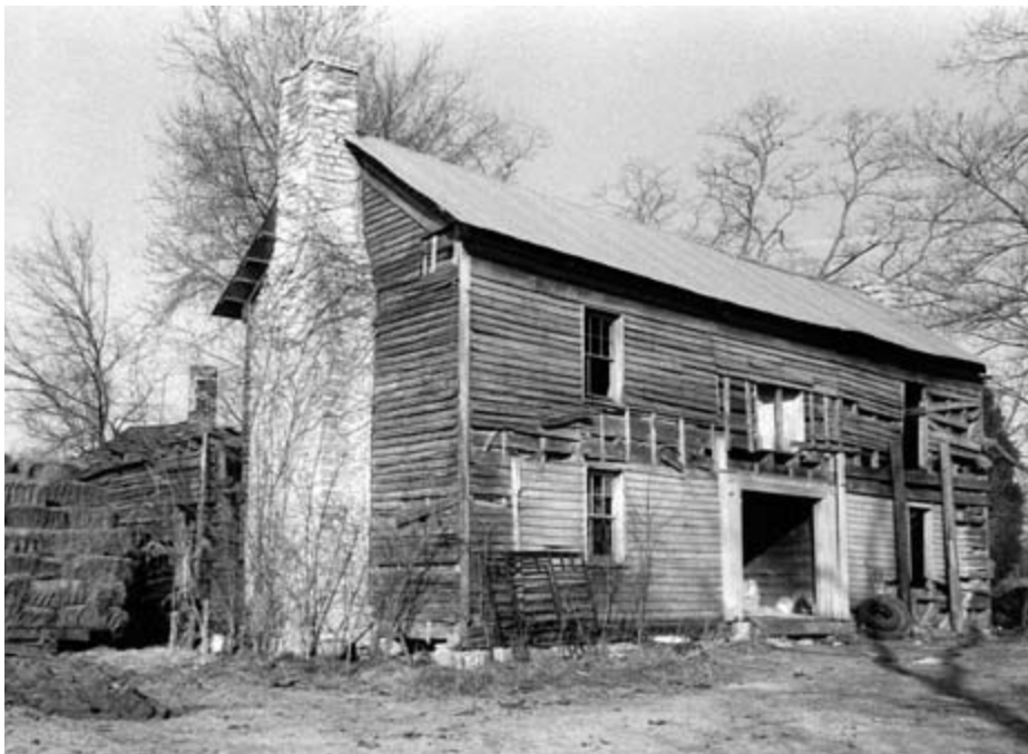
I-houses come in all kinds of conditions. This one, converted into a barn and found in Marshall County south of Nashville, has a dogtrot breezeway entrance—but don't call it a dogtrot house. (Courtesy of the Tennessee Historical Commission.)
