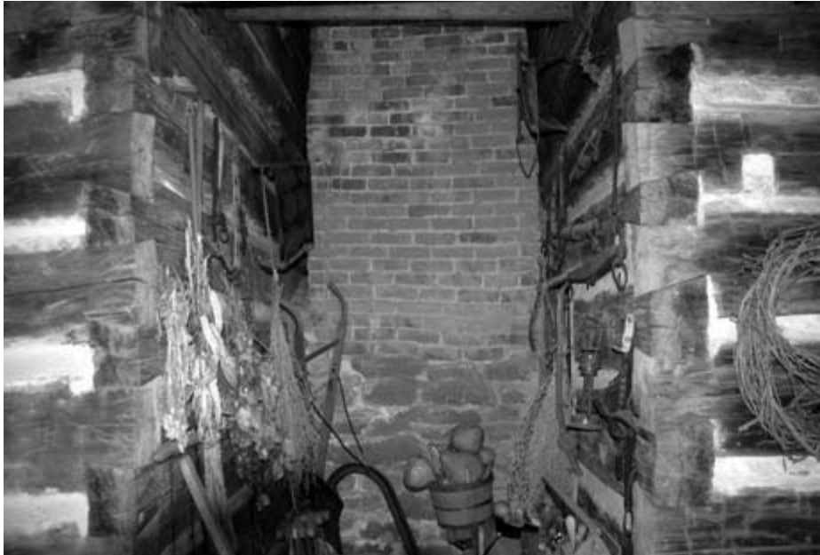
Details of the central chimney in the Hamilton-Tolliver place indicate that limestone was the original construction material before the chimney was later rebuilt with bricks. The chimney area was a storage place, and in some saddlebags, the warm sheltered space made for a convenient chicken coop.
