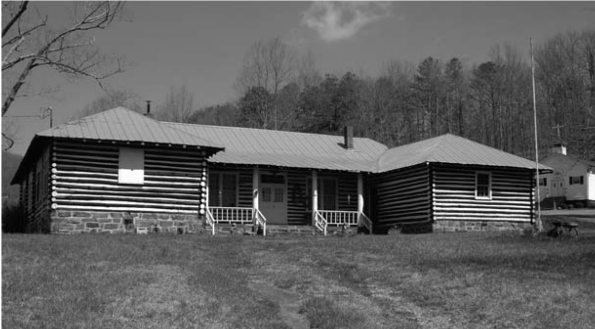
The Stone Mountain School (Poor Valley, Hawkins County) was built in 1940 with saddle notches on round pine logs. The well-preserved building is now a private residence.
