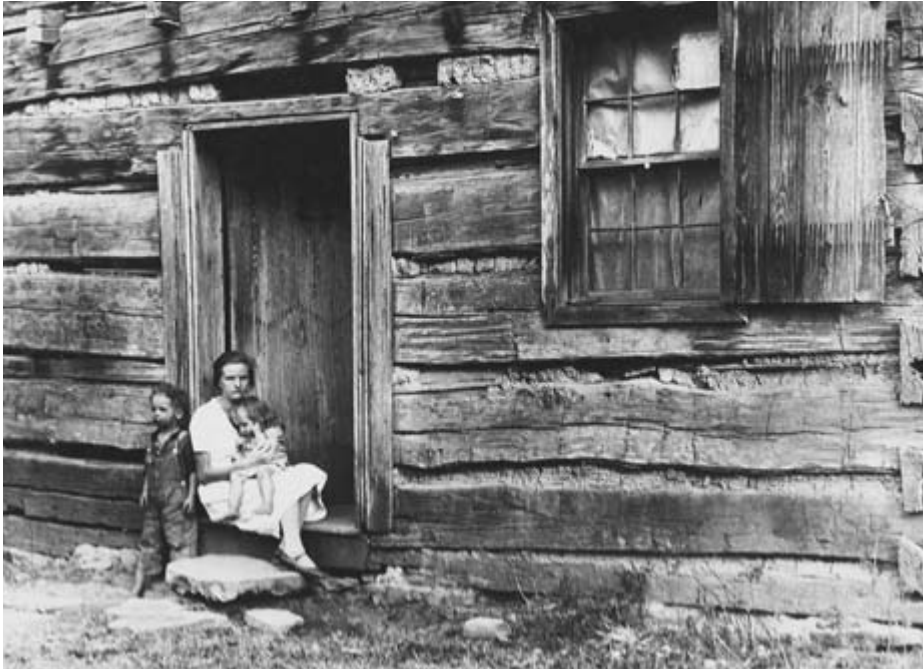
An East Tennessee family and their old log house, October 31, 1933. By 1936, the Tennessee Valley Authority had flooded this site in Union County near Loyston during the creation of the Norris Reservoir, the agency's first hydroelectric dam project. (TVA photo courtesy of the Roy Acuff Museum, Maynardville, TN.)
