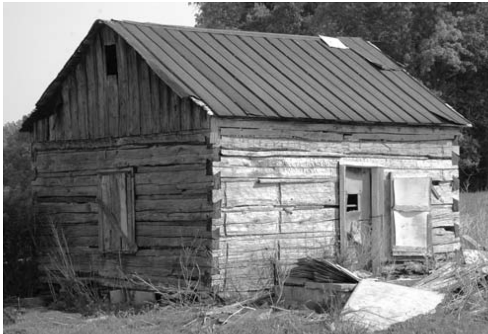
Not much is known of this single-pen with half-dovetail notches on huge yellow poplar logs. Once weather boarded, it had escaped the historical buildings survey in 1982 in Putnam County. The author stumbled upon it twenty-three years later.
