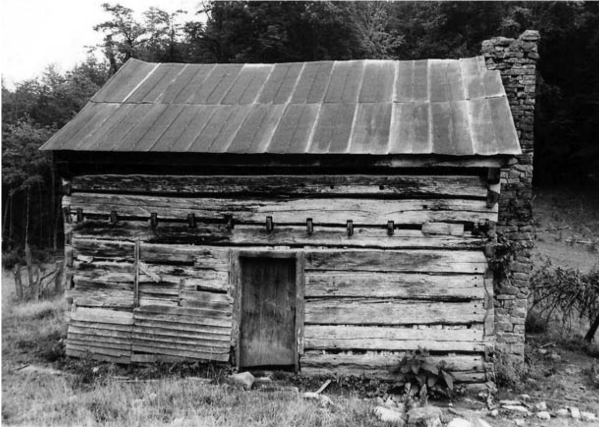
Our image of a typical log cabin might be like this one, a single-pen log house in Grainger County, photographed in 1978.
