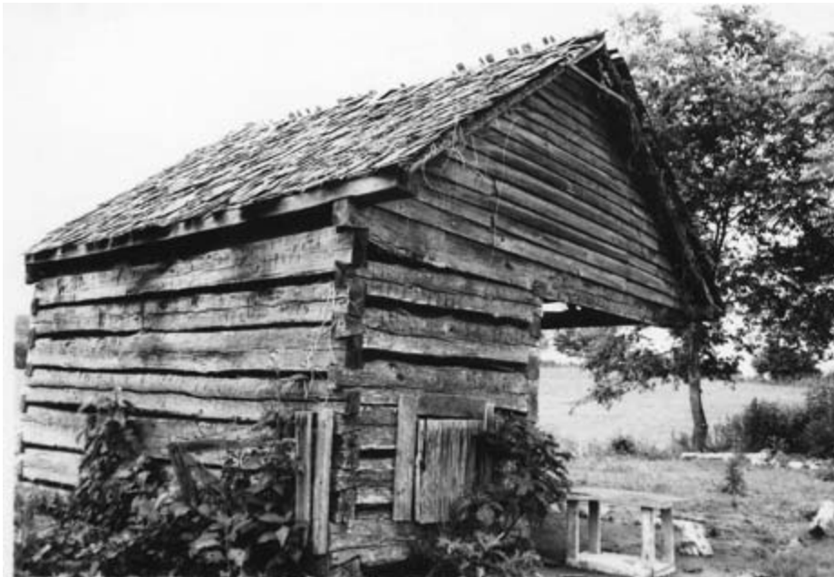
The single-crib with a gear shed, like this one in Grainger County, combines a single-crib (left) with an open shed (right) for implement or gear storage. (Courtesy of the Tennessee Historical Commission.)
