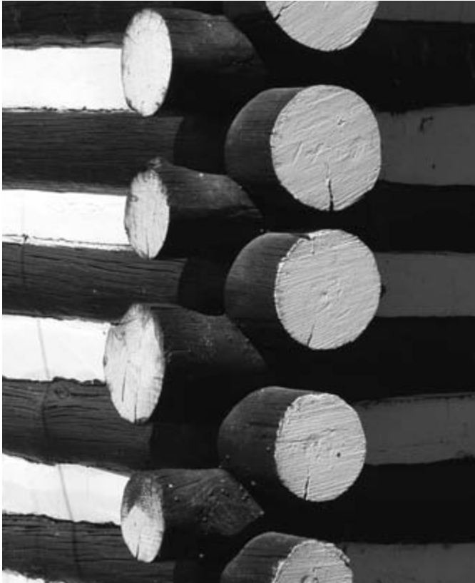
The saddle notch, the simplest of notch types, is made on round logs, usually from pine trees.
