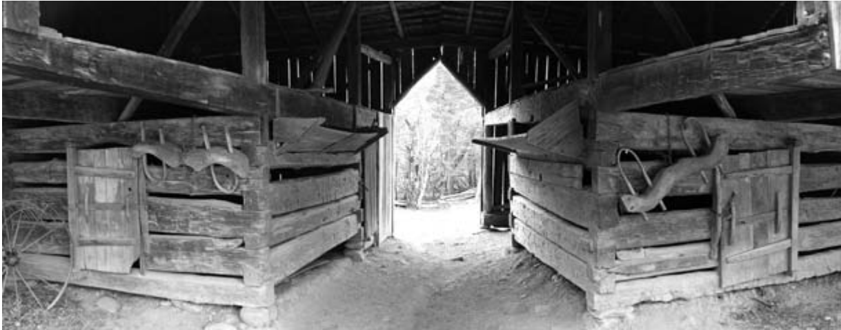
A cantilever barn's foundation consists of two log cribs, as shown in this example from Cades Cove in the Great Smoky Mountains National Park (Blount County).
