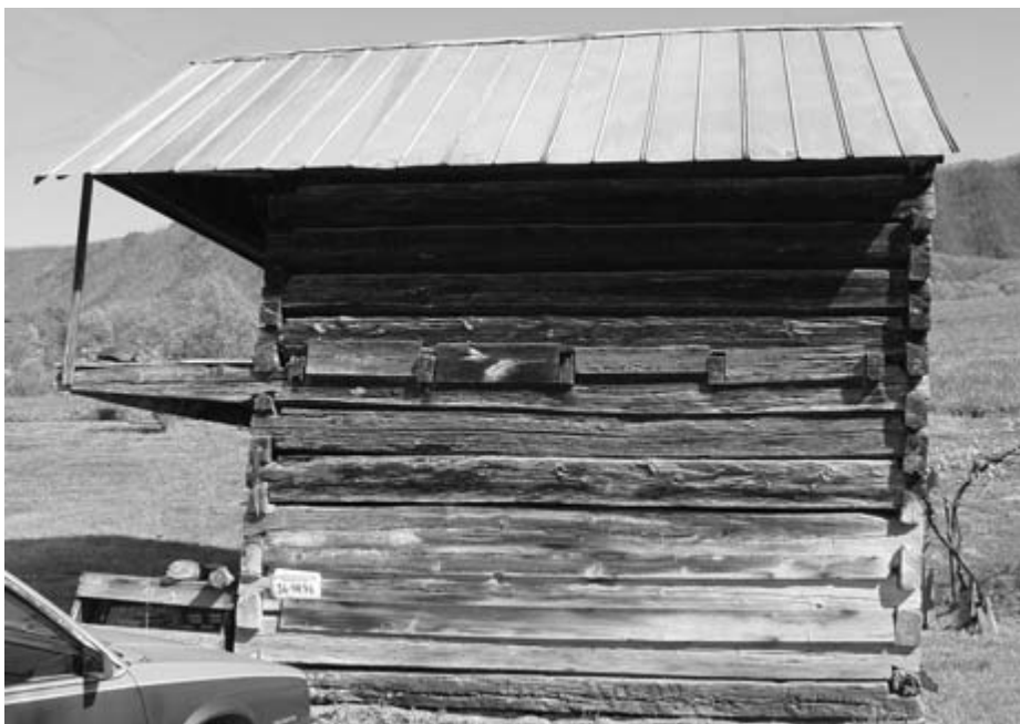
The use of cantilevers was not exclusive to barns. This rare two-level smokehouse with half-dovetail notches on pine logs was built in the 1880s in the "Old Dutch (Deutsch) Settlement" in eastern Sevier County.
