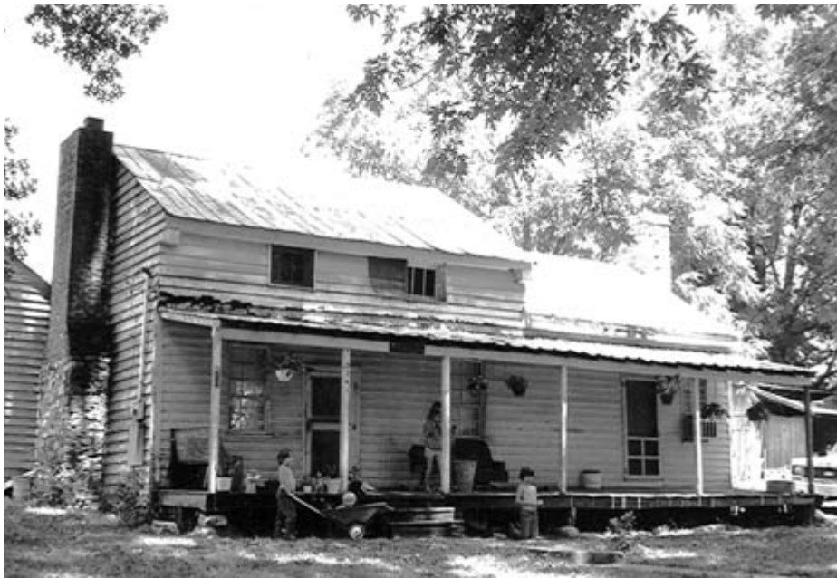
In 1984, the "Walker Springs" place was a weatherboarded Cumberland double-pen house. The home, then occupied, was located on Fox Lonas Road in west Knox County. (Courtesy of the Tennessee Historical Commission.)
