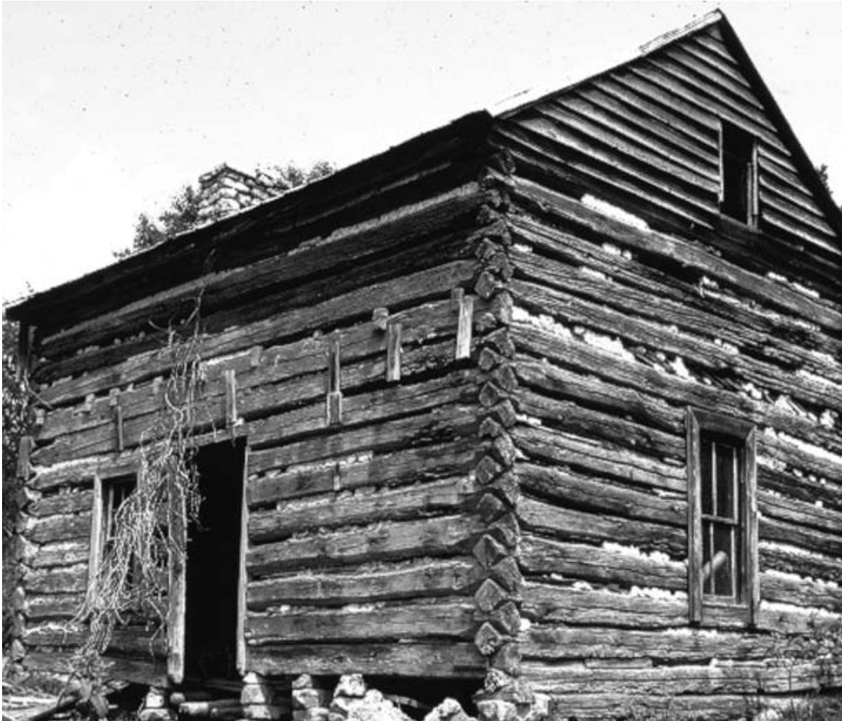
The diamond notch type is as rare as real diamonds. This Grainger County house was razed in 1978.
