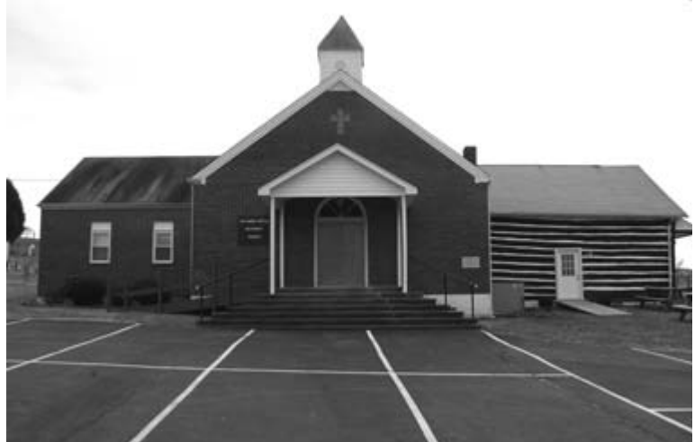
The Old Union United Methodist Church, established in 1834 in Hawkins County, is a testament to historic preservation. The original log unit measures 30 feet by 27 feet and was built with V-notched oak logs.
