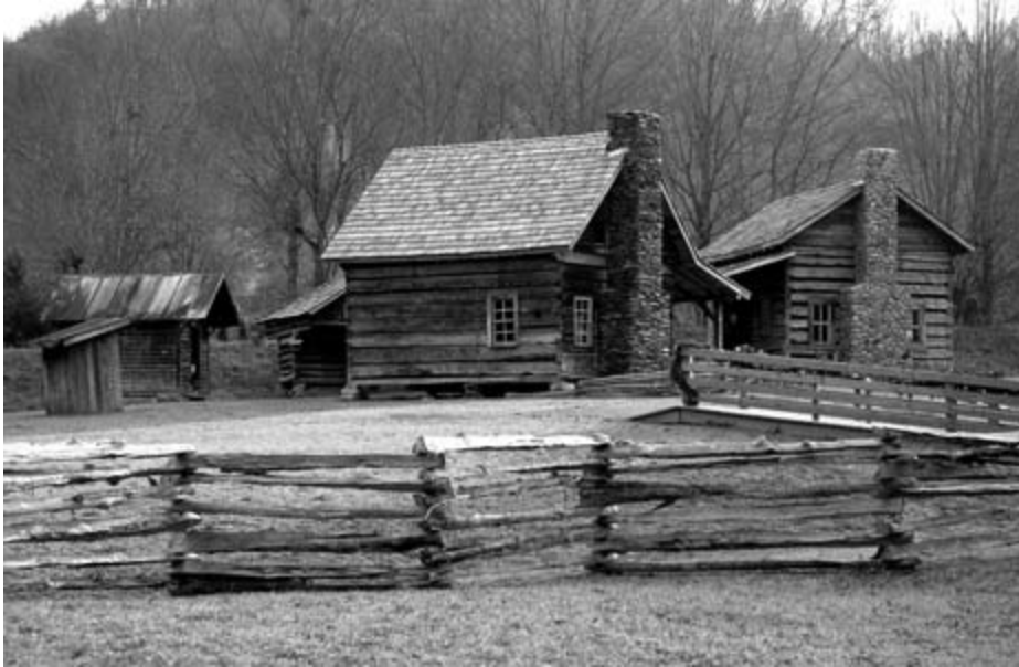
The Great Smoky Mountains Heritage Center, featuring several log buildings and an indoor museum, is located on highway US 321 in Townsend (Blount County).
