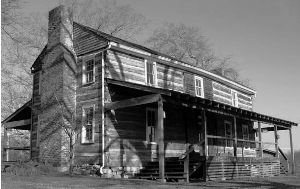
The I-house, like this one in Blount County, is marked by a special formula of room arrangements: two stories tall, two rooms wide, and one room deep.
