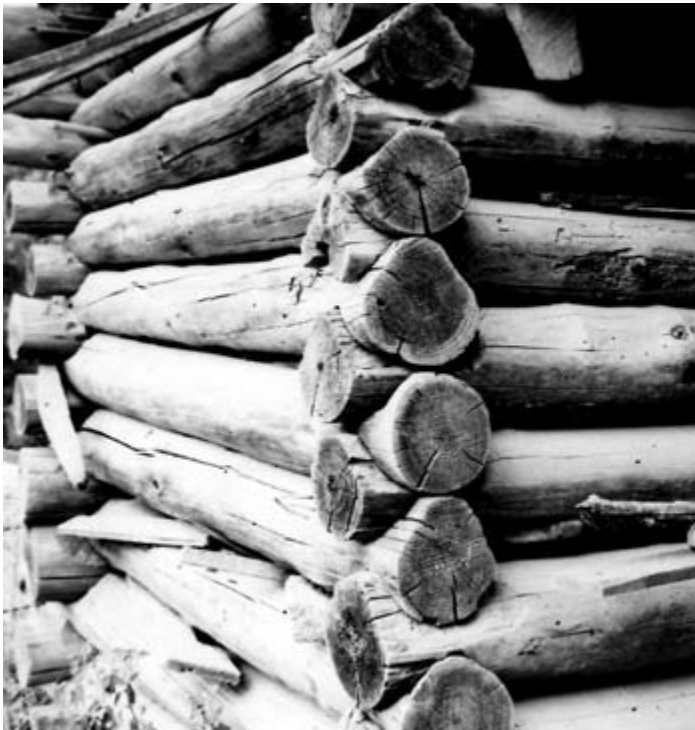
Saddle-V notches have a characteristic “V” cut on top of logs that are left in the round.
