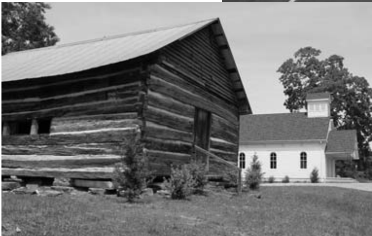
The old log portion of the Okolona Church (Overton County) was built in 1890 with half-dovetail notches on oak logs.
