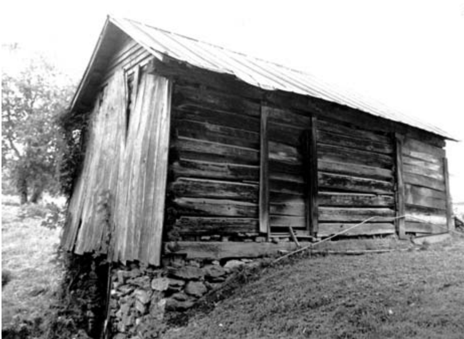
Root cellars, canning cellars, and apple houses have a stone semi-subterranean cellar for long-term food storage. The upper portion, constructed of logs or framed sawn wood, became another storage facility. This example was photographed in Johnson County. (Courtesy of the Tennessee Historical Commission.)
