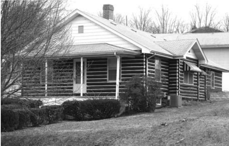
Log bungalow house types are a twentieth-century phenomenon. This one is found in Church Hill, Hawkins County.
