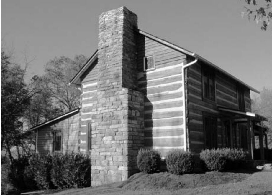
This log house in Hamblen County, featuring V notches on yellow poplar logs, was dated to 1812 with dendrochronology analysis by William M. Reding in 2002.
