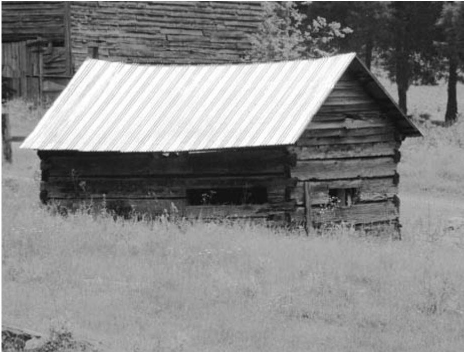
Log blacksmith shops are scarce. This one in Union County is one of the oldest documented log buildings in Tennessee. Dendrochronology determined a date of 1793.
