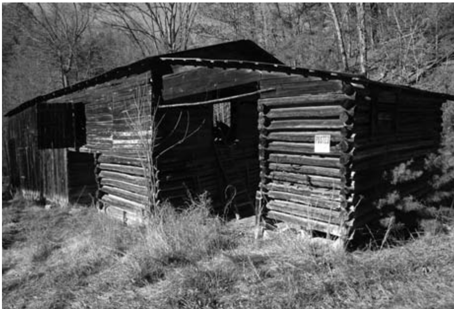
The complex barn on the Meek Williams place includes a log corn crib (right), a large log crib in the center, a framed lumber section (left), and a huge loft above.
