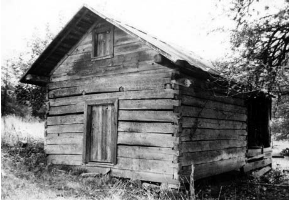
Like this one in Grainger County, granaries were built with tighter walls and raised floors and were used for storing grain other than corn. (Courtesy of the Tennessee Historical Commission.)
