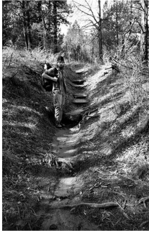
Fig. 13.2. It is impossible to drain water out of this entrenched trail in Zion National Park, USA, due to its low slope alignment angle. Re-routeing is recommended to avoid the need for extensive tread work involving erosion control measures and steps on the existing alignment.
