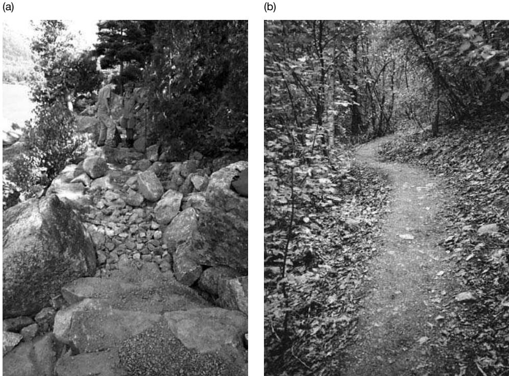
Fig. 13.3. (a) Extensive rockwork and application of gravel are employed to sustain traffic in reconstructing this highly used trail at Acadia National Park, USA. (b) While gravel can be visually obtrusive when initially applied, over time it sinks in and combines with soil to produce the highly resistant tread shown on this trail in Shenandoah National Park, USA.
