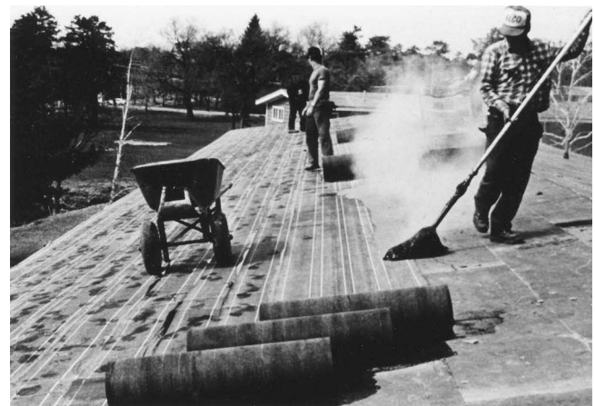
Fig. 11—Felts are laid shingle fashion.
