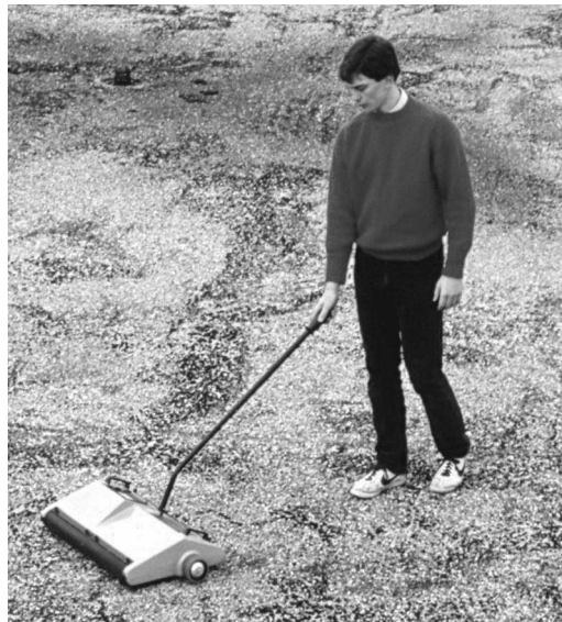
Fig. 57—Surveying a roof with a capacitance meter.
