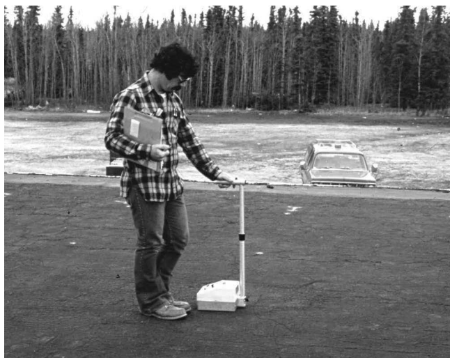
Fig. 56—Surveying a roof with a nuclear meter.
