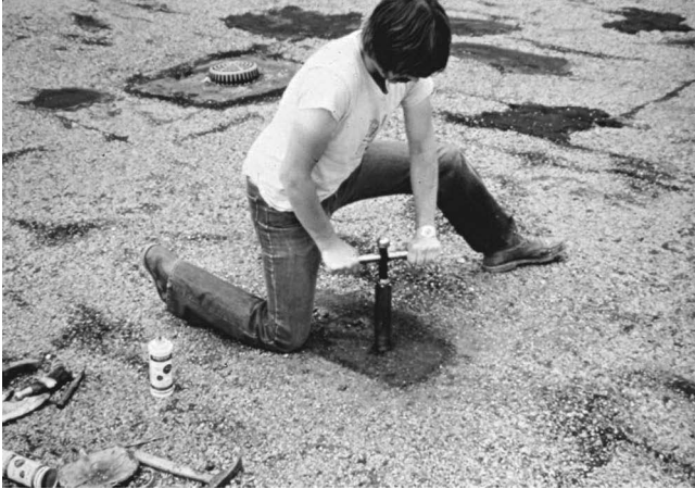
Fig. 62—Obtaining cores to verify a roof moisture survey.
