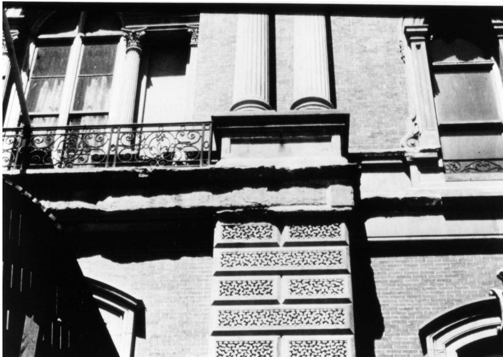
Fig. 11 —Care must be taken in designing repairs using synthetic patching compounds. When large sections of masonry need repair, it is often best to use new sections of masonry instead of synthetic compounds. Moisture, which moves naturally within a wall, can be trapped by vapor impermeable materials, leading to further decay of the historic substrate, as seen in this epoxy repair of the balcony. Photo: NPS files.
