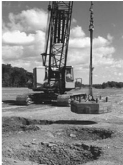
FIGURE 5.9 Dynamic compaction. (Photo courtesy of Terra Systems, Inc.)
