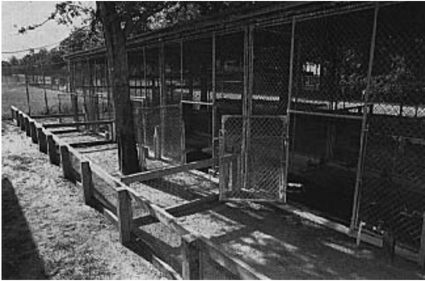
FIG 46.4 Facilities that are designed with individual enclosures, but a common pool, increase the risk of disease transmission. Preferably, each enclosure should have its own pool that can be drained into a common ditch outside the enclosure (1994 Busch Gardens Tampa. All rights reserved.).
