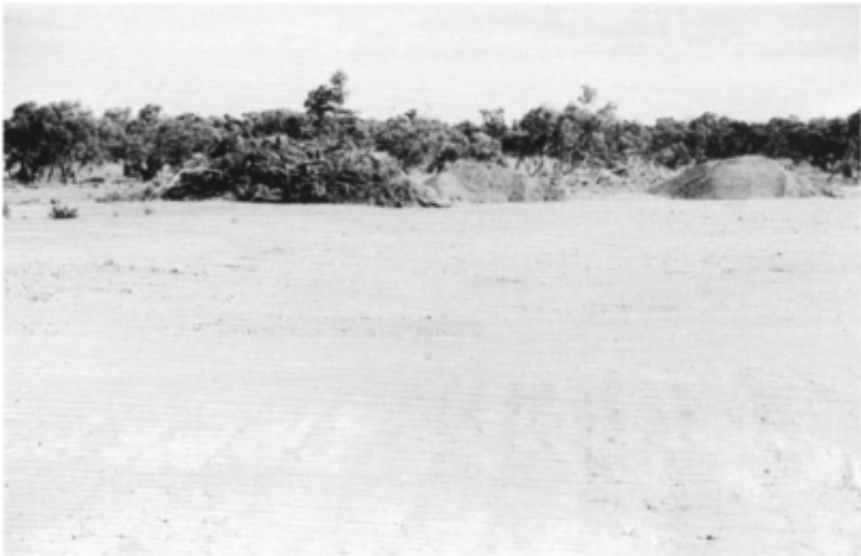
Figure 1.2 Preparing for quarry restoration in a north Queensland ferricrete (laterite) roadbase pit. At this stage the ferricrete surface has just been exposed; topsoil and vegetation mulch are stockpiled on the left, thin subsoil overburden in the other two mounds. Low soil fertility and low rainfall inhibit site rehabilitation, and the shallow depth (about 1.5 m) of the ferricrete means that a large area must be stripped to obtain the required volume of gravel. Usually the time interval between stripping and restoration is 6–12 months.
