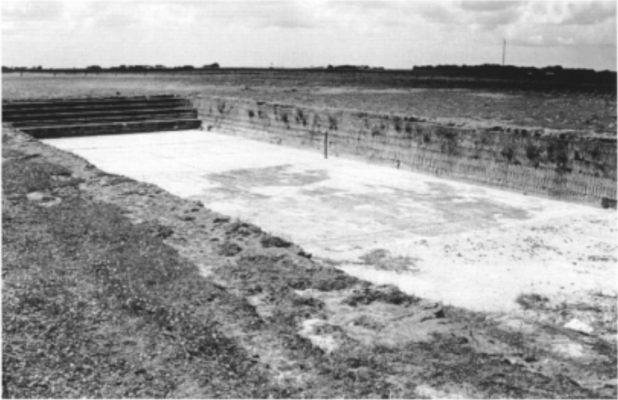
Figure 21.2 An unusual example of quarry rehabilitation—as a tennis court, near Mount Gambier, South Australia. The sunken aspect also provides protection from winter winds! The Gambier Limestone here is a soft, non-abrasive rock that is cut as dimension stone.
