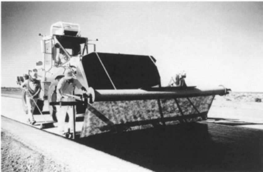
Figure 11.5 Experimental geofabric seal placed directly on an expansive clay subgrade (i.e. no pavement courses) in western New South Wales. This is an attempt to provide an all-weather surface for a lightly trafficked road at minimal cost. The aim is to keep the subgrade at a constant moisture content with a good-quality seal; the geofabric both reinforces the seal and resists any heaving or shrinkage that may occur. (Photo: M.Sutherland.)
