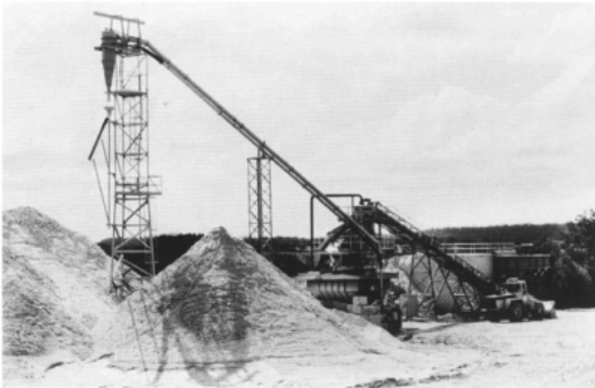
Figure 6.10 Dewatering hydrocyclone (conical object at the top of the tower), Calga, New South Wales. The lower (high pressure) of the inclined twin pipes carries the feed slurry and the upper pipe drains off silt-laden water to tailings dams. Two product stockpiles are visible.
