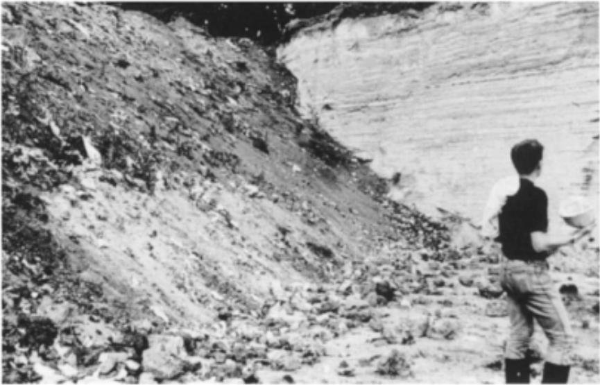
Figure 19.3 Conjunctive use of a quarry site, Reading, UK. As Eocene sands are extracted to the right (outside the photograph), the pit is being backfilled with waste (left). (Photo: J.H.Whitehead.)
