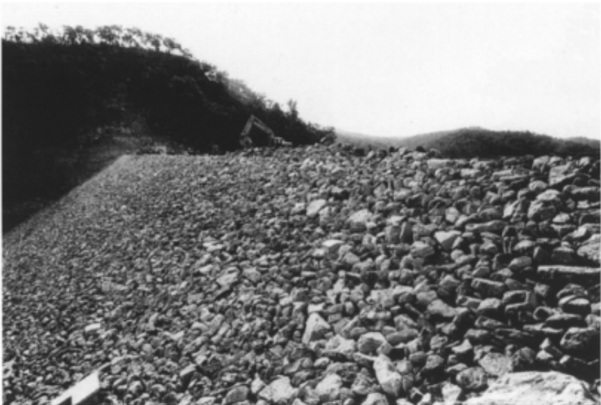
Figure 12.5 Slope protection boulders on downstream face of Mangrove Creek Dam, a soft rockfill CFR dam north of Sydney. The maximum size of this rip-rap is about 1.5 m. (Photo: D.F.Branagan.)
