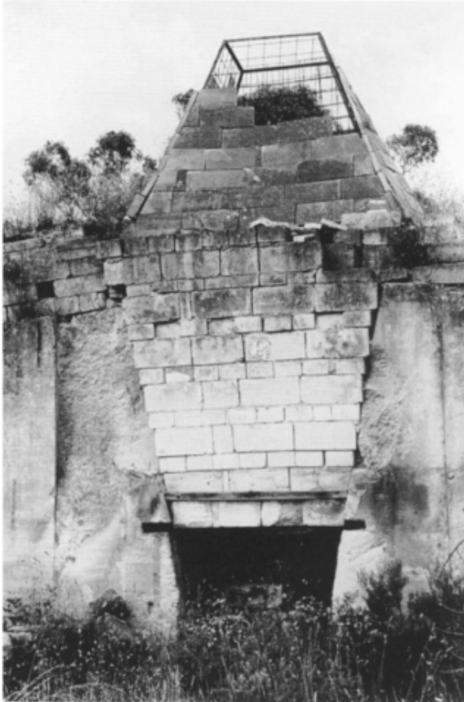
Figure 1.6 Quarrying heritage—a limestone kiln, now abandoned, built into a rock face near Mount Gambier, South Australia. The kiln was built out of offcuts from Gambier Limestone used primarily as sawn dimension stone.
