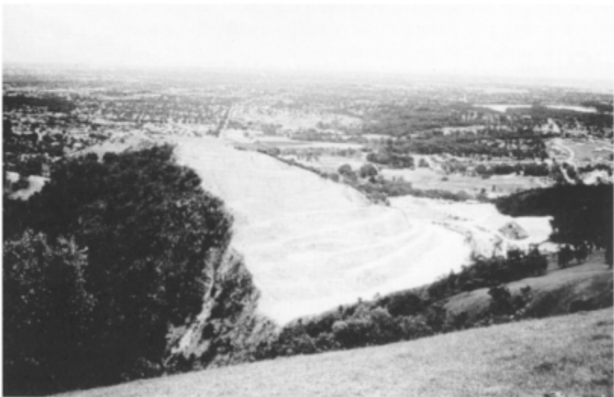
Figure 19.4 Quartzite quarry face oriented so as to be unseen from the eastern suburbs of Adelaide, South Australia; this arrangement also radiates airblast away from most residents. This site is located along the sensitive Hills Face zone, where quarrying is now subject to severe environmental controls.
