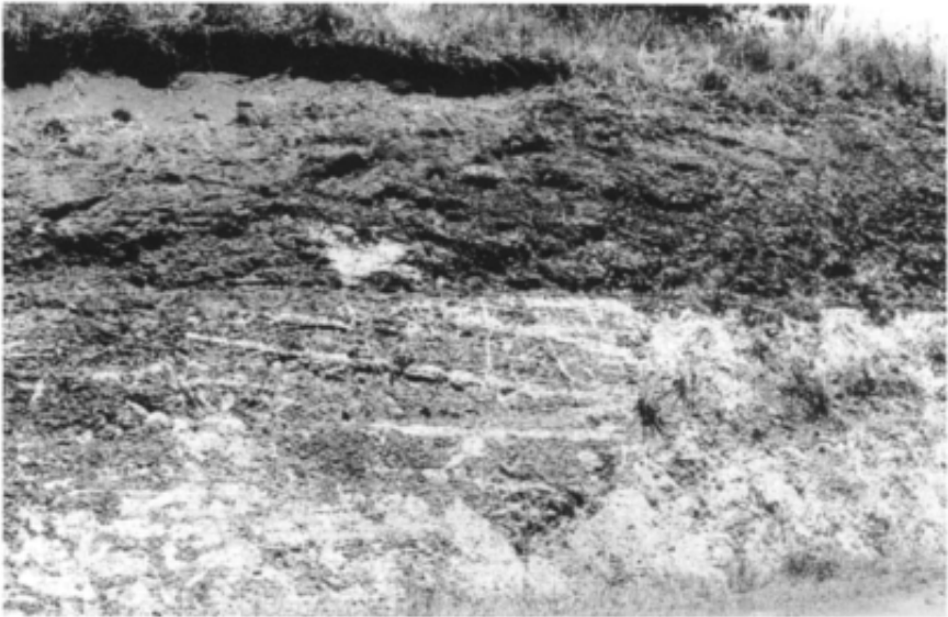
Figure 4.5 Laterite profile near Casino, New South Wales, showing ferricrete horizon (about 1 m thick) at top and mottled zone beneath. In extracting this material about 0.5 m of topsoil would first be stripped, and the ferricrete ripped, blended and stockpiled in the pit. The pit floor would be located at the top of the mottled zone.
