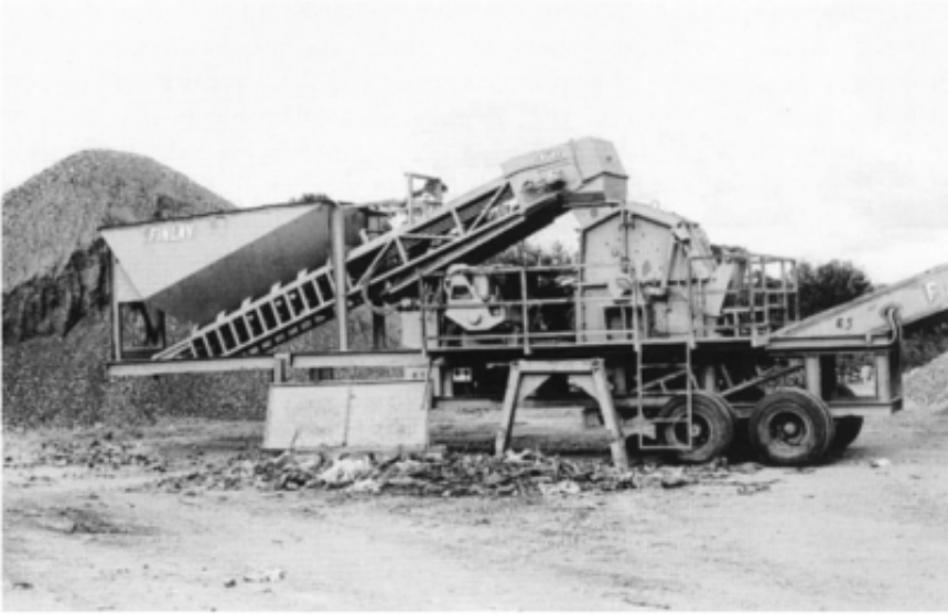
Figure 5.9 Small portable impact crusher being used for comminution of demolition rubble. Note hopper and elevating feeder conveyor, and product stockpile at rear. The right-hand conveyor feeds to a screening unit.
