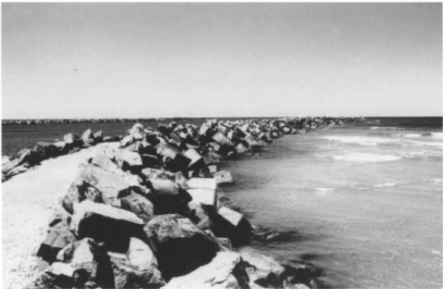
Figure 13.7 River-mouth breakwater, Yamba, New South Wales. The primary armour here is sandstone, supplemented by 10 tonne concrete blocks to the extent of about 5%.
