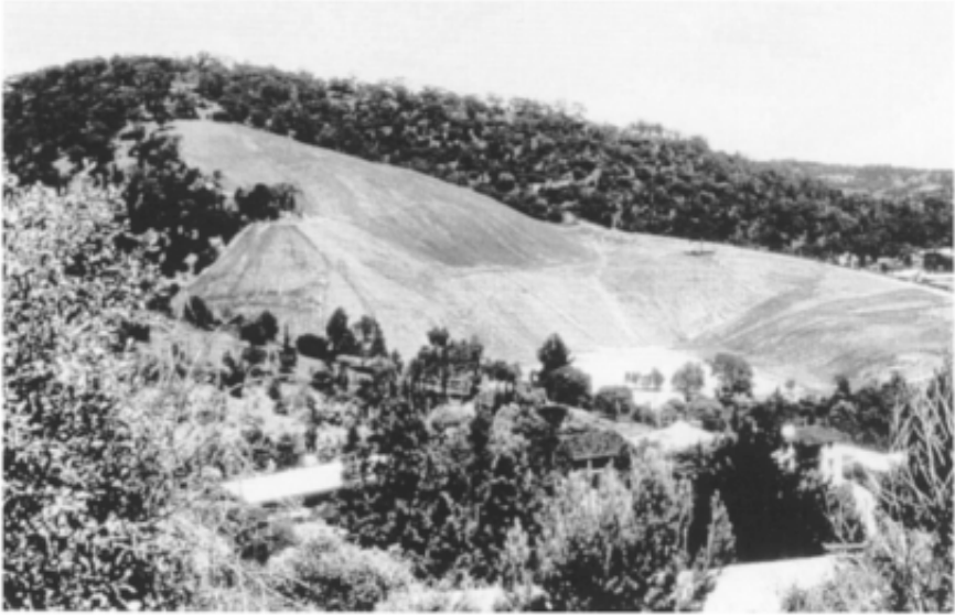
Figure 21.6 A former quartzite quarry so successfully reshaped that former benches are almost invisible, near Adelaide, South Australia. Grasses have been planted, but some sheet erosion and sedimentation (at pit floor) are visible, and the native treescape has not yet been reproduced. The site was recycled for housing and recreational uses.
