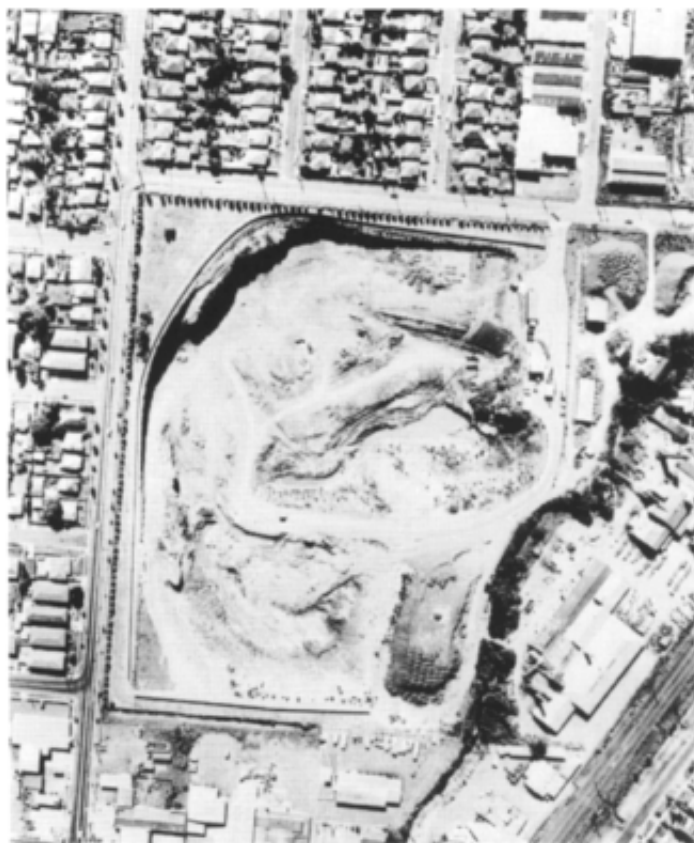
Figure 16.8 Brickworks (lower right) and Ashfield Shale pit, western Sydney. The pit is about 300 m square and has since been backfilled with garbage and recycled as a public park. Note the suburban encroachment on two sides, though the brickworks managed to operate for several decades after these houses were built. (Photo: P.Dupen.)
