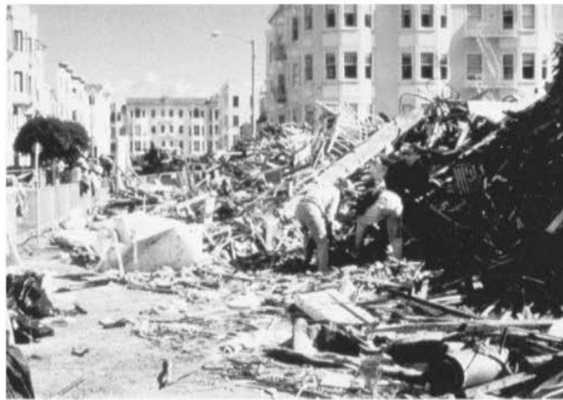
► FIGURE 8.33 Rubble from collapsed building on Jefferson Street in the Marina District of San Francisco resulting from the Loma Prieta earthquake. Source: D. Perkins; photo courtesy of U.S. Geological Survey.
