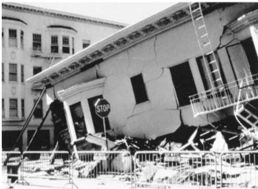
▲ FIGURE 8.61 The third story of a three-story building in the Marina district of San Francisco. The first and second stories collapsed due to ground shaking and liquefaction. Source: D. Perkins; U.S. Geological Survey.
