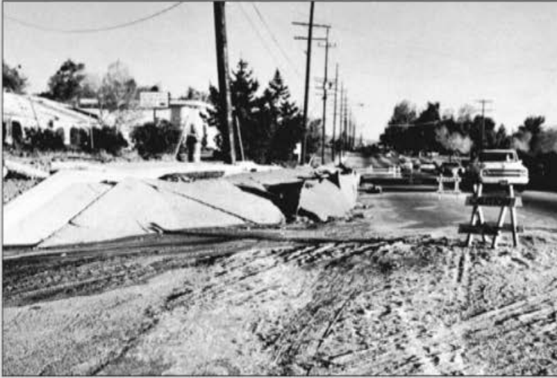
◀ FIGURE 8.77 Damage to highway by surface rupture from the 1971 San Fernando, California, earthquake. Source: Photo courtesy of U.S. Geological Survey.
