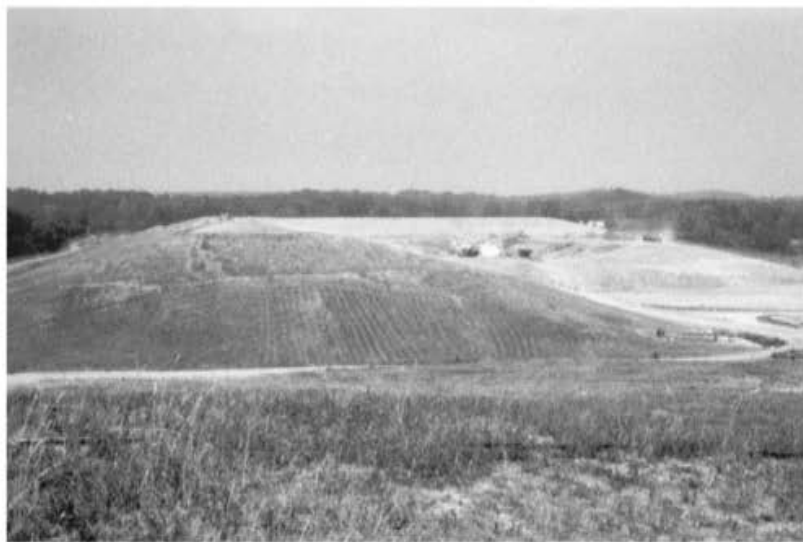
◀ FIGURE 12.9 Photo of a waste cell being filled in a landfill of the area type in southwestern Michigan. Source: Photo courtesy of the author.
