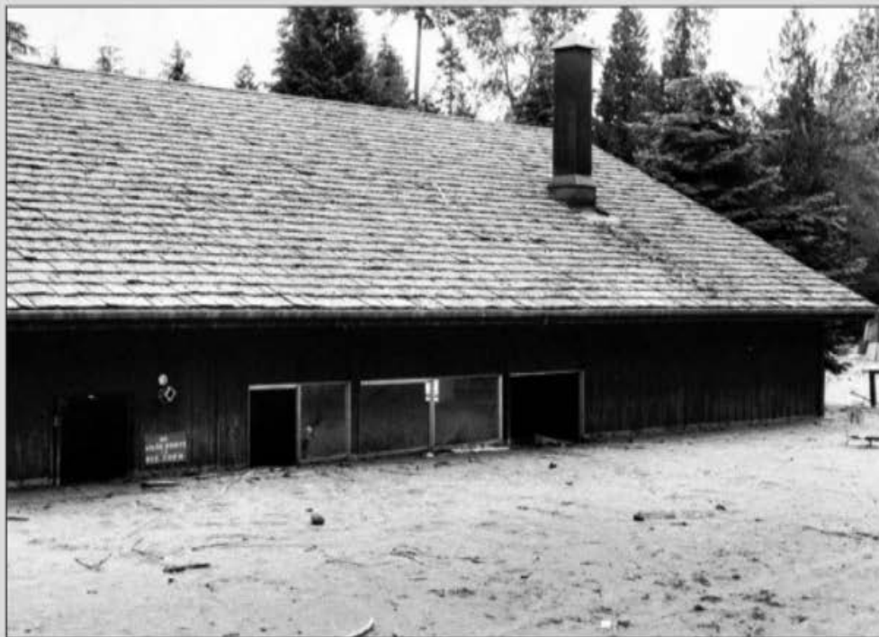
▲ FIGURE 4.43 Building partially buried by lahar deposits, North Fork Toutle River valley. Source: R. L. Shuster; photo courtesy of U.S. Geological Survey.
