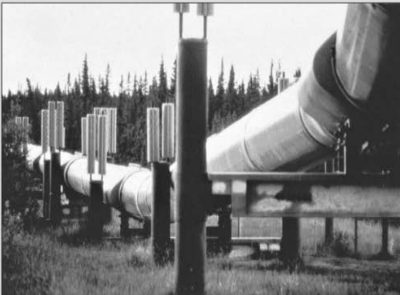
◀ FIGURE 16.52 Photo of aboveground section of pipeline near Paxson, Alaska. Source: Photo courtesy of Glenn Oliver.
