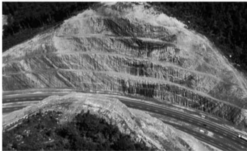
▲ FIGURE 8.4 Exposure of a syncline in Devonian shales and sandstones in a road cut through Sideling Hill along I-68 in western Maryland. The roadcut is approximately 255 m in height. Source: Photo by Paul Breeding; courtesy of Maryland Geological Survey.
