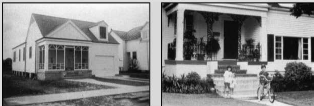
▲ FIGURE 10.51 Subsidence of organic soils in New Orleans after drainage. The photo on the left shows the house built on pilings just after construction in 1941. The photo on the right shows the same house in 1992. Front-porch steps were added over the years as the ground surface subsided. Source: Photo courtesy of J. O. Snowden.
