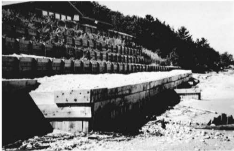
► FIGURE 15.54 Tiered seawall designed to prevent erosion along the shore of Lake Michigan. Source: Photo courtesy of the author.
