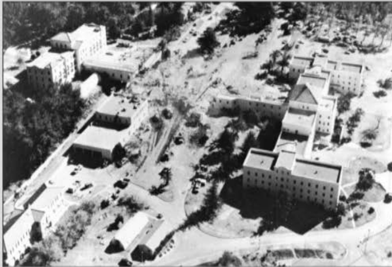
◀ FIGURE 8.78 Cleanup following collapse of Veterans's Hospital during the San Fernando earthquake. Forty-five people were killed. Source: Photo courtesy of U.S. Geological Survey.
