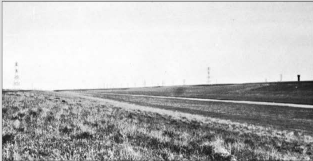
▲ FIGURE 14.57 The Red River floodway. Source: Photo courtesy of the author.
