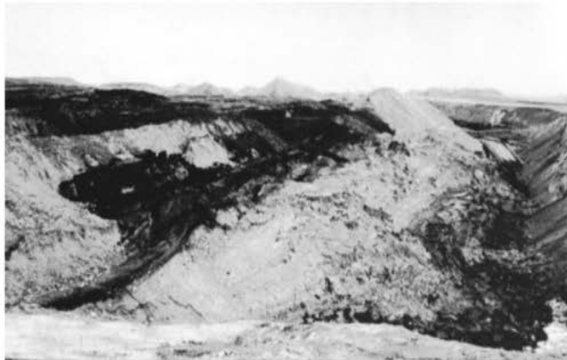
◀ FIGURE 13.37 Slumping of surface mine spoils into a newly excavated mine pit was caused by piling too much spoil material at the edge of the pit. Source: Photo courtesy of the author.
