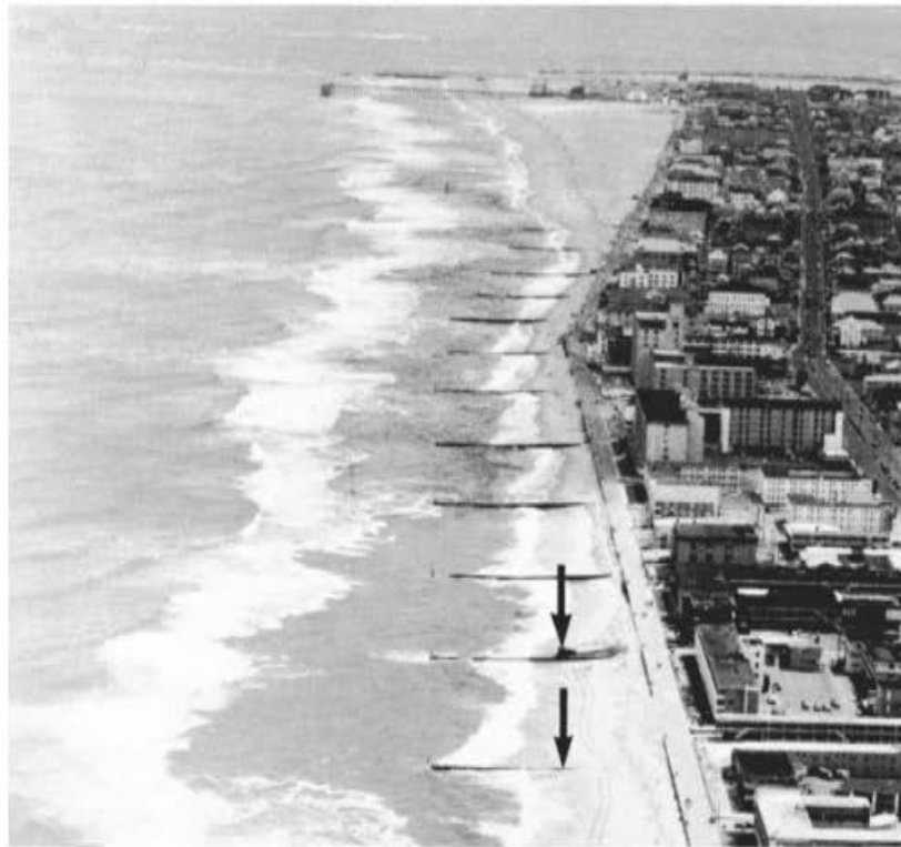
► FIGURE 15.55 Aerial view of groin field along the Maryland coast. Arrows show individual groins in the foreground. Source: R. Dolan; photo courtesy of U.S. Geological Survey.
