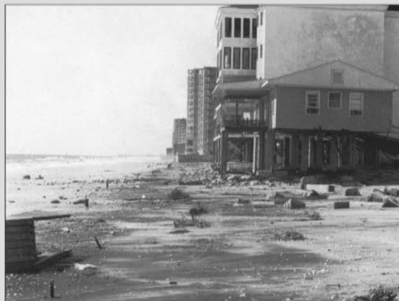
▲ FIGURE 15.49 Flat storm beach produced by erosion of sand and damage to buildings at Surfside Beach, near Charleston, S.C. by Hurricane Hugo. Source: From R. H. Willoughby and P. G. Nystrom, Jr., 1990, Some effects of Hurricane Hugo on shoreline landforms, South Carolina, Columbia, September 21–22, 1989, South Carolina Geology , 33:39–58.
