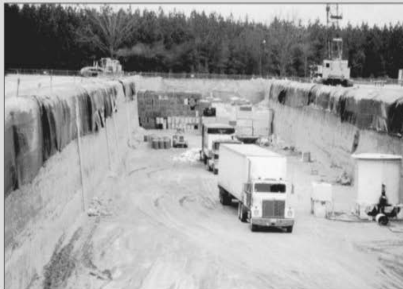
▲ FIGURE 5.47 Active trenches containing low-level radioactive waste at the Barnwell, South Carolina, site. Source: Photo courtesy of the author.
