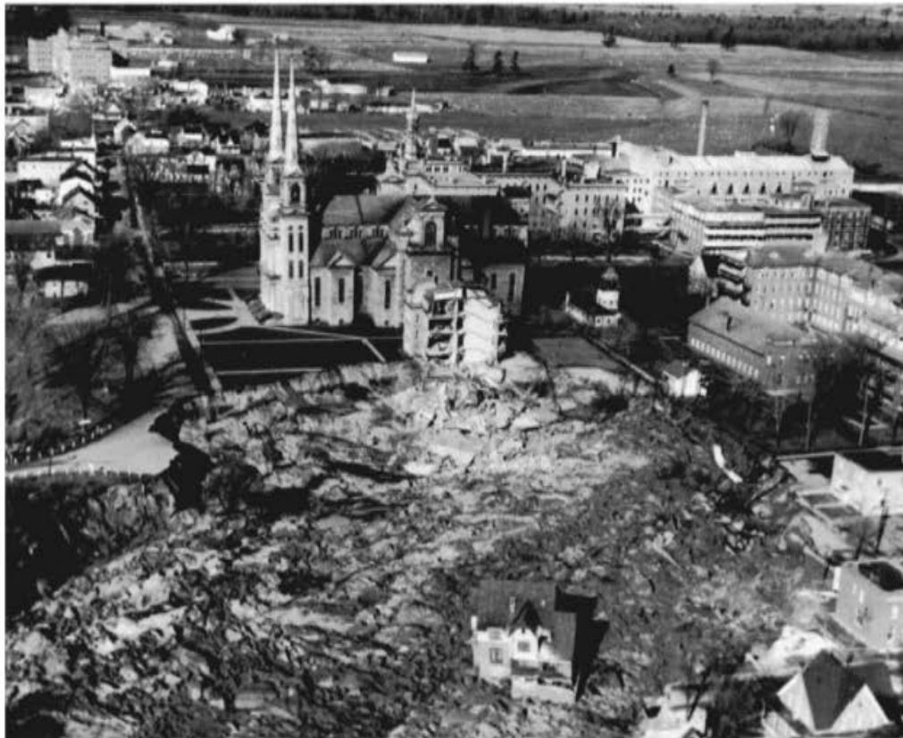
▲ FIGURE 13.16 Aerial view of the Nicolet, Québec, lateral spread of 1955. Buildings and trees were rafted along in an upright position. Source: Henry Laliberté; photo courtesy of Gouvernement du Québec, Ministère de l'Environnement.
