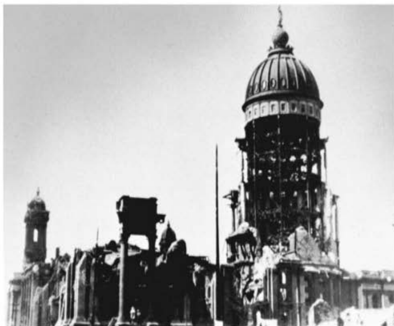
◀ FIGURE 8.32 Damage to the San Francisco City Hall by the 1906 earthquake. Source: W. C. Mendenhall; photo courtesy of U.S. Geological Survey.
