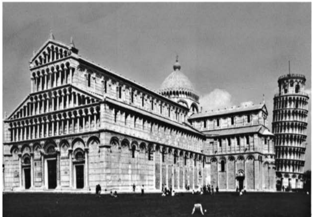
▲ FIGURE 10.23 The Leaning Tower of Pisa (tower at right), whose tilt is the result of nonuniform consolidation beneath the structure. Source: Photo courtesy of the Italian Government Travel Office, E.N.I.T.
