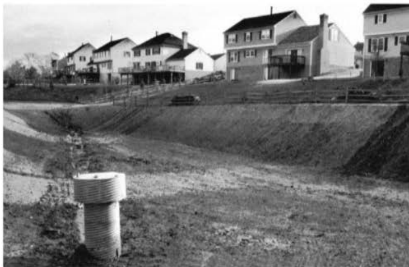
▲ FIGURE 9.31 A sediment detention basin used to trap sediment in an urban area. Source: Photo courtesy of USDA Natural Resources Conservation Service.
