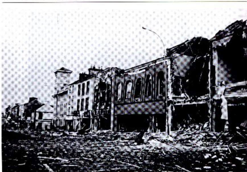
Plate 8. The disintegration of buildings in Bangor, N. Ireland due to blast loading produces fragments that could inflict serious injuries. Photograph courtesy of Kirk McClure Morton
