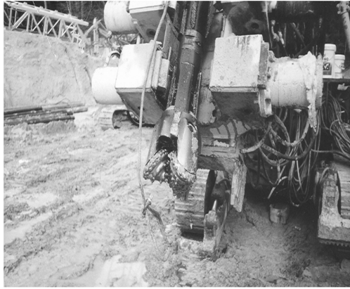
Figure 12.24. Photograph showing auger drill for micro-piles.
