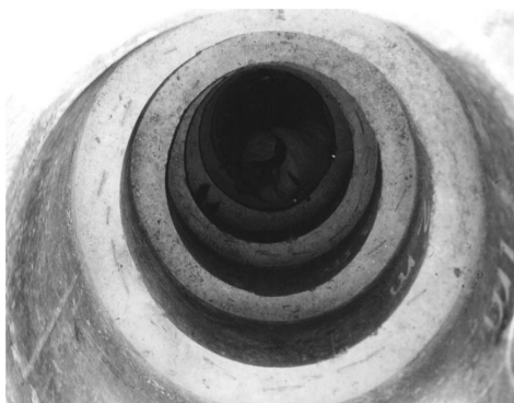
Figure 7.1. In-situ concrete linings of a hand-dug caisson.
