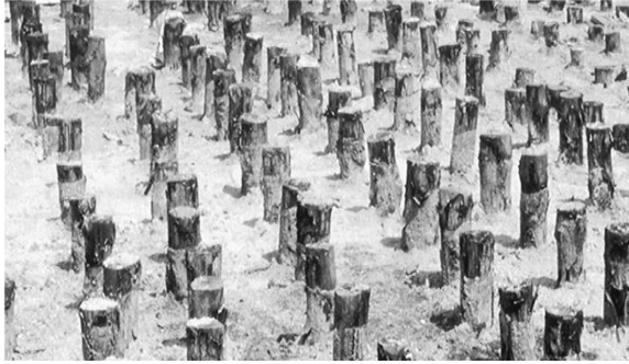
(a) Bakau piles
