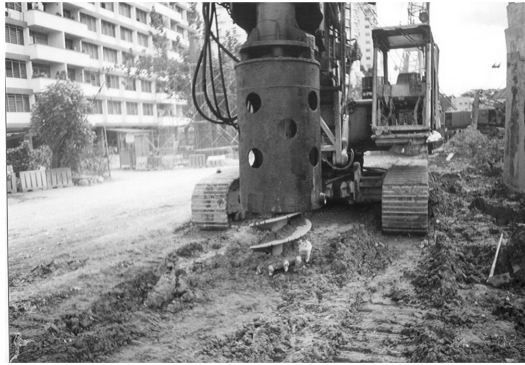
Figure 6.5. Photograph of a drill rig showing an auger drill at the tip.
