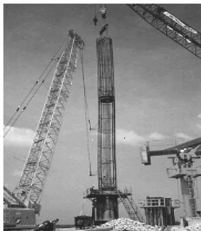
(b) Photograph of the Osterberg load test. ( www.loadtestasia.com/about.htm )
