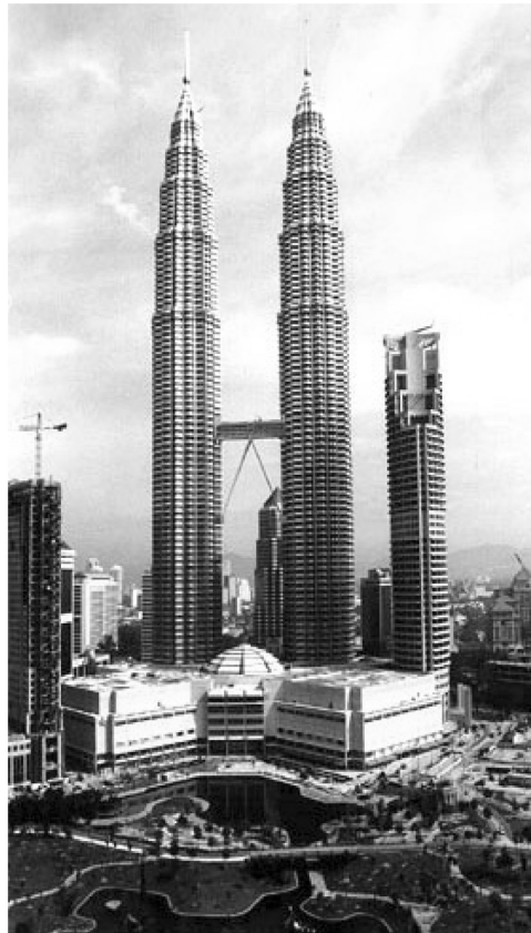
Figure 6.12. The Petronas Twin Tower, Kuala Lumpur, Malaysia.
