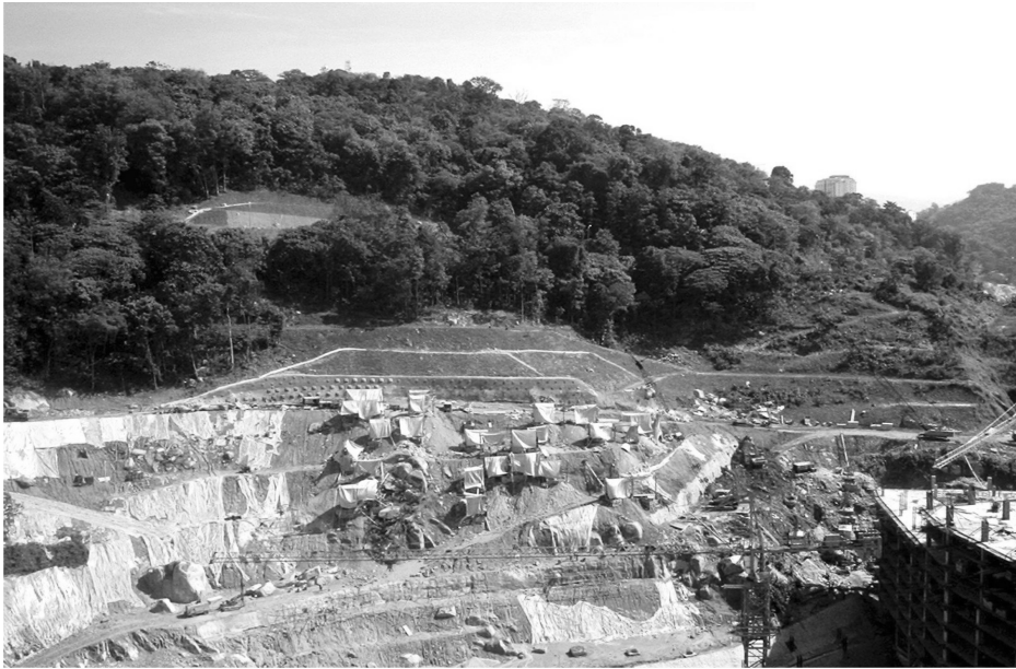
Figure 7.3. Hand dug caissons for a hill site development.
