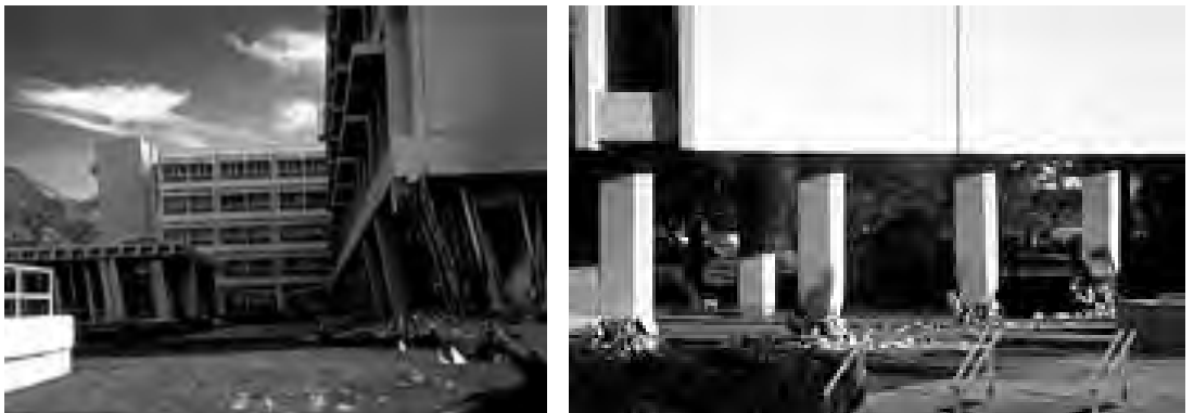
FIGURE 14.3 Collapse of building due to excessive deformation in San Fernando earthquake, 1972.
