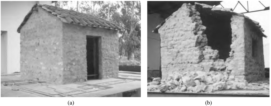
FIGURE 31.7 (a) Model 4 under shock test (b) Out-of-plane failure of Model 4.
