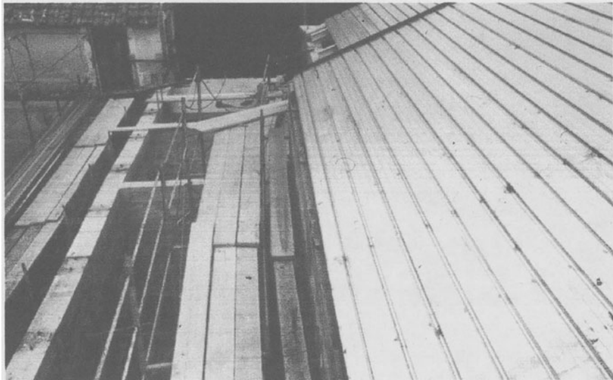
Figure 59. Corrugated sheeting for a new steel roof
