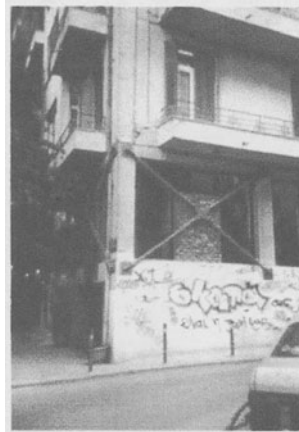
Figure 73. Steel cross braces in a building of Tessaloniki (Greece)
