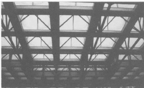
Figure 94. Support structure of the dome skylights
