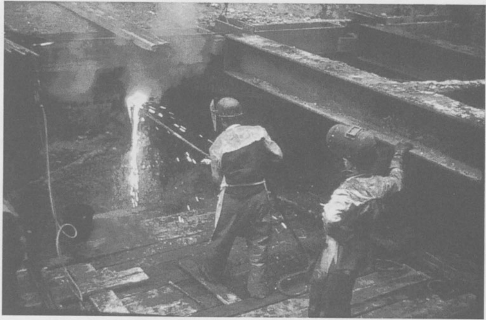
Photo 9. Thermic lance cutting (Courtesy Zschokke)
