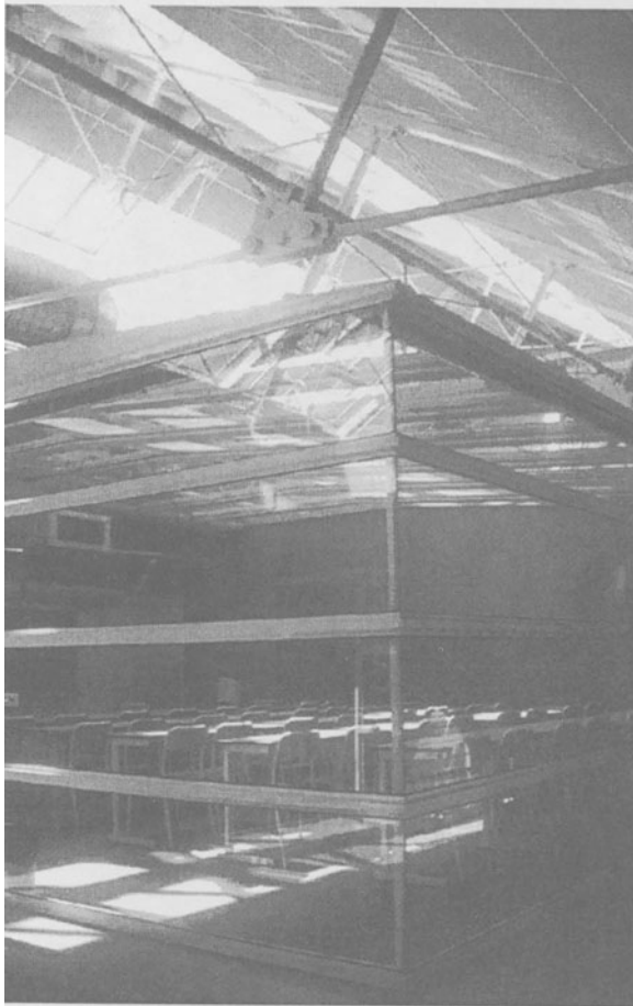
Photo 14. Internal view of the "Polonceau" trusses and upper teaching rooms.
