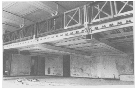
Figure 44. Insertion of mezzanine in the Ducal Palace of Genoa (Italy)
