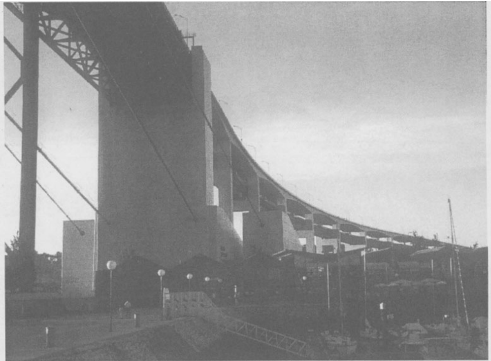
Photo 26. North bank anchorage blocks
