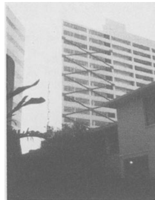
Figure 72. Steel cross braces in a building of St. Monica, Los Angeles (California USA)
