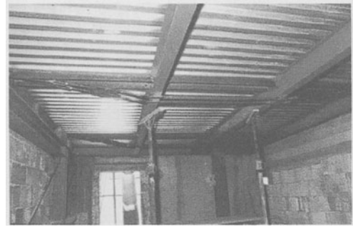
Figure 78. The new floor structure of the Capodimonte district (Ancona, Italy)
