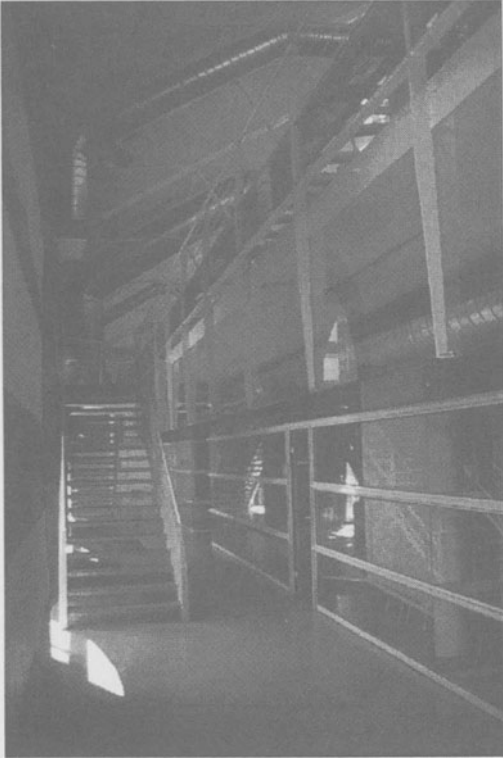
Photo 15. Stairs and lower level.
