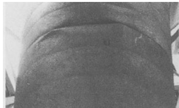
Figure 20. External view of the deformed hopper.
