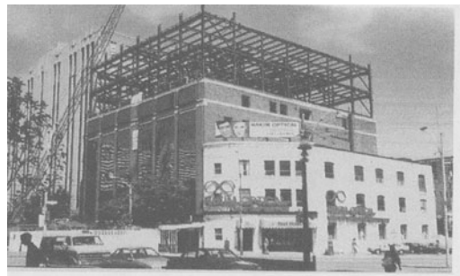
Figure 119. The additional floors under construction
