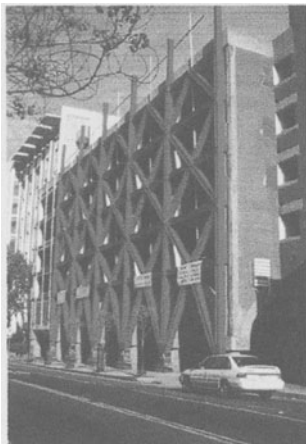
Figure 71. A parking building in Berkeley (California, USA)
