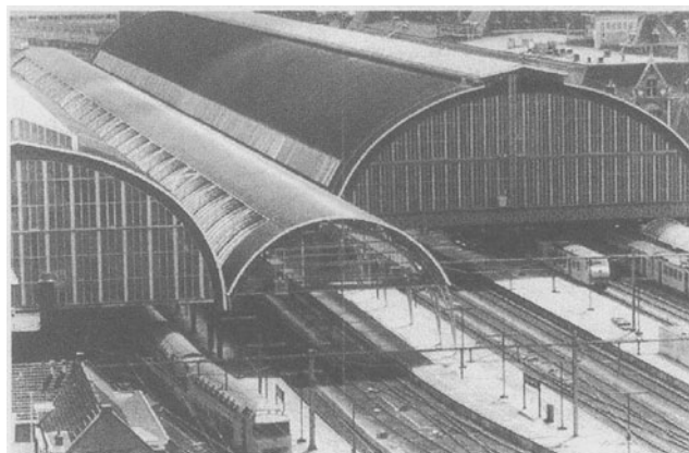
Figure 12. Intermediate Roof between North and South Roofs.
