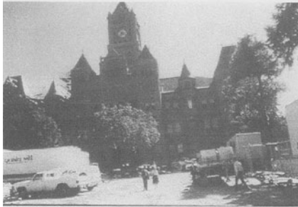
Figure 80. The first application of “base isolation” in a historical building: The City and Country Hall of Salt Lake City (USA)
