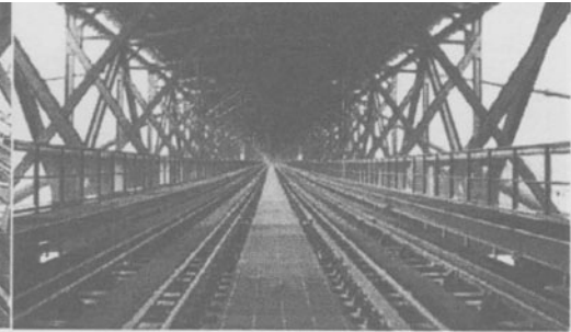
Photo 34. Railway tracks after completion
