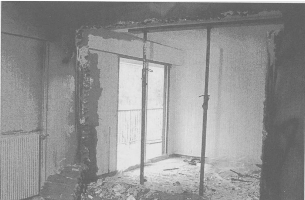
Photo 10. Result of an opening cut with a thermic lance (Courtesy Zschokke)
