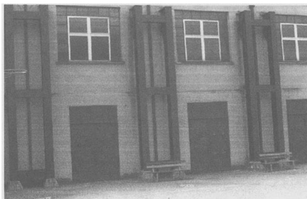
Figure 112. The new facade of the transformed building in Como (Italy)
