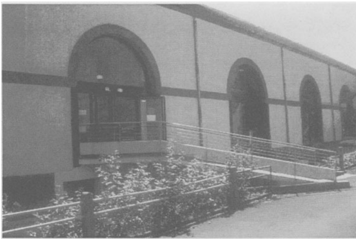
Photo 11. External view of the "Manège"
