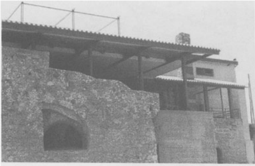
Figure 55. Vertical addition in a restored building in Briatico (Calabria, Italy)
