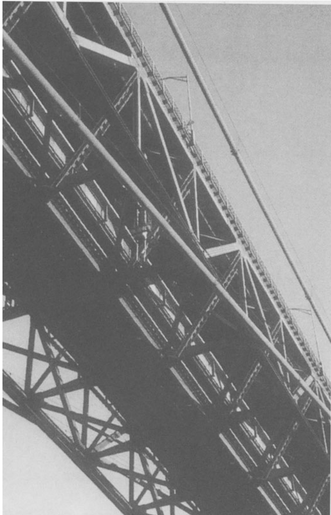
Photo 36. Downside view of the truss girder after completion of the improvement
