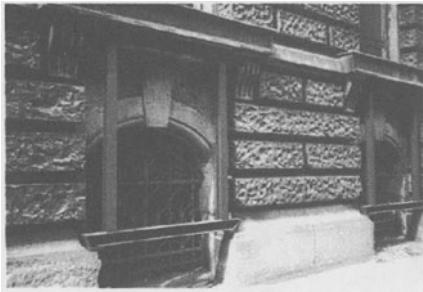
Figure 4. Provisional reinforcement by means of steelworks (Berlin)
