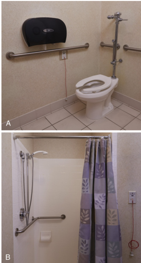
FIGURE 25.10 Grab bars provide a measure of safety for the patient using the toilet (A) and shower (B).
