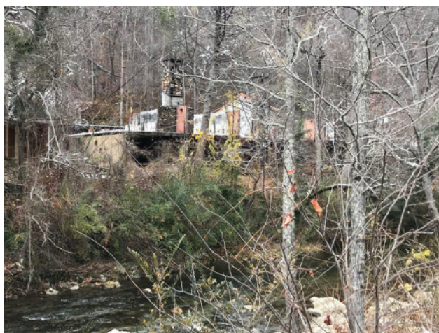
Figure 22-4 Remains of burnt riverside chalets from 2016 wildfire impacting Gatlinburg, TN. (Photo credit: Gordon Gillespie.)
