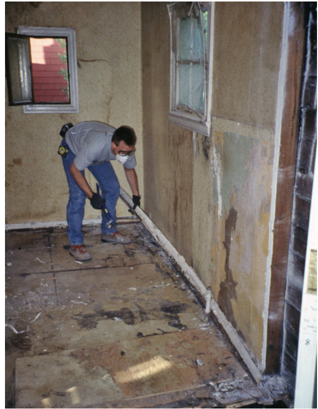
Figure 6-4 Removal of baseboards with lead paint. (From CDC/Aaron L. Sussell, 1993.)
