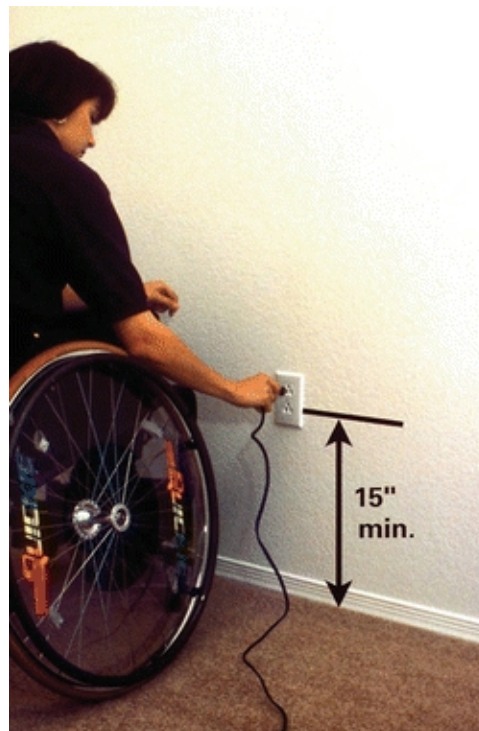
FIGURE 24-6 Recommended height of electrical outlet for ease of access for wheelchair-seated person. (From CDC Image Library. Retrieved from http://phil.cdc.gov/Phil/quicksearch.asp .)
