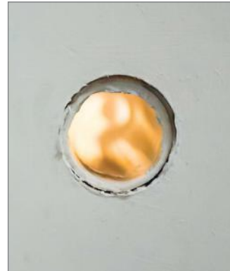
Fig. 11.3.4: A wave guide is simply a brass conduit through the scan room wall.
