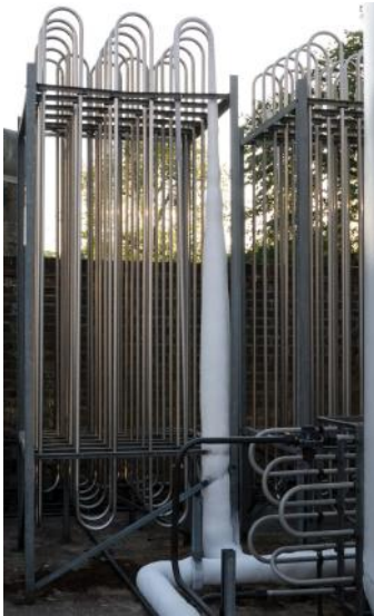
Fig. 1.1.3: Superheater coils. The pipes leading from the VIE are covered in frost because of the extreme cold.
