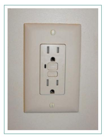
Figure 10.23 A GFCI With Three-Pronged Receptacle
