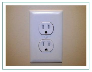
Figure 10.21 A Polarized Receptacle
