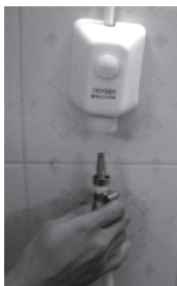
Fig. 1.2: Flexible colour coded Schrader probe
