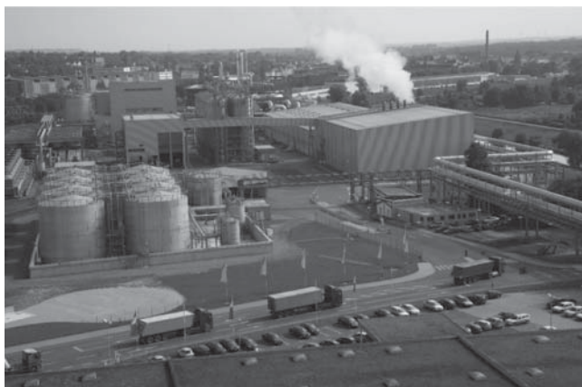
Figure 4.2 Ethanol fermentation plant of CropEnergies AG in Zeitz. Source: Courtesy of CropEnergies AG, Mannheim; © Martin Jehnichen.
