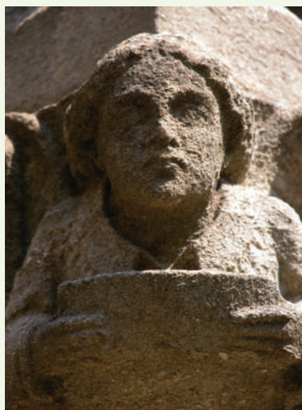
▲ This limestone statue adorning the Rheims Cathedral in France has been severely eroded by acid rain.
