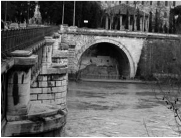
Figure 4 Outfall of Cloaca Maxima as it appears today. Source: Wikipedia.
