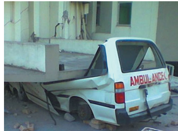
Figure 30.1 Damage to emergency medical services.
