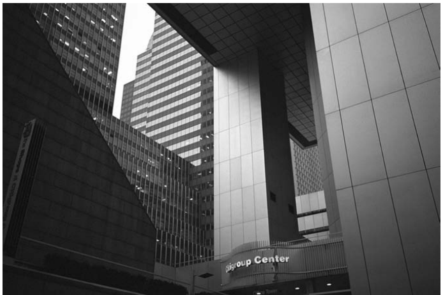
Figure 10-1. St. Peter's Church under the Citicorp Tower. Courtesy Bob Pitt, University of Alabama.
