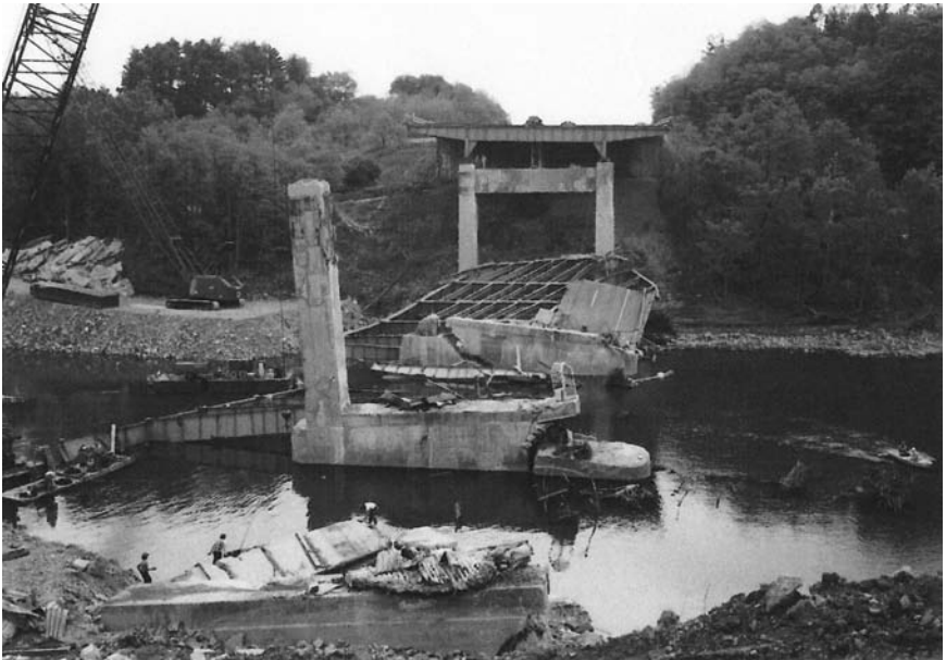
Figure 8-9. Schoharie Creek Bridge collapsed spans. Courtesy Howard F. Greenspan.
