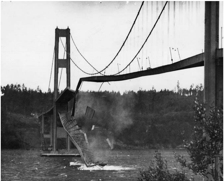
Figure 2-11. Tacoma Narrows Bridge collapse. Courtesy University of Washington Special Collections, photo UW21422.
