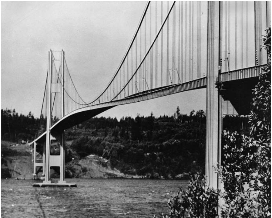
Figure 2-10. Tacoma Narrows Bridge torsional motion. Courtesy University of Washington Special Collections, photo UW21413.
