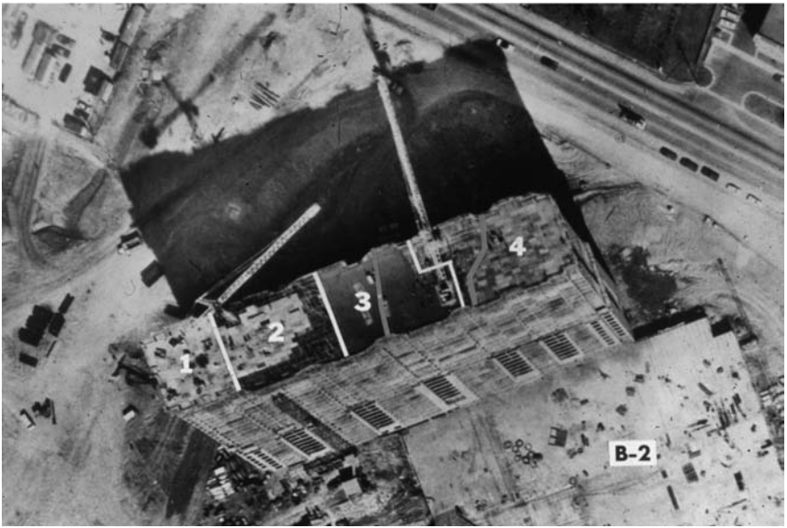
Figure 5-5. Skyline Plaza before the collapse.
