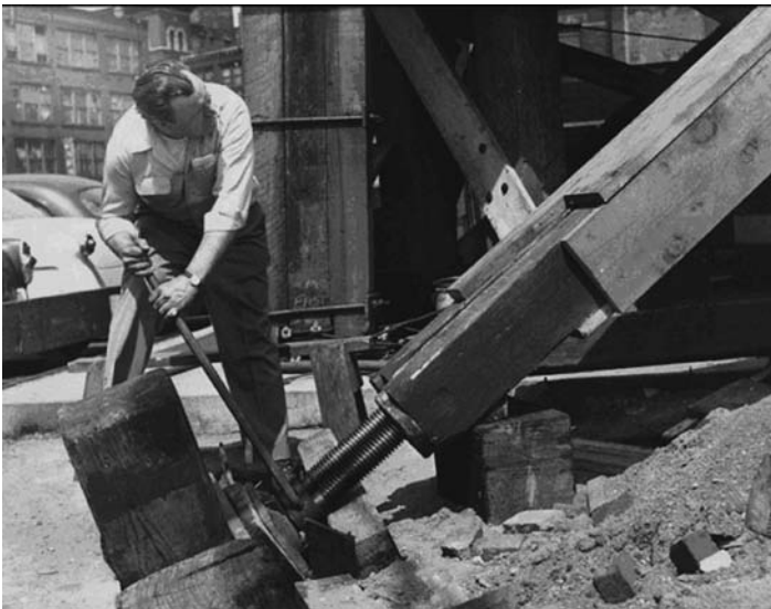
Figure 4-18. Restoring the Cleveland parking garage to plumb. Courtesy Cleveland Press Collection, Cleveland State University Library.
