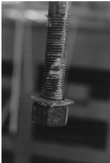
Figure 2-6. Hanger rod. Courtesy Lee Lowery, Texas A&M University.
