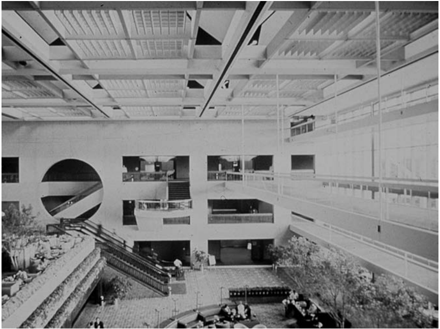
Figure 2-2. The Kansas City Hyatt Regency atrium walkways.
