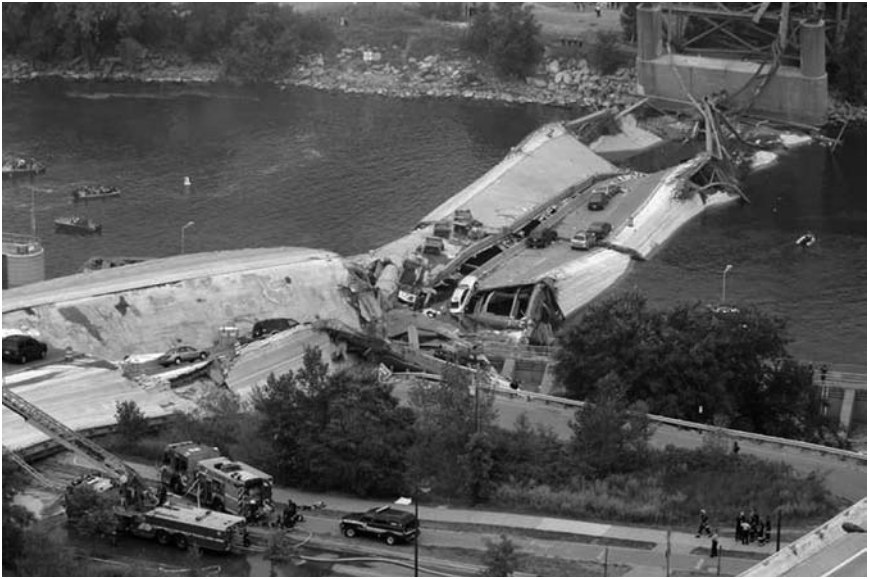
Figure 6-12. Wreckage of the collapsed Minneapolis I-35W Bridge.
