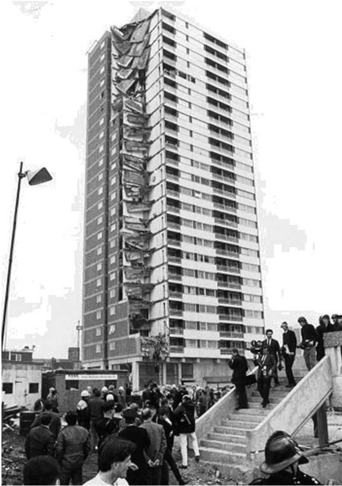
Figure 4-5. Ronan Point after collapse. Source: Pearson and Delatte (2005).
