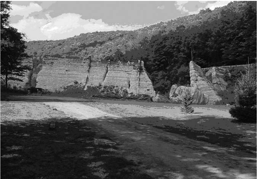
Figure 9-2. The failed Austin Dam.
