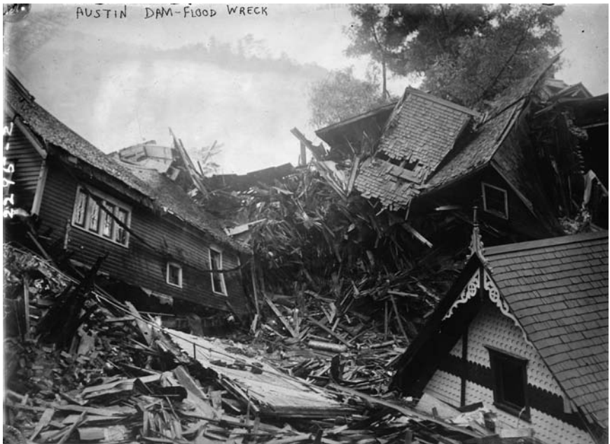
Figure 9-3. Damage from the Austin Dam failure. Courtesy Library of Congress.
