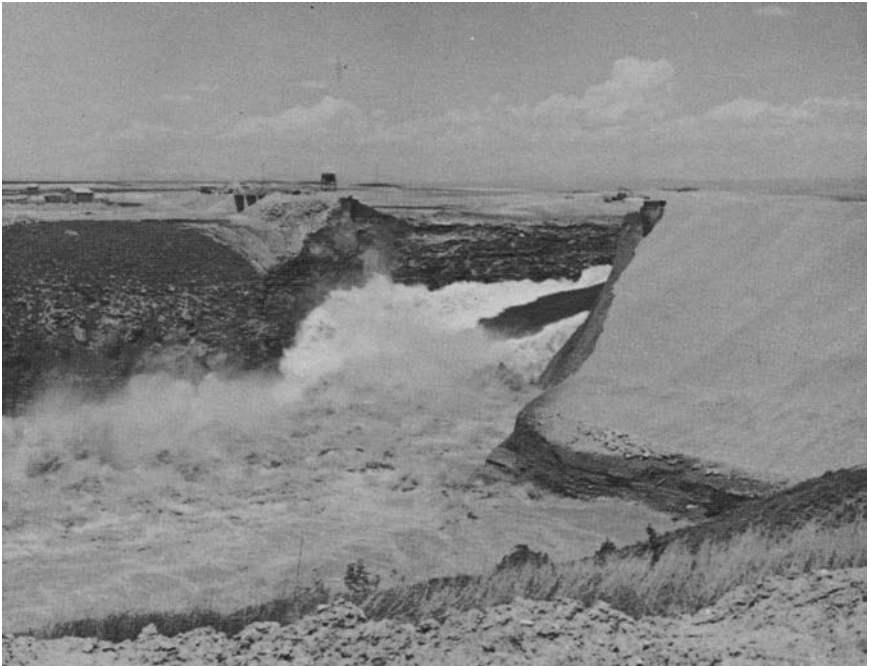
Figure 7-3d. Failure sequence, failure of dam. Source: Independent Panel (1976).
