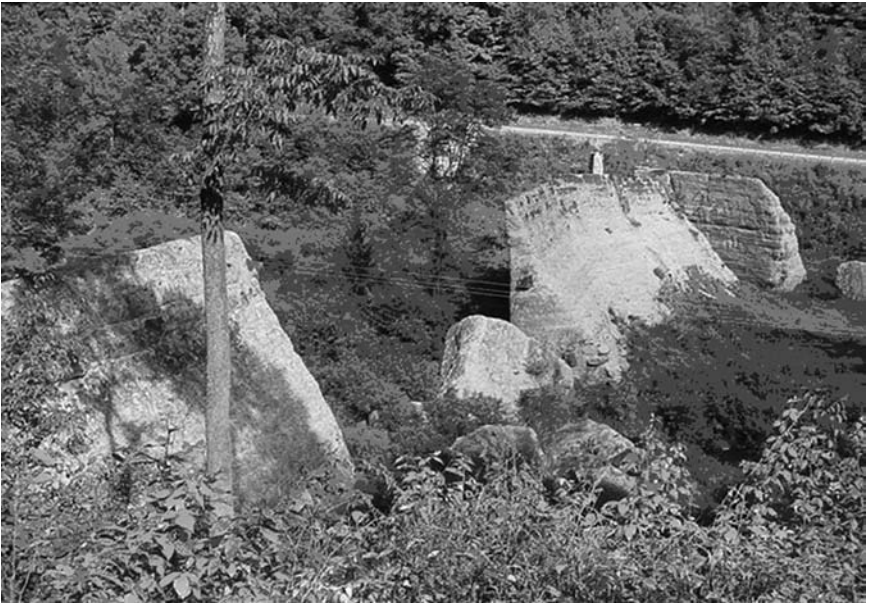
Figure 9-1. The failed Austin Dam.
