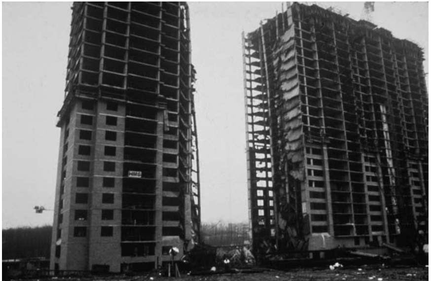
Figure 5-6a, b. Collapse of Skyline Plaza, Bailey's Crossroads. Courtesy National Bureau of Standards/National Institute of Standards and Technology.
