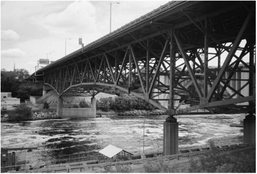
A view of the west side of the deck truss portion of the bridge, looking northeast.
