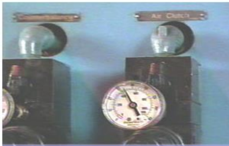
Figure 2. Be sure that the clutch or brake psi settings are correct.
