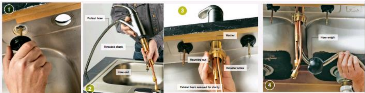
Figure 3.81 Steps of Installation of sink
