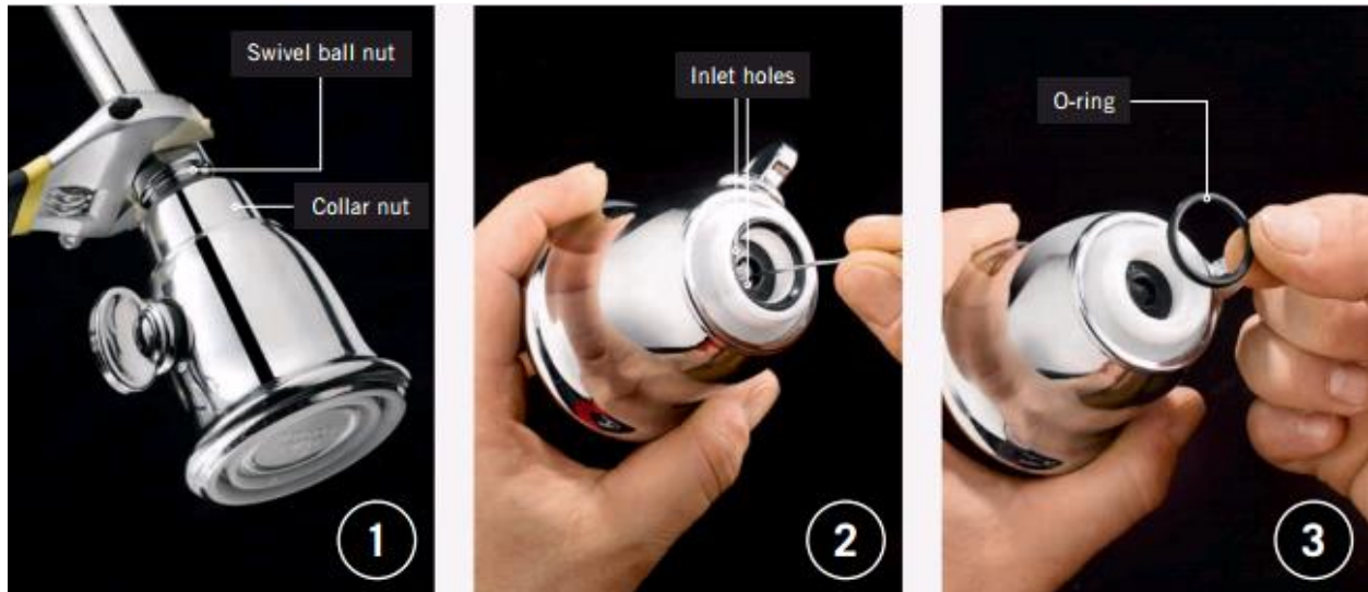
Figure 3.69 Repairing of shower head
