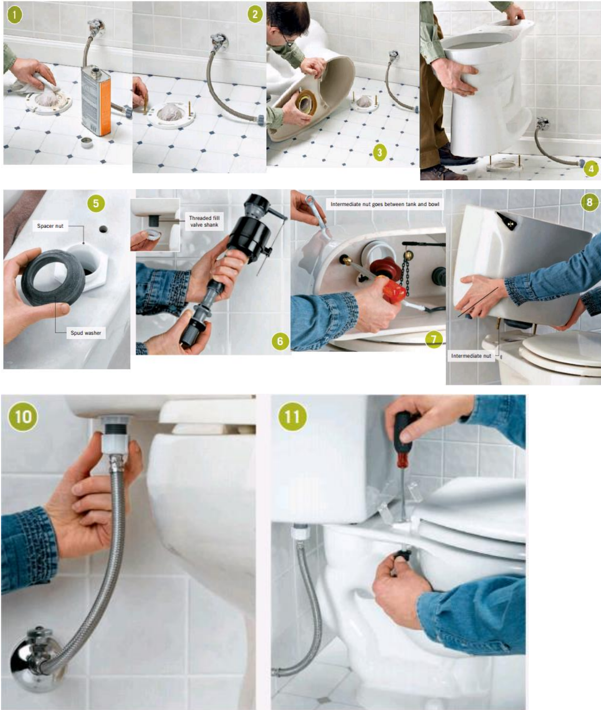
Figure 3.51 Steps installation of floor-mounted water closet bowl
