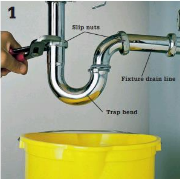
Figure 3.93 Remove and Clean Sink Drain Trap
