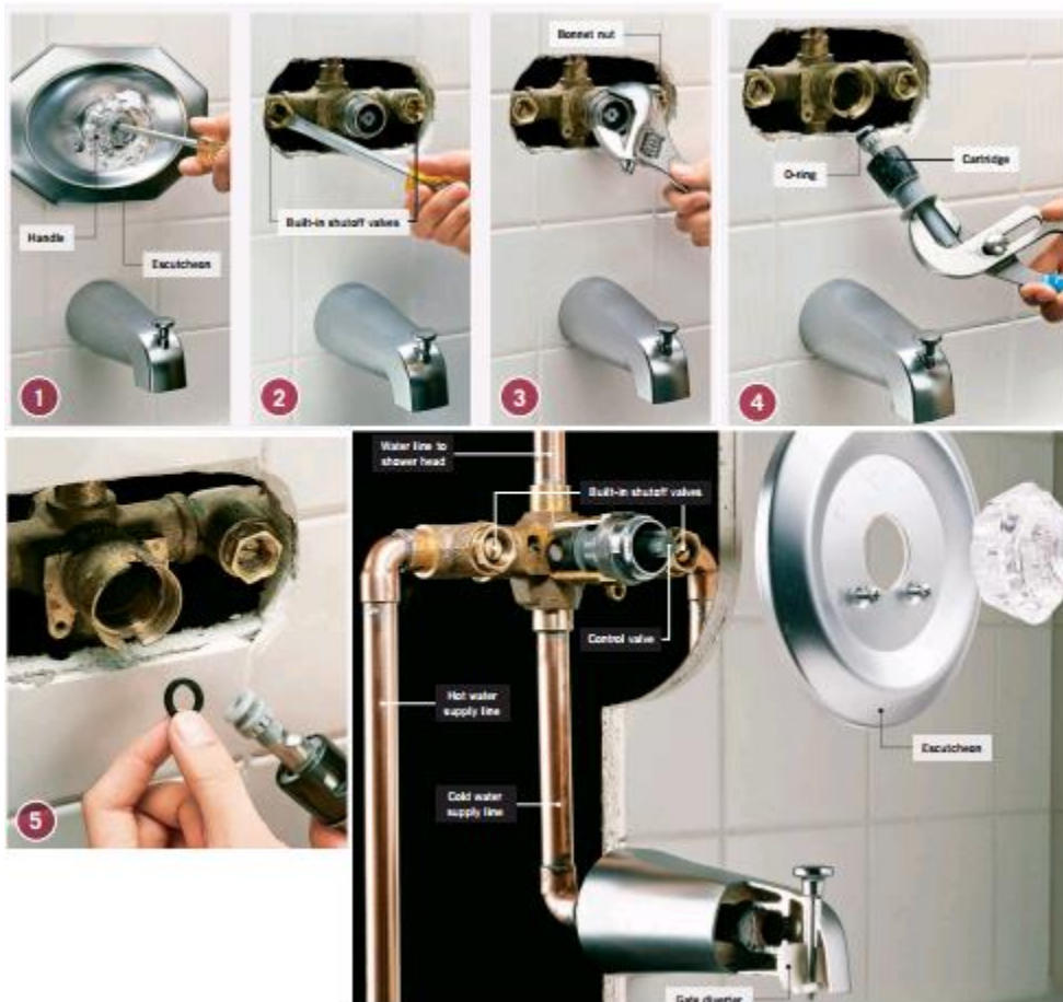
Figure 3.72 Fixing Single-Handle Tub & Shower Faucets
