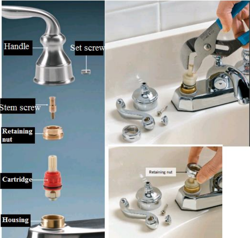
Figure 3.88 Washerless Two-Handle Faucet
