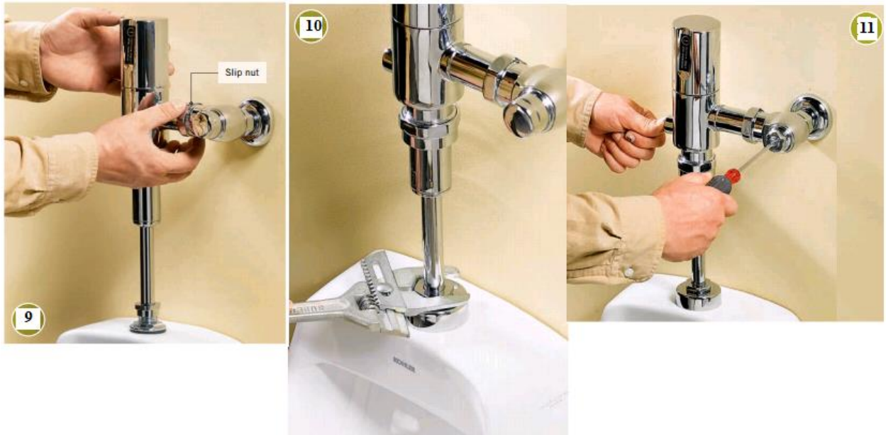
Figure 3.61 Steps to Install Wall-hung Urinal
