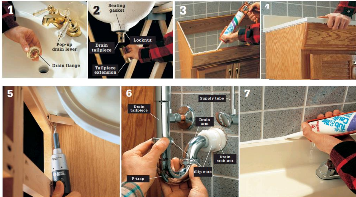
Figure 3.85 Installing an Integral Vanity Top
