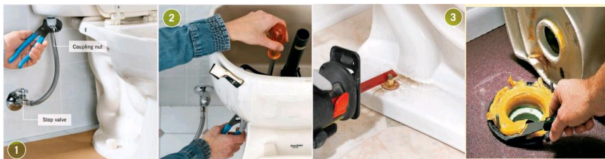
Figure 3.55 Steps to Repair water closet
