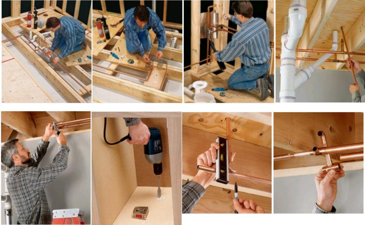
Figure 2.40 Copper pipe system installations
