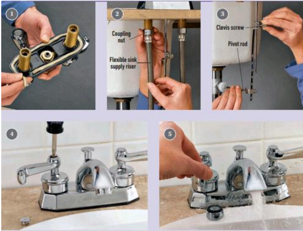
Figure 3.32 Installing a single-body faucet
