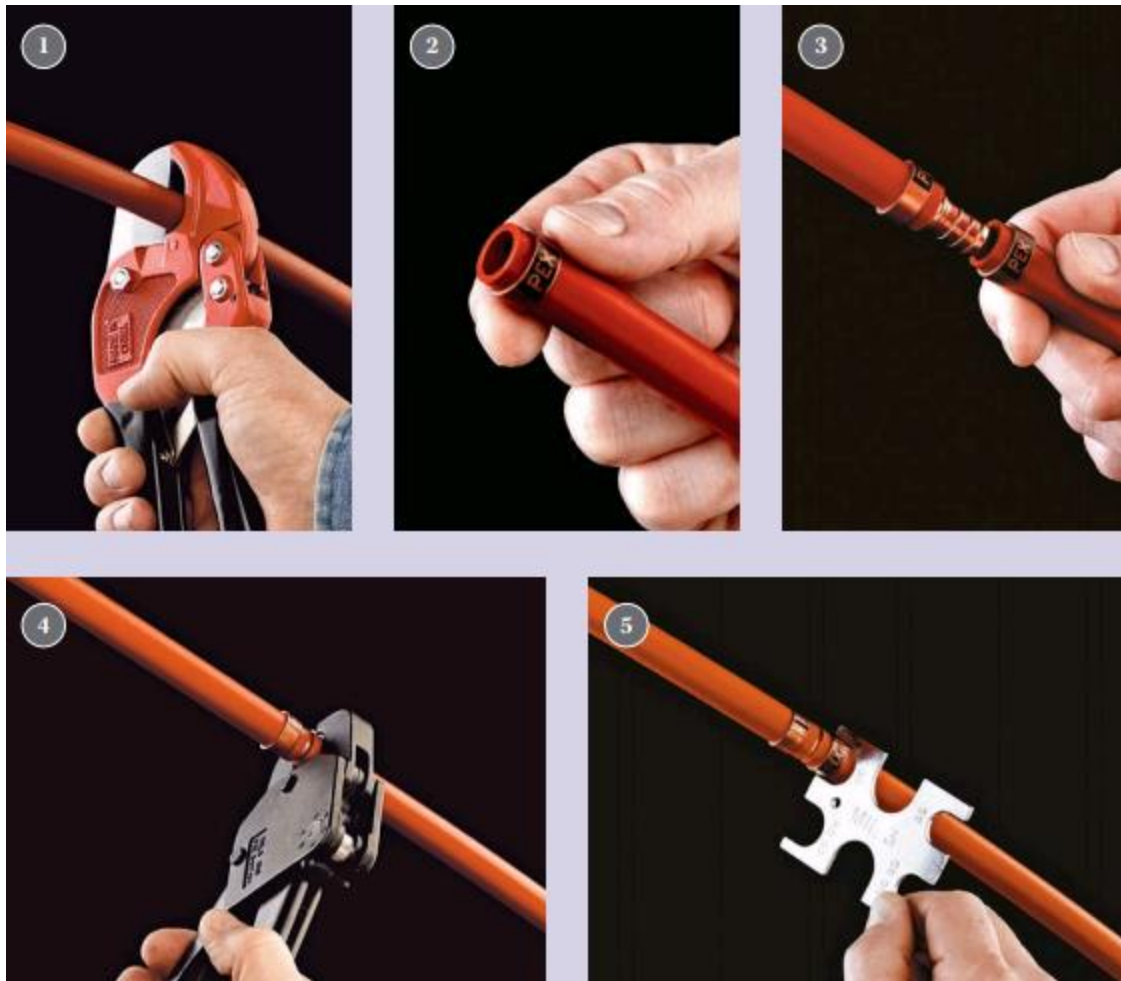
Figure 2.42 Steps of installing PEX
