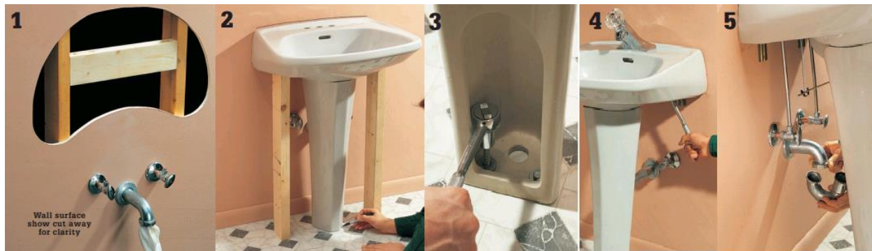
Figure 3.27 Install a Pedestal Sink
