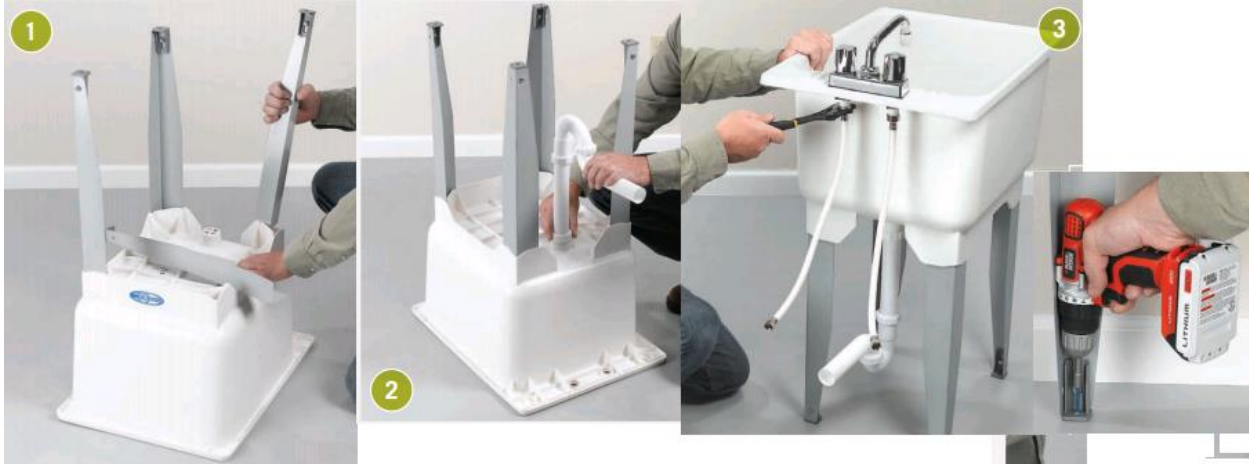
Figure 3.86 Detailed steps to install slop sink
