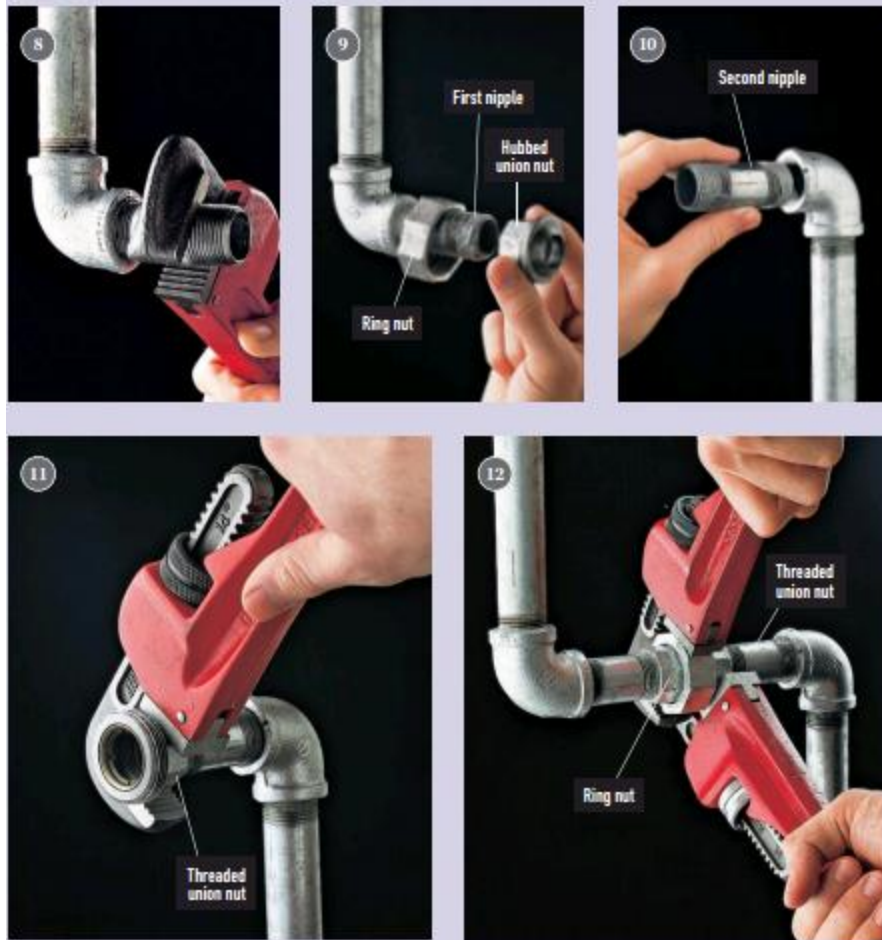
Figure 2.24 Replacing, maintaining, and joining old pipe
