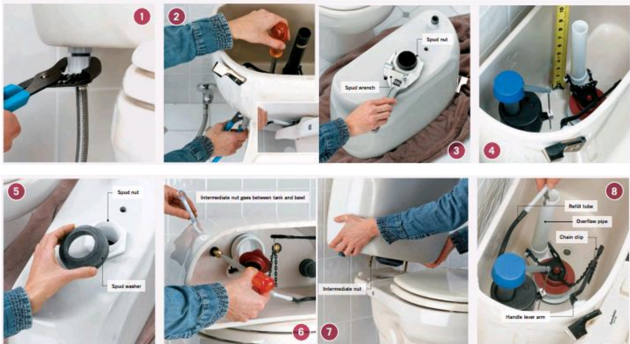
Figure 3.44 Installation of Flush Valve
