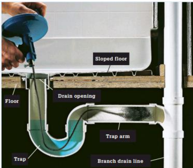
Figure 3.66 Clearing of Shower pan installation
