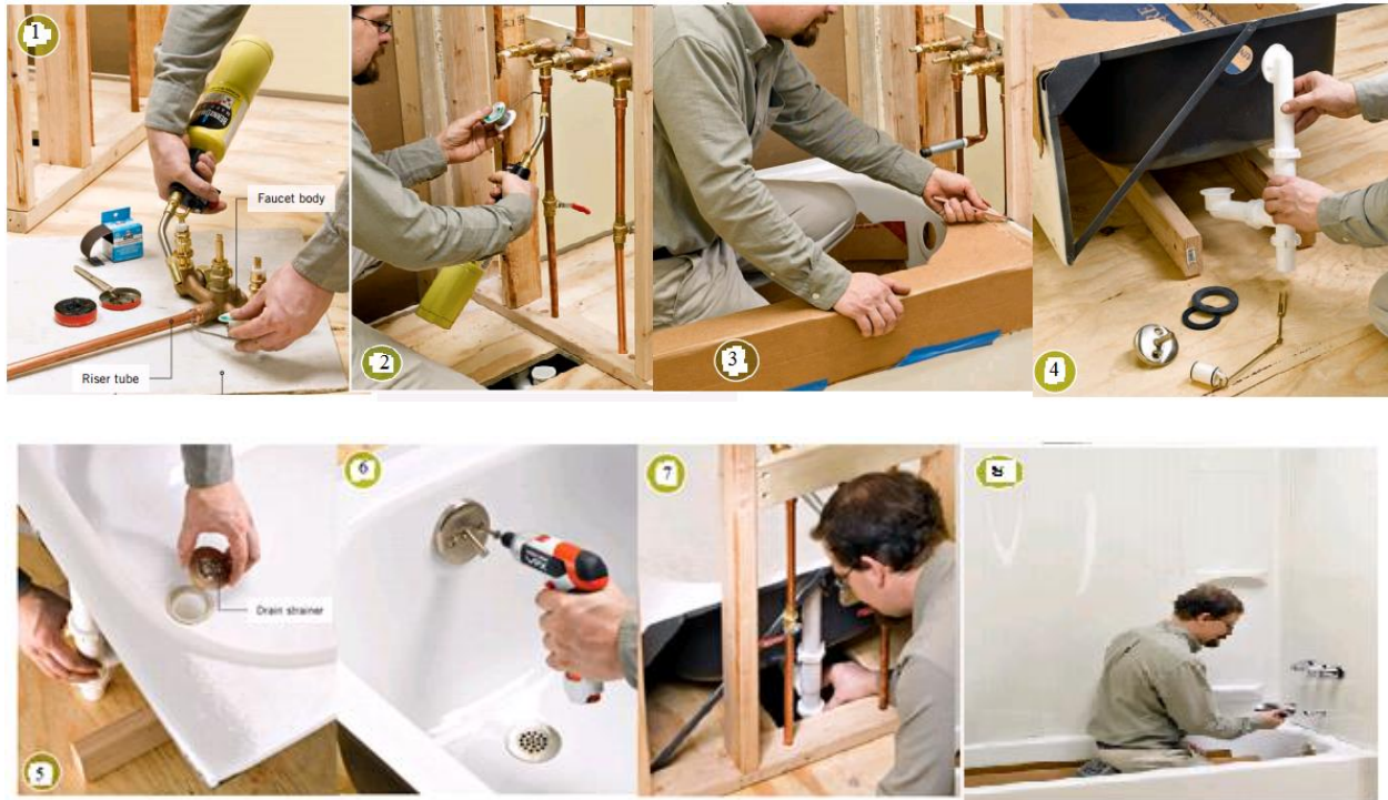
Figure 3.7 Steps of Installation of Bathtub
