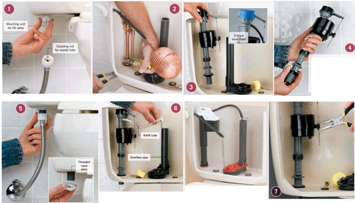
Figure 3.45 Installation of Fill Valve
