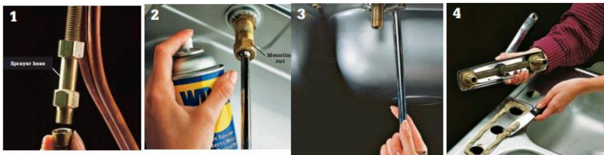
Figure 3.98 Maintaining and Repairing of Sink faucet
