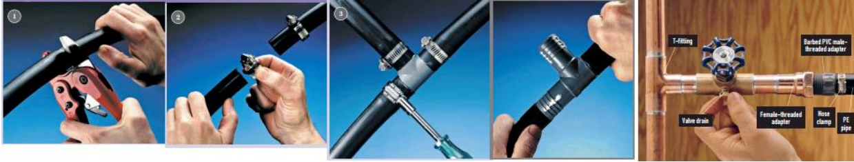
Figure 2.49 Steps to join flexible plastic pipe
