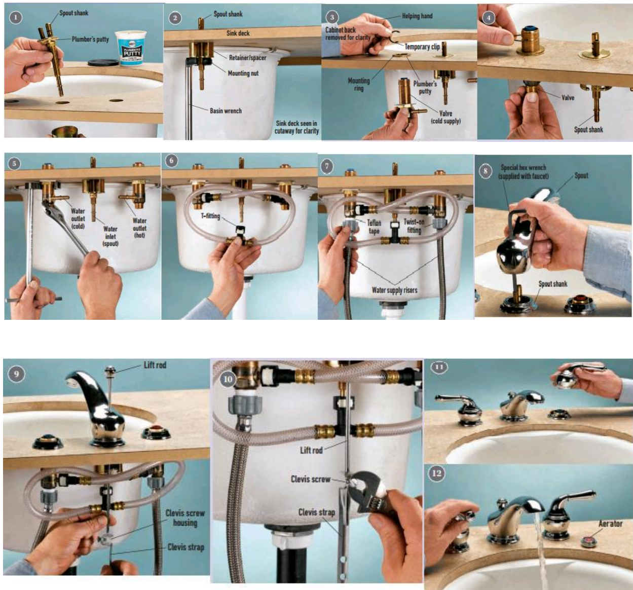
Figure 3.31 Installing a widespread faucet
