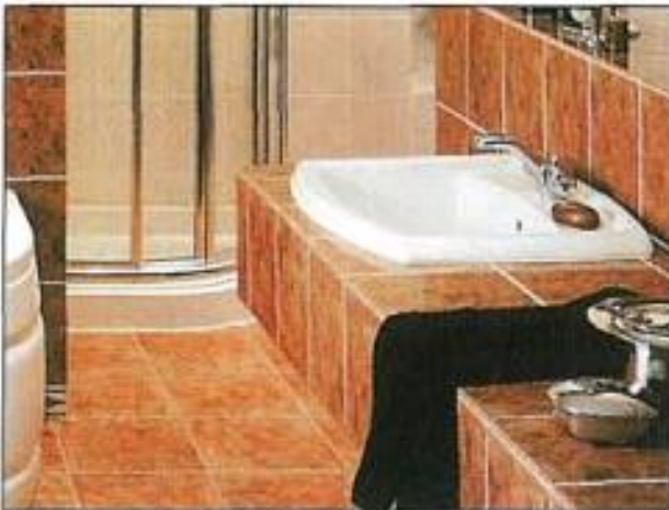
Figure 3.25 Counter-top basins
