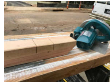
Fig 107 Cut the cross lap perimeters
