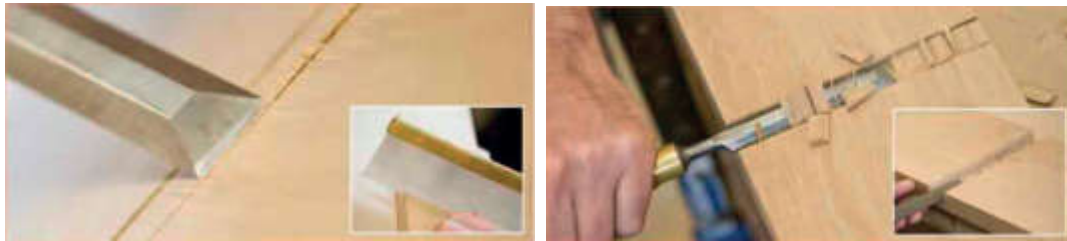
Fig 133 Cut the dado with a chisel
