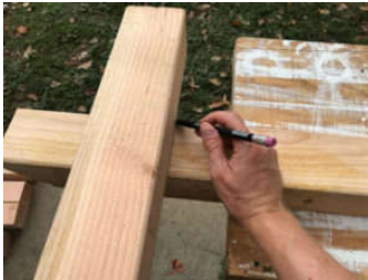
Fig 106 Mark the cross lap position
