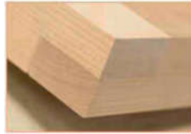
Fig 105 The finished joint
