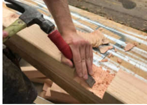
Fig 110 Clean the groove with a chisel
