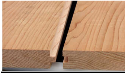
Fig 117 The tang and the groove
