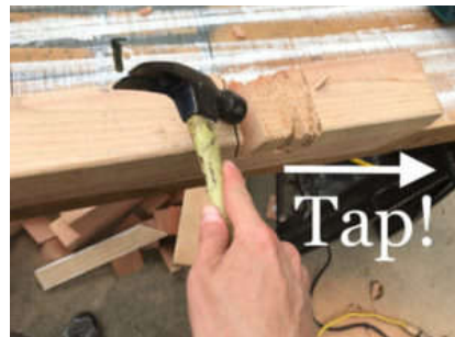
Fig 109 Remove the cut scraps
