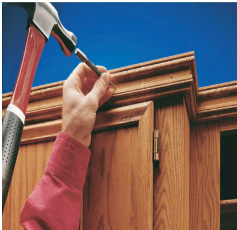
Fig. 153 Decorative moldings give a finished appearance walls, doors, windows, and cabinets.
