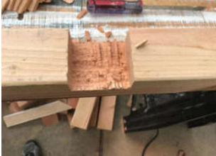
Fig 110 Clean the groove with a chisel
