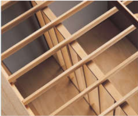
Fig 149 A new wall is perpendicular to the ceiling
