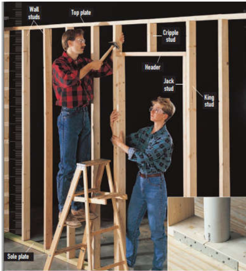
Fig 148 A typical partition wall
