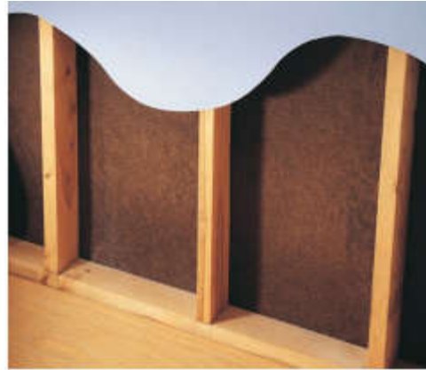
Fig 139 Platform framing
