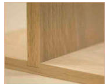
Fig 136 The final joint
