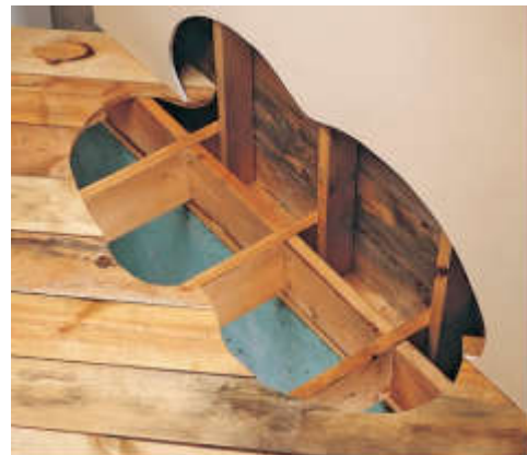
Fig 141 Balloon framing
