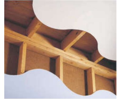
Fig 143 Load bearing wall
