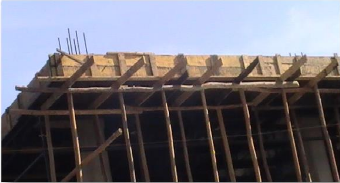
Beam and slab formwork
