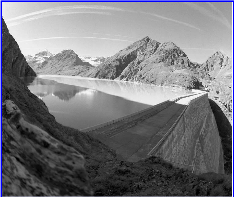
Grande Dixence Dam, Switzerland (285 m, 1961).
