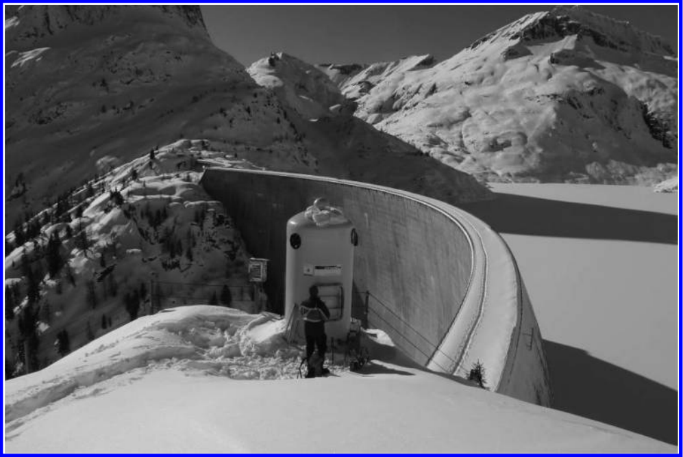
Figure 4. Protective cabin for the permanently installed total station T1 on the left bank (photo: Straub AG).
