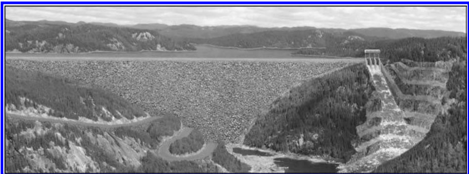
Figure 4. Romaine 2 Main dam and spillway (CATIA simulation).
