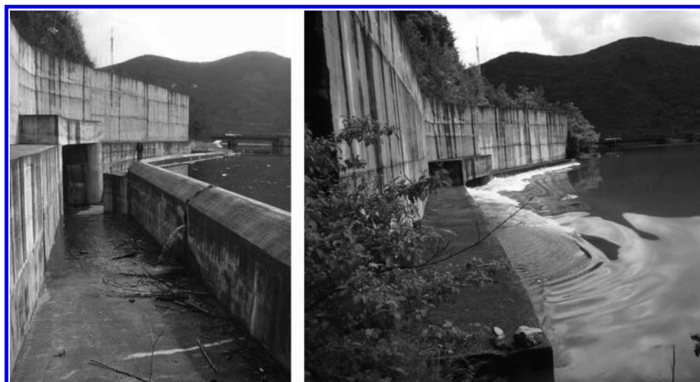
Figure 5. Additional uncontrolled side spillway and its use during floods in 2010.
