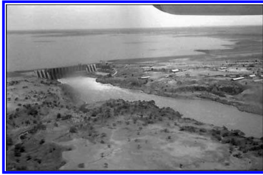
Figure 5. General view dam and reservoir.
