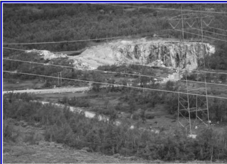
Figure 3. The quarry during construction periode (Photo: Skrindo).
