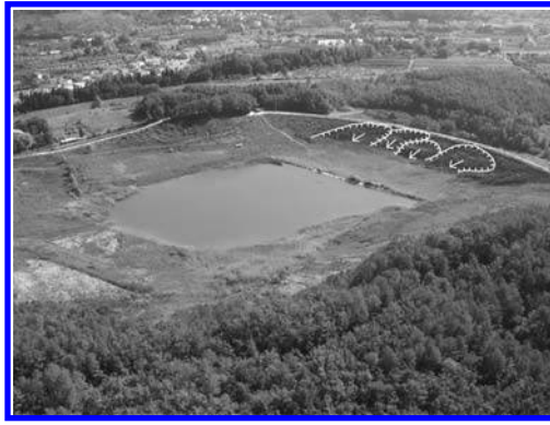
Figure 1. Giudea impound—evidence upstream shell slides (2007).
