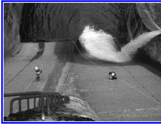
Figure 1. Dam surface inspection by rope access.
