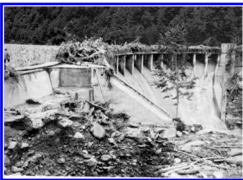
Figure 4. Palagnedra Dam. Spillway clogged with debris during 1978 flood.
