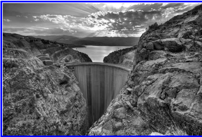
Figure 2. Picture of the dam from downstream taken in October 2010.
