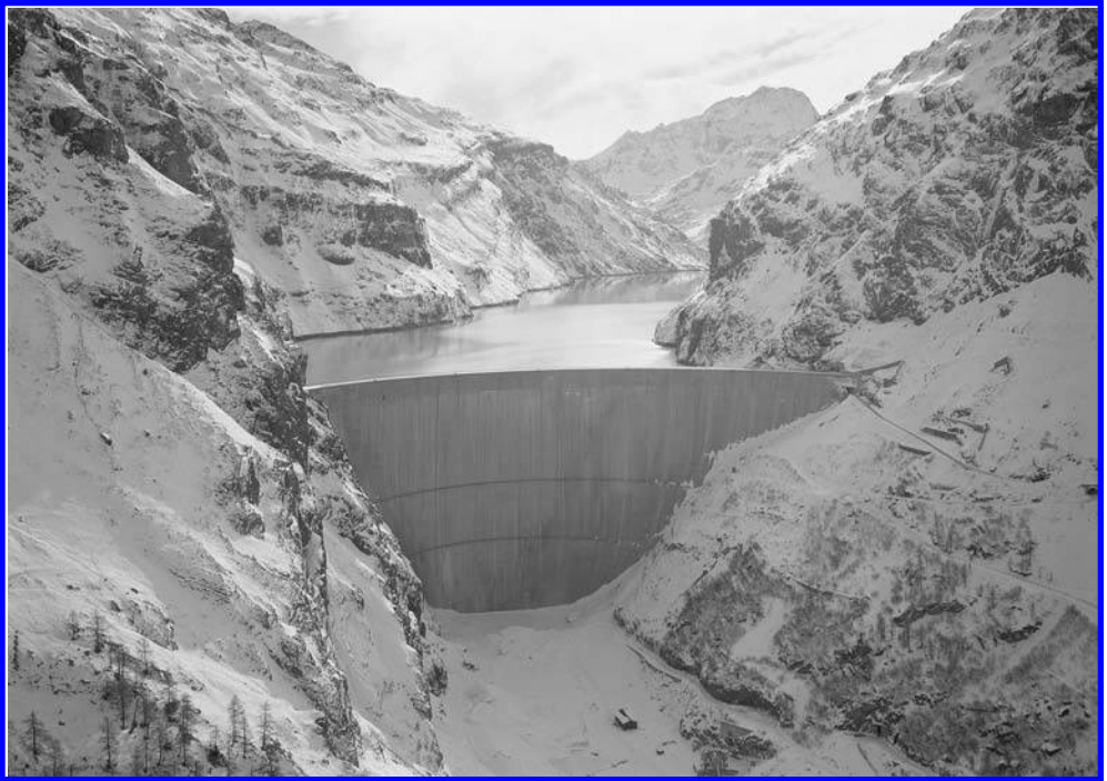
Mauvoisin Dam, Switzerland (250 m, 1957/1991).
