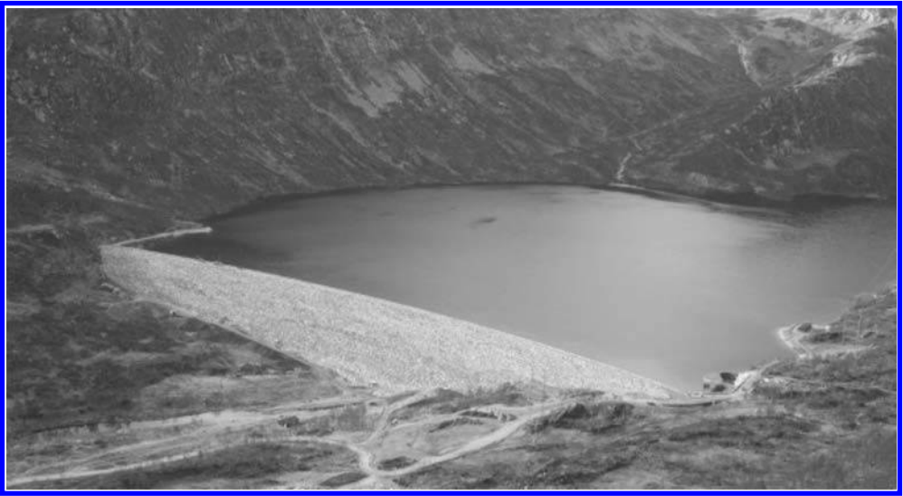
Figure 7. Bitdalen dam after rehabilitation (Photo: Søreide).
