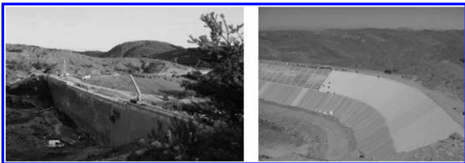
Figures 12 and 13. At left Riou RCC dam, new construction, exposed geomembrane. At right Sar Cheshmeh tailings dam in Iran, upstream exposed PVC geomembrane anchored with PVC wings.
