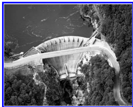
Figure 5. Bridge and piers were removed from spillway. New bridge constructed downstream.
