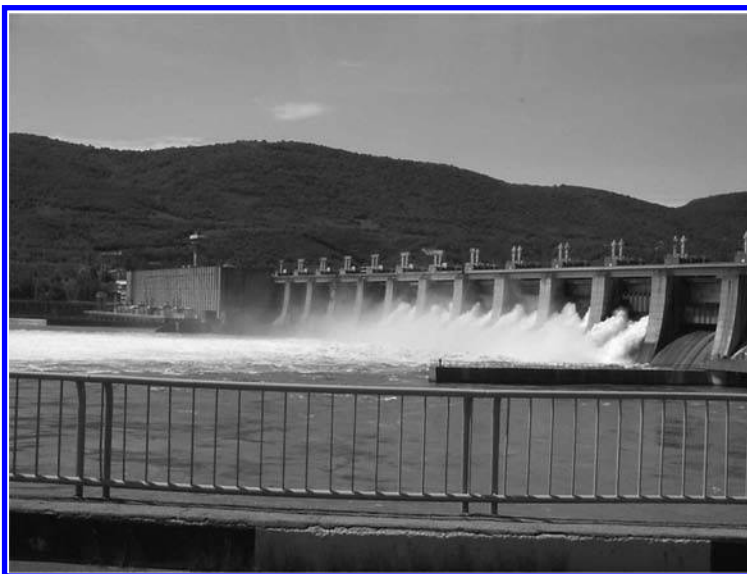
Figure 2. Hydropower plant, control center.
