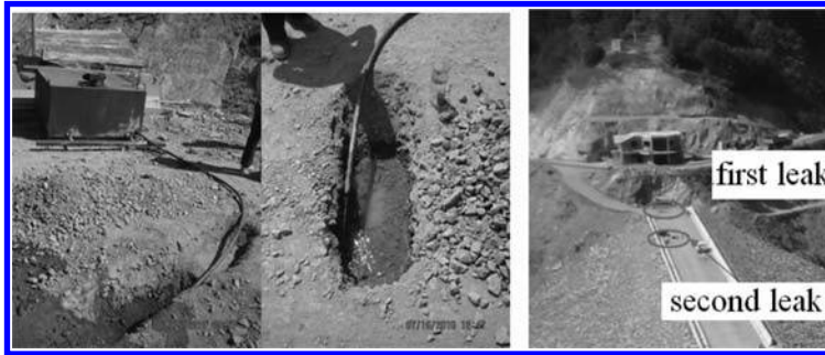
Figure 10. Leakage simulation test with 0.15 l/s.
