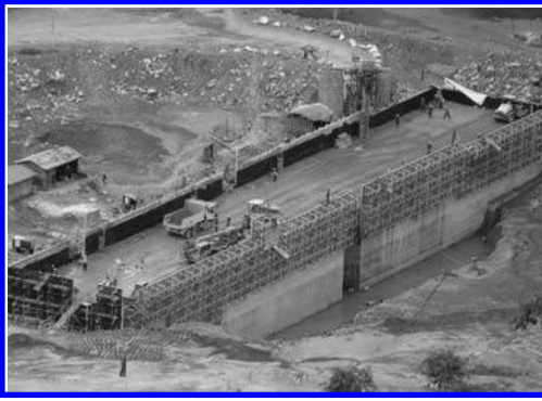
Figure 14. Separation wall under construction.
