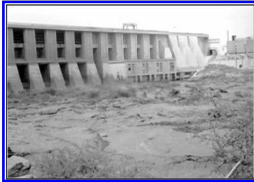
Figure 7. Downstream dam flushing.
