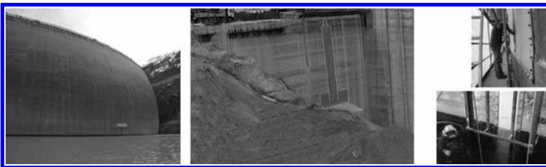
Figures 4, 5, 6 and 7. Scheme of the areas waterproofed at Toules dam (left) and Platanovyssi dam (middle, artist's impression from the upstream side). At right, the waterproofing system installed from fixed sheltered scaffolding at Toules (top) and underwater at Platanovyssi (bottom).
