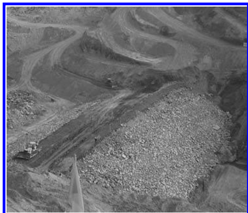
Figure 4. U/s cofferdam with clay core.
