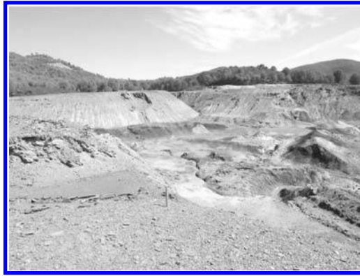
Figure 1. Las Viñas abandoned mine (13 September 2010). 400,000 m 3 of waste embankments have been thrown into Almagrera reservoir.
