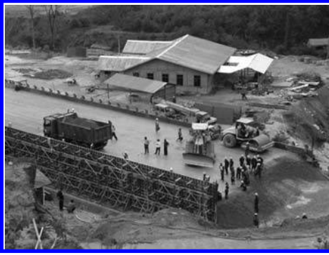
Figure 12. RCC FST embankment.
