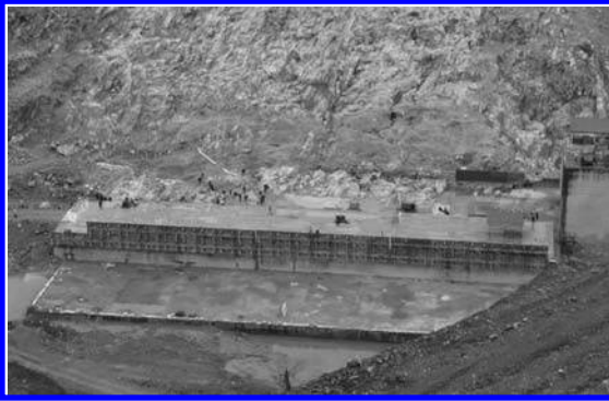
Figure 16. Leveling concrete and RCC.
