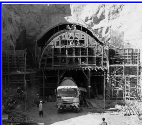
Figure 3. Diversion inlet under construction.
