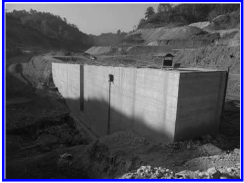
Figure 15. Separation wall completed.
