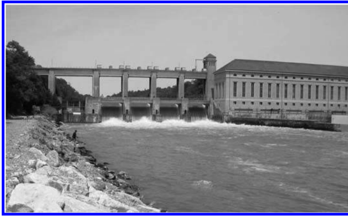
Figure 1. Chancy-Pougny hydroelectric development.
