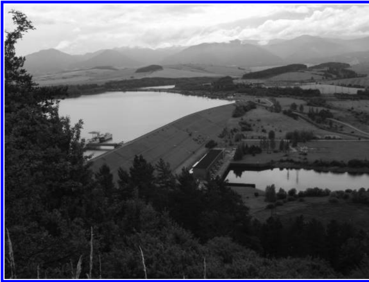
Figure 2. Liptovská Mara Dam—technical and safety supervision found a lack of efficacy of the injection sealing curtain, subsequently bedrock was sealed.
