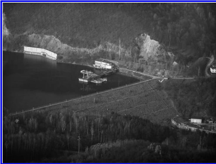
Figure 3. Rockfill Dam Ružín I, where was inadequate capacity of safety spillway found, subsequently side safety spillway with bypass tunnel was built.
