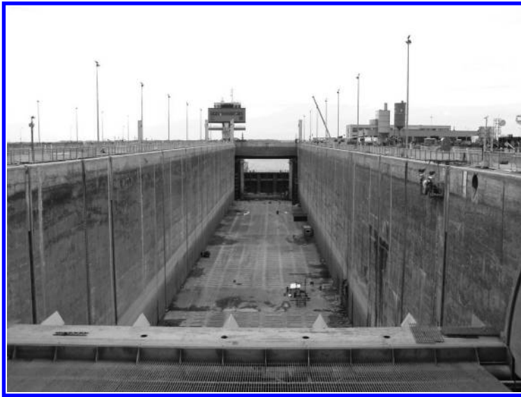
Figure 4. Lock chamber of Waterwork Gabčíkovo—inspection and repairing of dilatation.
