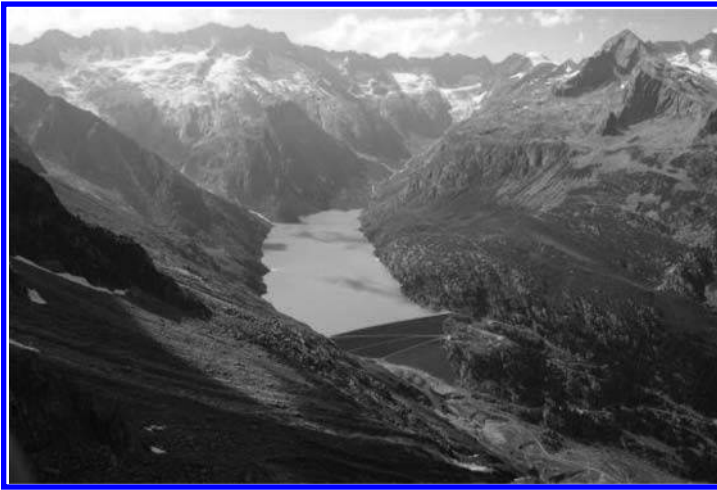
Figure 2. Goescheneralp dam and reservoir with Dammastock mountain in the background (view from East to West).
