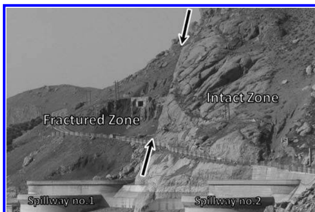
Figure 3. Fractured and intact zone and morning glory spillways.
