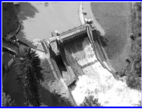
Figure 6. Wichelsee Weir with (1) bottom outlet, (2) lift gate and (3) adjacent embankment dam after passage of the flood of 2005.
