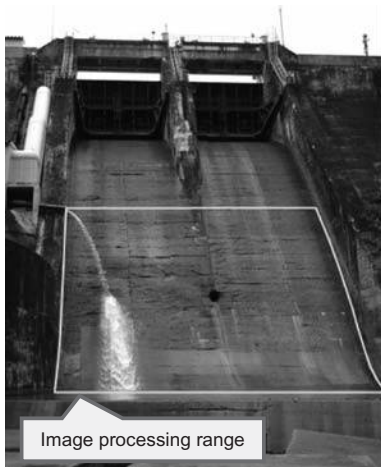
Figure 6. Distant view on the dam downstream side.
