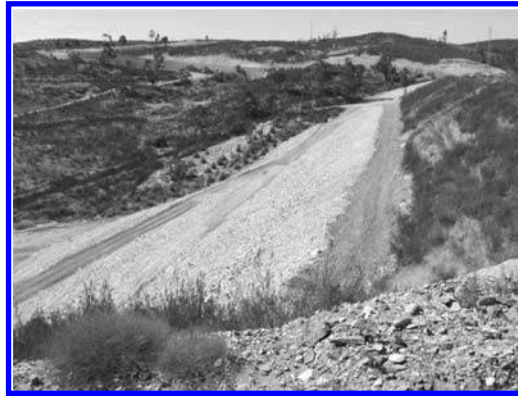
Figure 5. Almagrera closure reinforcement (13 September 2010).
