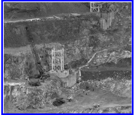
Figure 17. Conveyor belt foundation.
