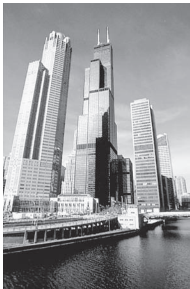
FIGURE 1.2 Willis Tower (formerly the Sears Tower). (© Bill Bachmann/Photo Researchers.)
