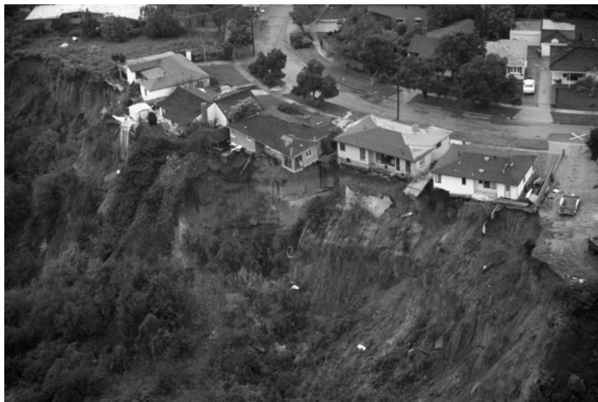
FIGURE 10.1 Shear failure of soil under several homes. (©Vince Streano/Corbis.)
