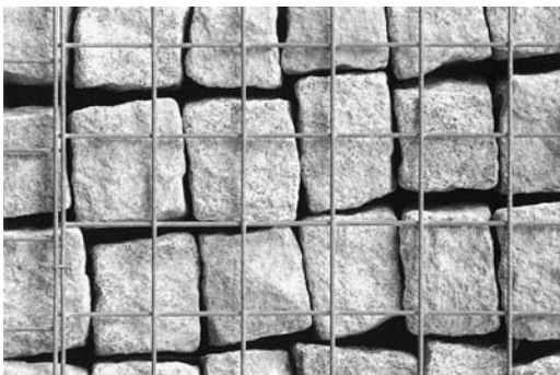
FIGURE 15.32 Gabion basket wall. (Alamy Images.)
