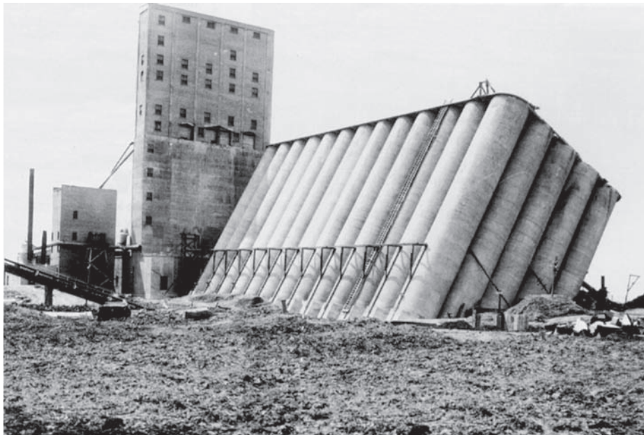
FIGURE 1.6 Failure of the Transcona Grain Elevator. (Photo courtesy of Parrish and Heimbecker Limited.)
