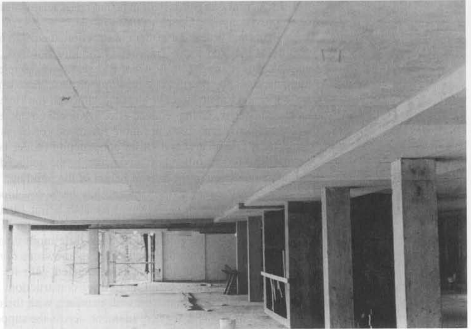
(a) Interior slab band
