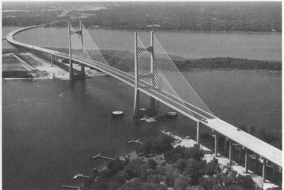
FIGURE 1.8 Napoleon Bonaparte Broward Bridge, with a 1300 ft center span at Dame Point, Jacksonville, Florida. (HNTB Corporation, Kansas City, Missouri.)
