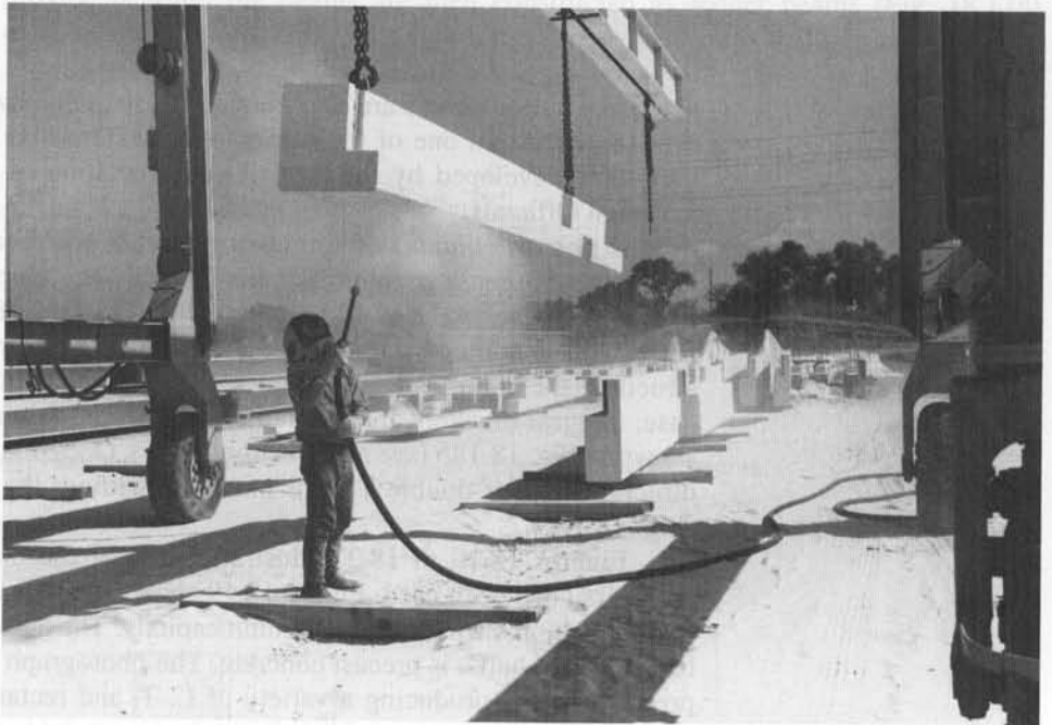
FIGURE 18.20 Sand-blasted architectural finish applied to a precast L beam.
