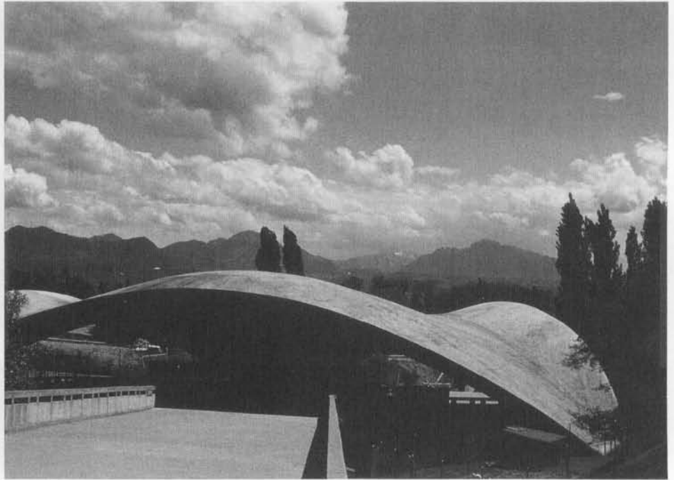
FIGURE 1.7 Spherical shell in Lausanne, Switzerland. Upwardly curved edges provide stiffening for the central dome.
