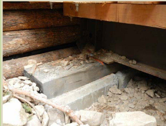
The steel superstructure is bolted to the timber cap and the deck panels are properly attached.
