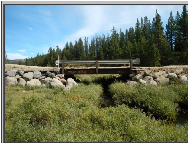
This bridge has adequate clearance for expected flows.
