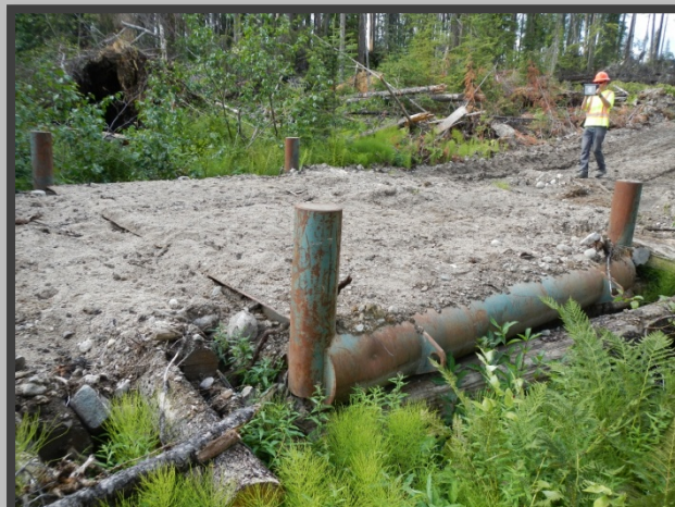
This bridge is resting on logs in the channel of a fish stream. It was supposed to be removed before spring but was in place in late July. It is blocking fish passage.
