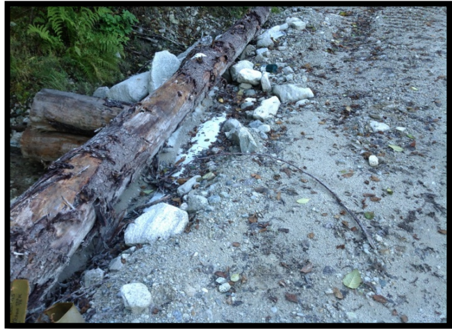
This curb log is undersized, unsecured and does not meet WorkSafe BC regulations.
