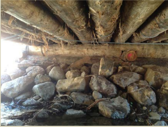
This log stringer bridge was lashed tightly with steel cable.
