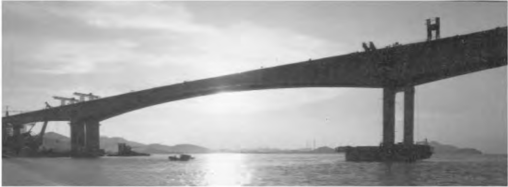
FIGURE 63.20 Humen Bridge (continuous rigid frame).
