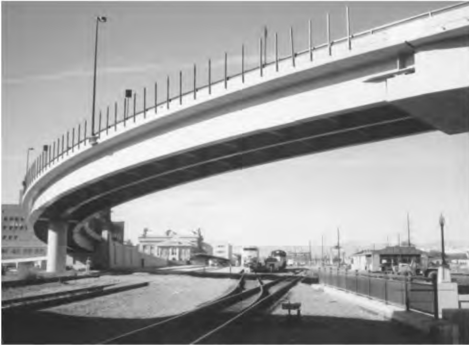
FIGURE 15.3 Curved I-girder bridge with integral bent cap.
