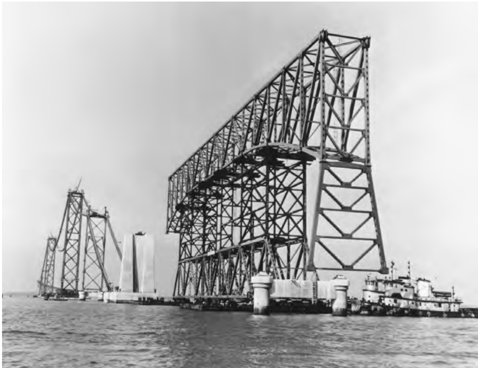
Figure 45.31 Floating-in erection of a truss span, first Chesapeake Bay Bridge, Maryland, 1952. A 480 ft (146 m) truss span, weighting 850 tons, supported on falsework consisting of a permanent deck-truss span along with temporary members, is being floated-in for landing onto its piers. Suspension bridge cables are under construction in background. (Courtesy of Bethlehem Steel Corporation.)
