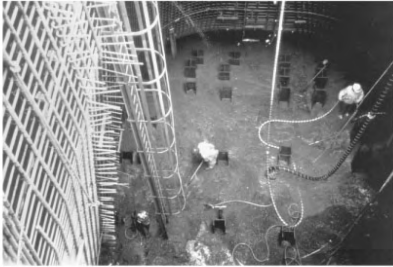
FIGURE 47.13 Pumped-out cofferdam showing tremie concrete seal and predriven steel H-piles.
