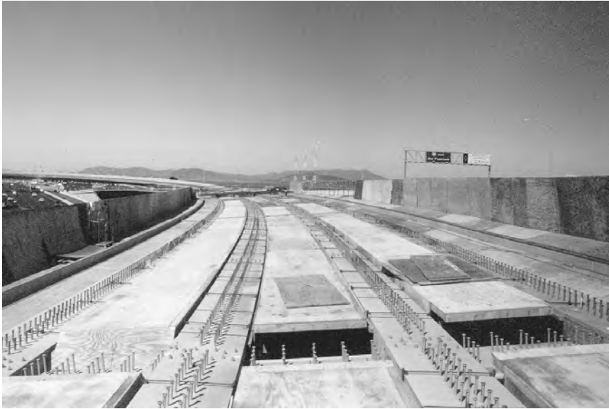
FIGURE 48.11 Temporary deck form for steel bridge.
