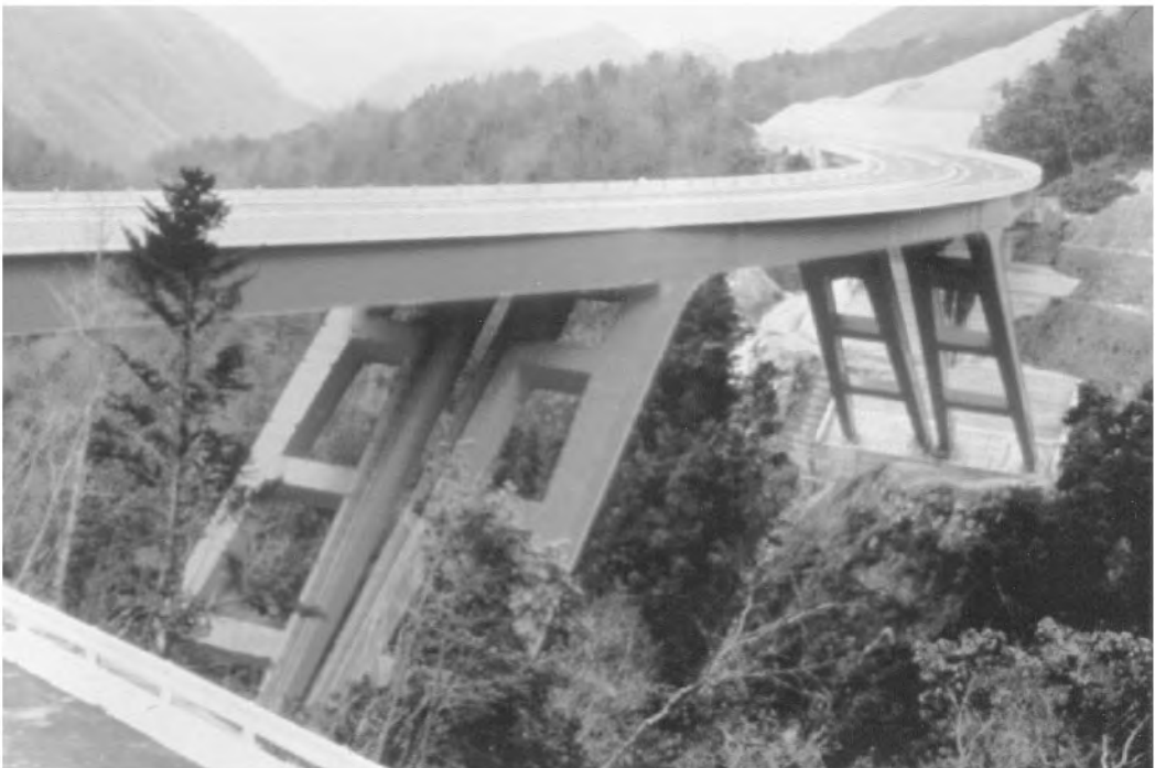
FIGURE 65.13 A typical \pi -shaped rigid frame bridge.
