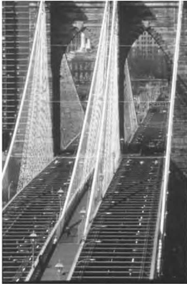
FIGURE 3.2 John Roebling's Brooklyn Bridge.
