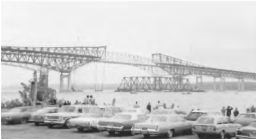
FIGURE 16.30 Float-in of suspended span.
