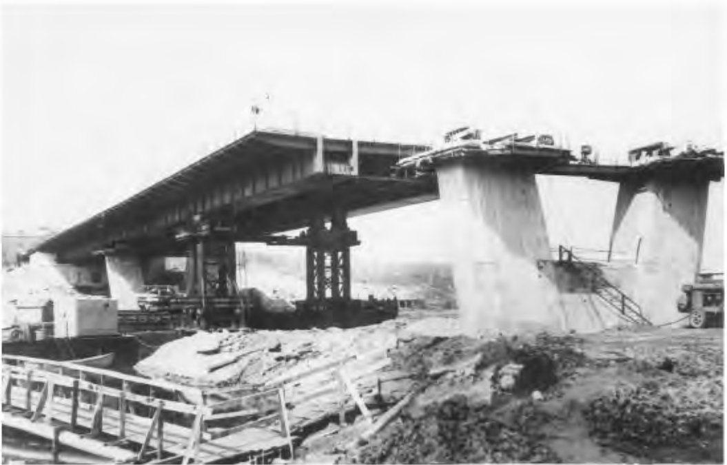
FIGURE 66.16 Superstructure launching for Moskva River Bridge in Krilatskoe.
