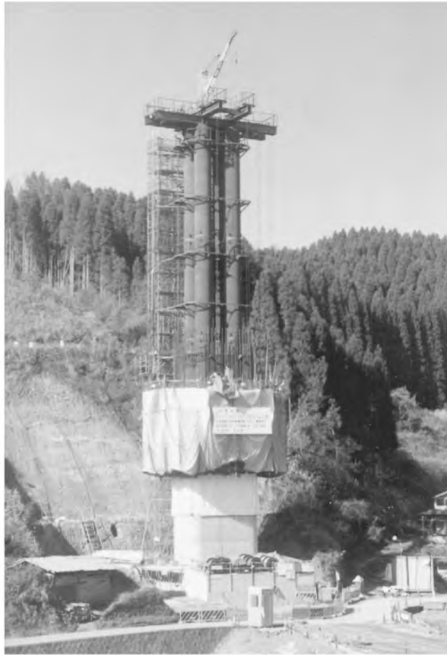
FIGURE 65.32 Piers of Shigehara Bridge. (Courtesy of Japan Highway Public Corporation.)
