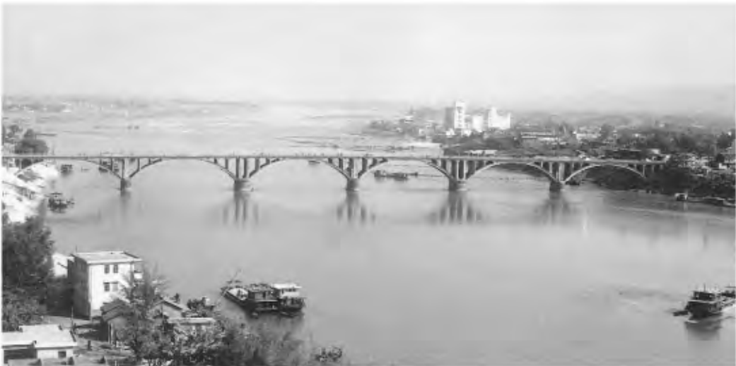
FIGURE 63.10 Heyuan Dong River Bridge.
