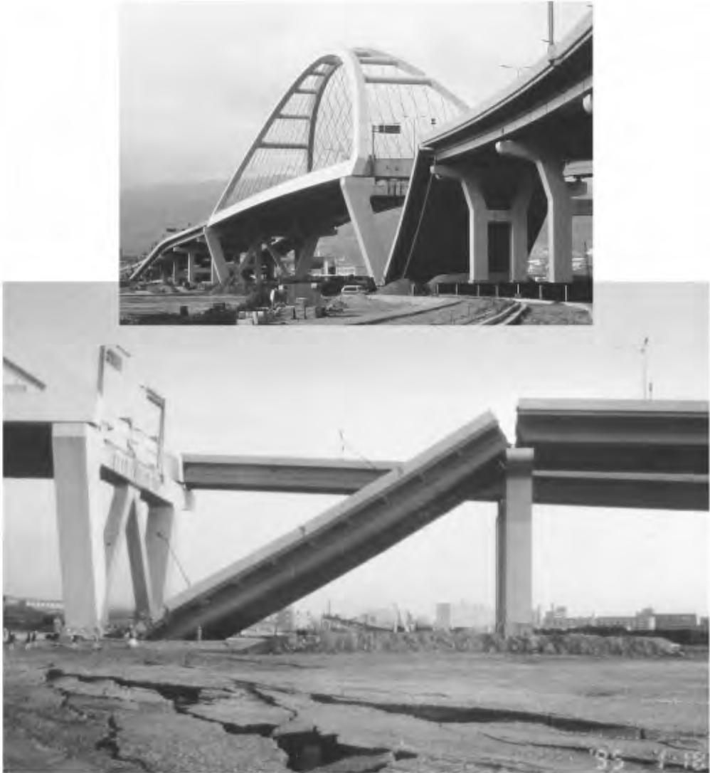
FIGURE 34.3 Nishinomiya-ko Bridge approach span collapse in the 1995 Hyogo-Ken Nanbu earthquake [Kobe Collection, EERC Library, University of California, Berkeley].
