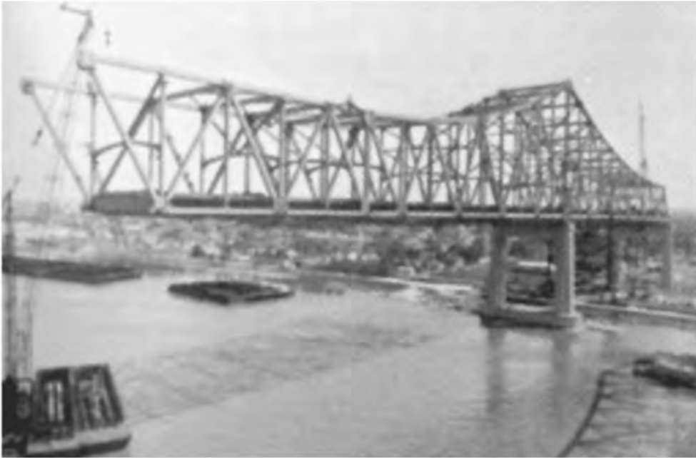
FIGURE 16.24 Advanced stage of cantilevering.
