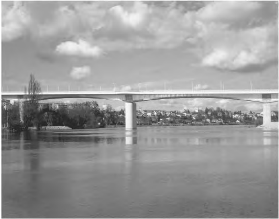
FIGURE 64.20 Dole Bridge. (Courtesy of Campenon Bernard.)
