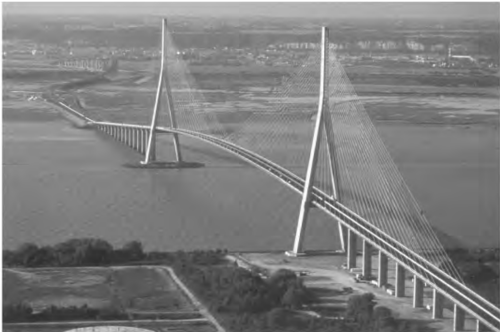
FIGURE 64.7 Normandie Bridge. (Courtesy of Campenon Bernard.)
