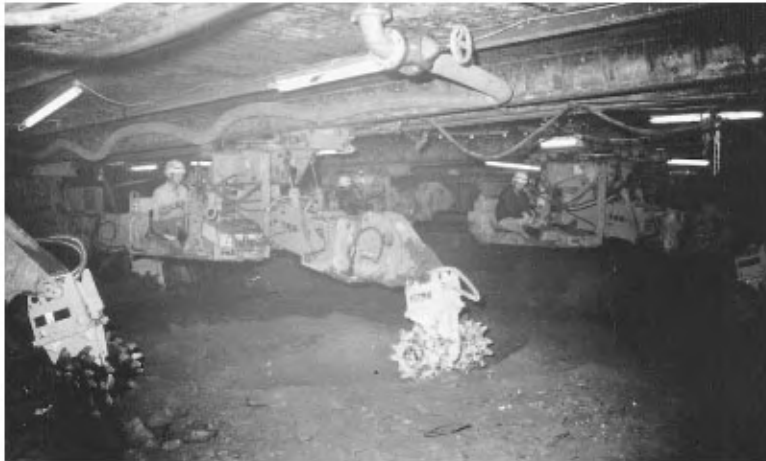
FIGURE 47.17 Excavating within pressurized working chamber of pneumatic caisson for Rainbow Suspension Bridge, Tokyo. (Photo courtesy of Shiraishi Corporation.)
