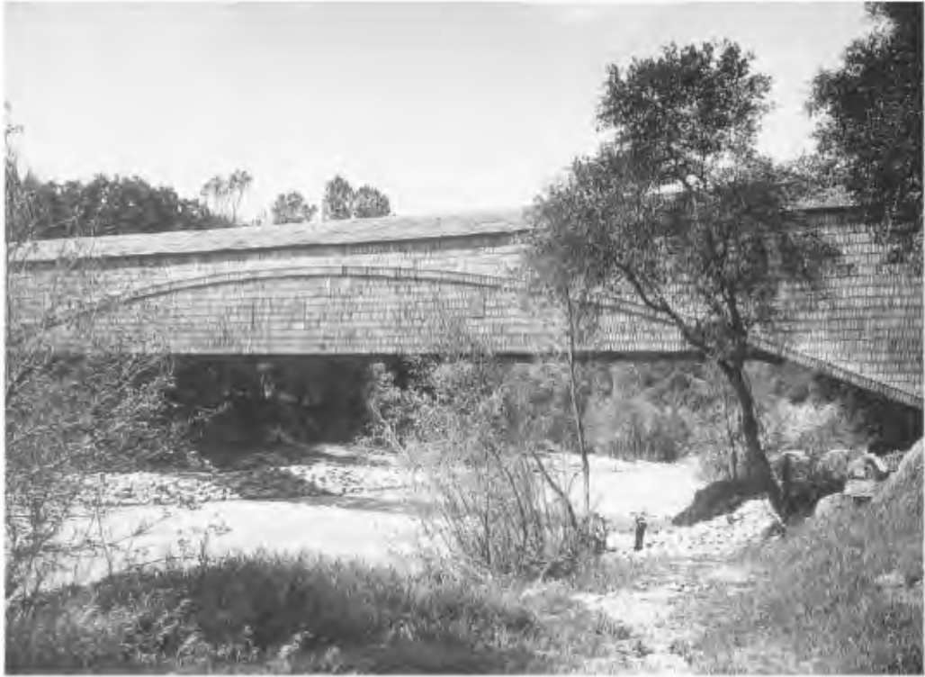
FIGURE 67.4 The Bridgeport Covered Bridge in California may be the longest single-span, 70.1 m, covered bridge in the world. The superstructure is a Burr arch superimposed on a Howe truss. It was a toll bridge built by David Wood in 1862, and was later purchased by the Virginia Turnpike Company. (Courtesy of California Department of Transportation.)
