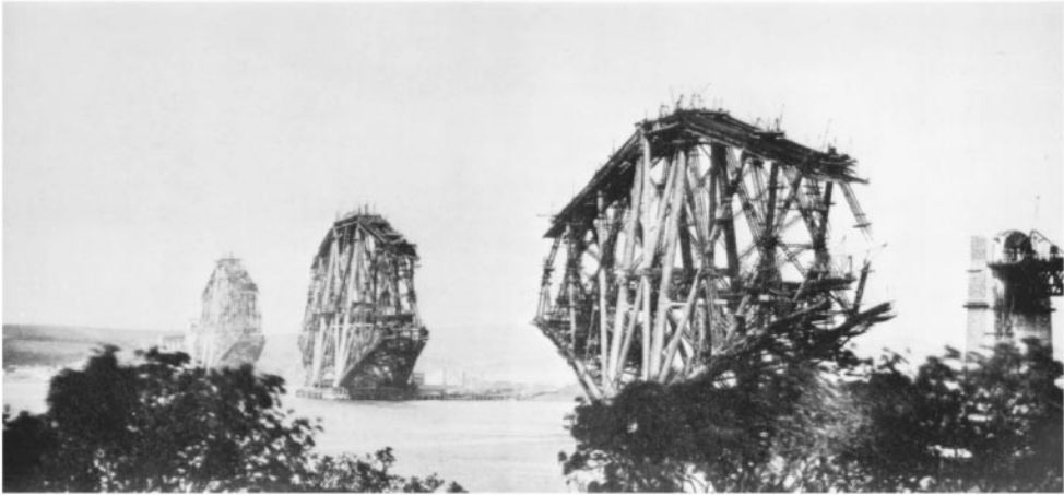
2. The massive cantilevers of the Forth bridge, shown under erection, were conceived in the shadow of the Tay bridge disaster.
