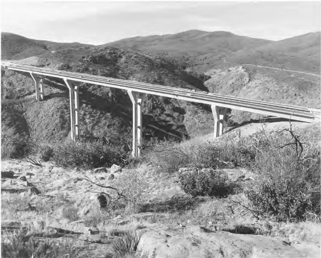
FIGURE 67.50 The California Department of Transportation experimented with and built its only segmental bridge, on Interstate Route 8 over Pine Valley in San Diego County in 1974. Bert Bezzone was the design engineer. The bridge received an American Society of Civil Engineers award in 1974. (Courtesy of California Department of Transportation.)
