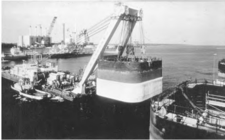
FIGURE 47.30 Setting prefabricated box caisson on which is mounted a temporary cofferdam, Great Belt Eastern Bridge, Denmark.
