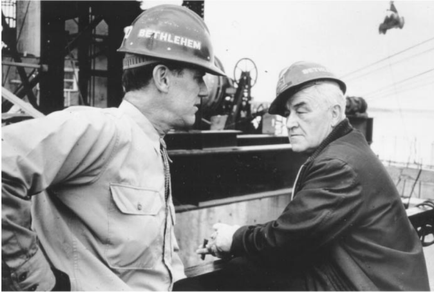
Figure 45.13 Visiting the work site. It is of first-order importance for bridge construction engineers to visit the site regularly and confer with the job superintendent and his foremen regarding practical considerations. Construction engineers have much to learn from the work forces in shop and field, and vice versa. (Courtesy of Bethlehem Steel Corporation.)
