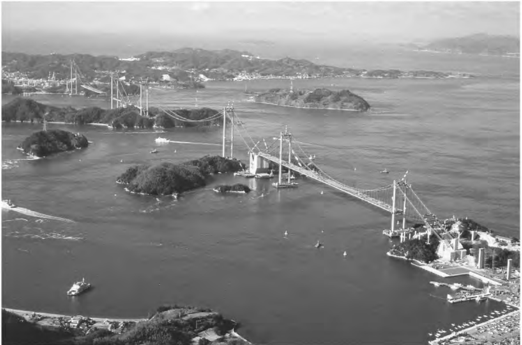
FIGURE 65.43 Kurushima Kaikyo Bridges.
