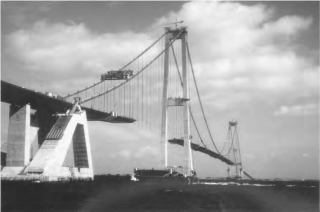
FIGURE 64.8 Storebælt Bridge. (Courtesy of Cowi Consult.)
