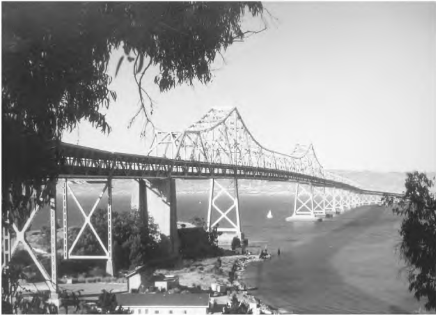
FIGURE 67.19 The San Francisco–Oakland Bay Bridge east, is part of the longer 13.3 km crossing composed of the west suspension span, a tunnel through Yerba Buena Island, and this cantilever truss east span. The seismic retrofitting solution at this site is to replace the bridge. There is local controversy over the type of span to be used. There are cost concerns, fear by San Francisco that an east side signature span could overshadow their west suspension span, and aspirations by Oakland that their city is also deserving of a signature span on their side of the Bay. (Courtesy of California Department of Transportation.)
