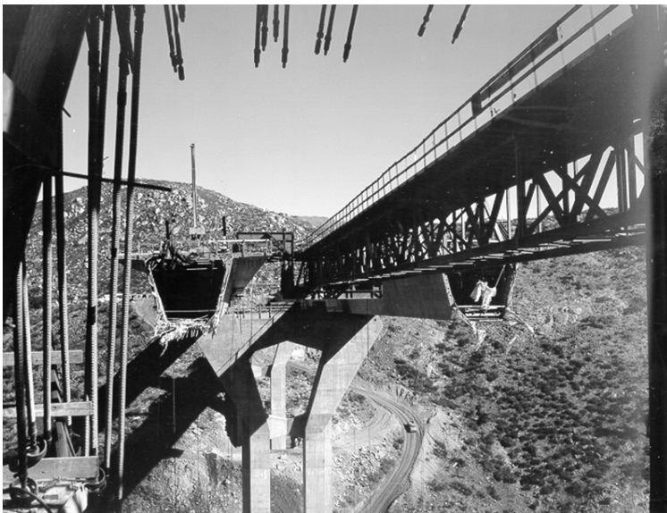
FIGURE 46.4 Pine Valley Creek Bridge — girder construction
