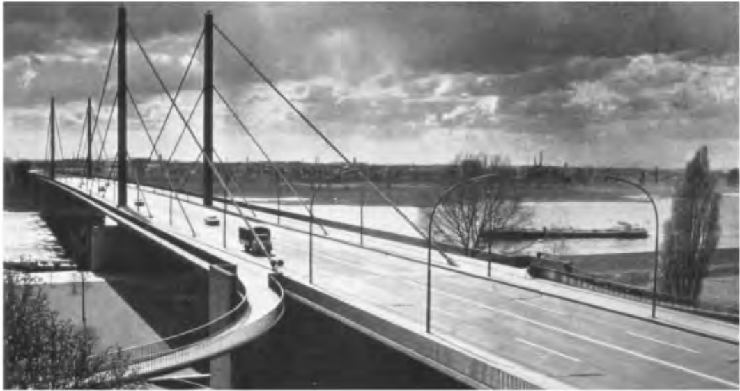
FIGURE 64.26 Theodor Heuss Bridge. (Source: Beyer, E., Brucknenbau, Beton Verlag, 1971. With permission.)
