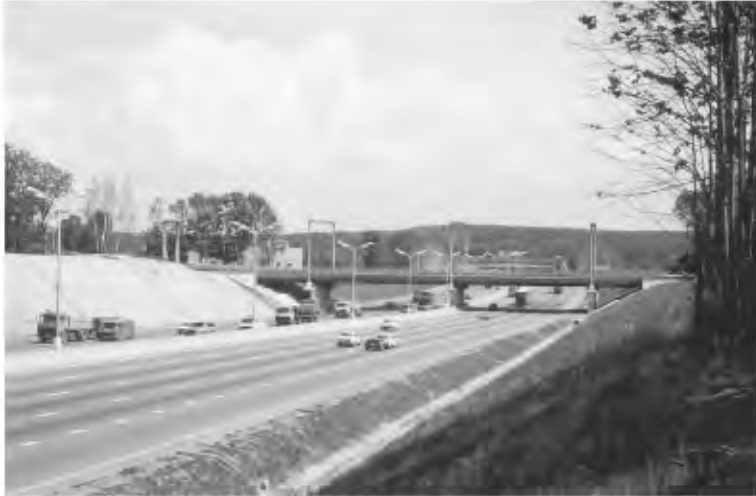
FIGURE 66.13 Paveletsky Railroad Overhead.
