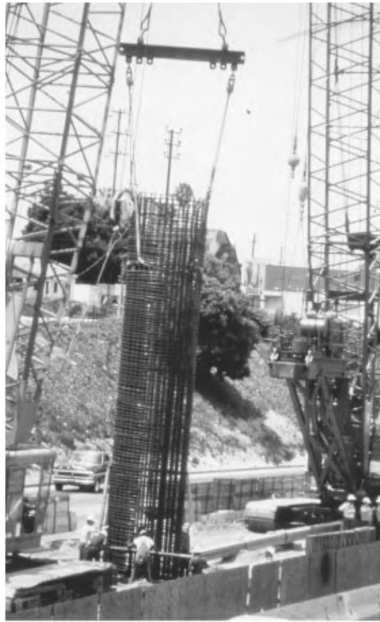
FIGURE 40.11 Column reinforcing steel cage.
