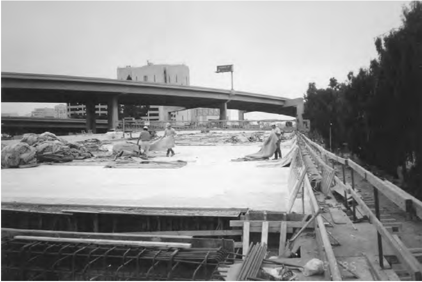
FIGURE 48.9 Bridge deck is being cured with moist rags.
