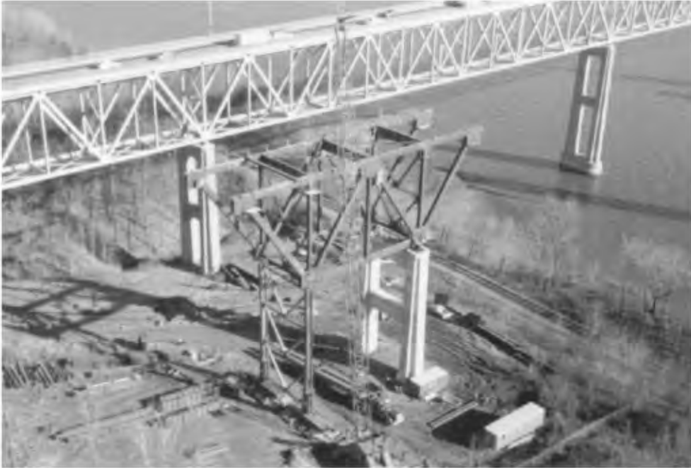
FIGURE 16.26 Use of falsework — 2.
