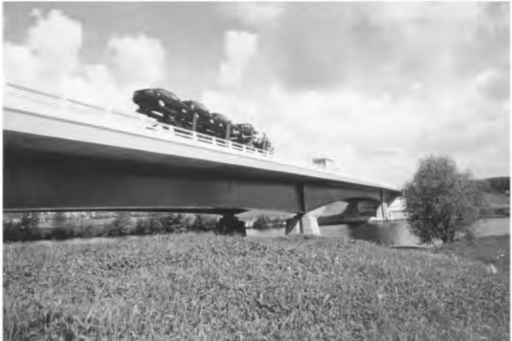
FIGURE 64.9 Oise Bridge. (Courtesy of Fred Boucher, SANEF.)
