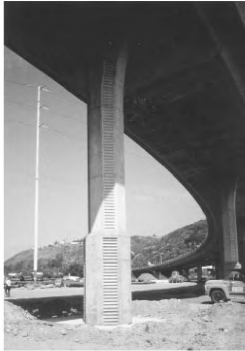
FIGURE 40.7 Concrete jacket column retrofit.
