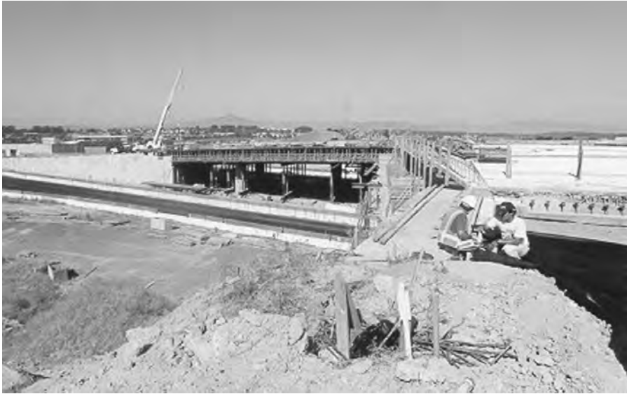
FIGURE 46.6 Falsework at I-80 HOV construction, Richmond, CA.
