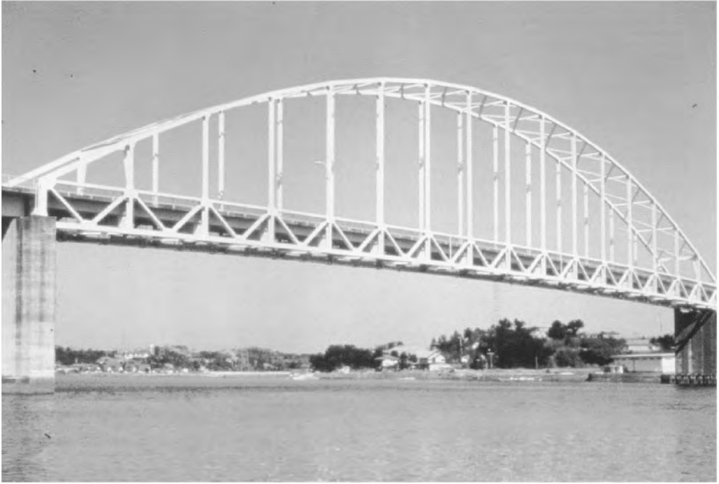
FIGURE 65.15 Ooyano Tsubasa Bridge.
