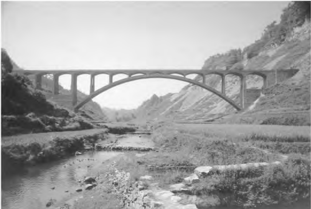
FIGURE 63.9 Wuchao River Bridge.
