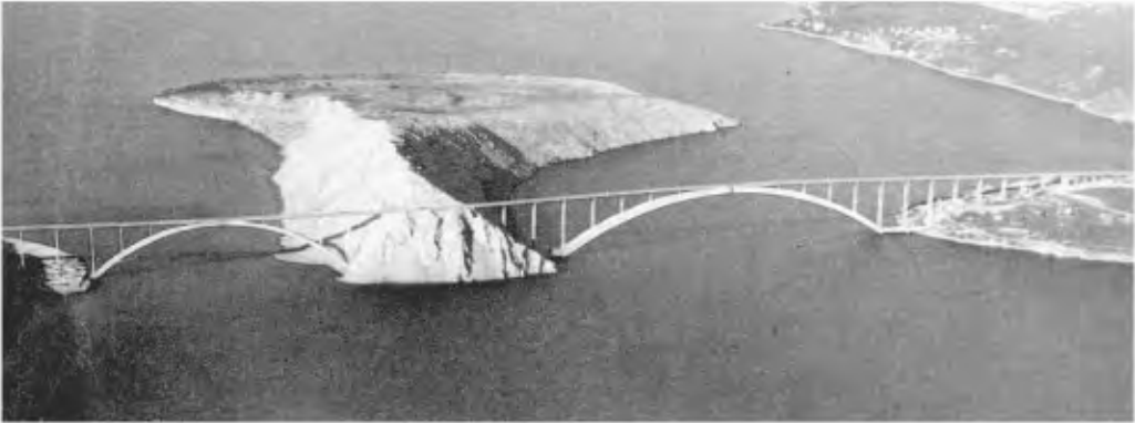
FIGURE 64.22 Kirk Bridges. (Source: Leonhardt, F., Ponts/Puentes — 1986 Presses Polytechniques Romandes. With permission.)
