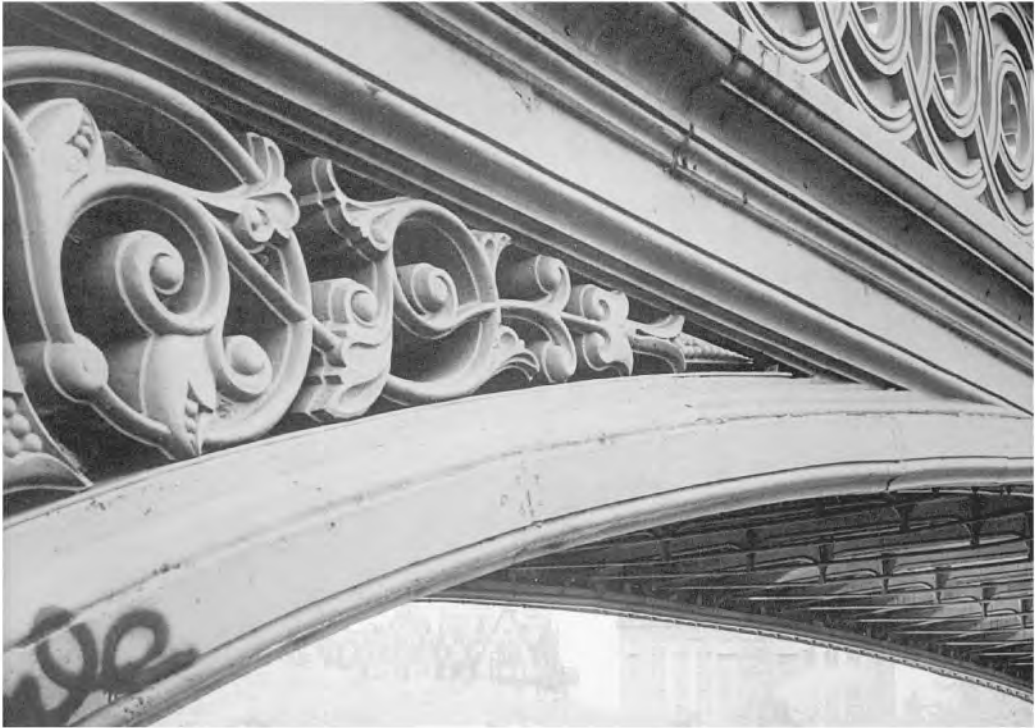
FIGURE 67.7 Bow Bridge in Central Park, New York, is the oldest surviving wrought-iron bridge in the United States, built in 1862. It has the longest span, 26.5 m, of five ornately decorated bridges in the park, all designed by Calvert Vaux and Jacob Wrey Mould. (Courtesy of American Society of Civil Engineers.)
