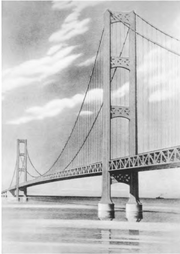
FIGURE 67.34 The Mackinac Straits Bridge was the winner of the 1958 American Institute of Steel Construction's Artistic Bridge Award and several gold medals. Its design provided a level of aerodynamic stability never before attained in a suspension bridge. It has a main span of 1158 m. It was designed by David Steinman and is owned by the Mackinac Bridge Authority in northern Michigan. (Courtesy of David Steinman.)
