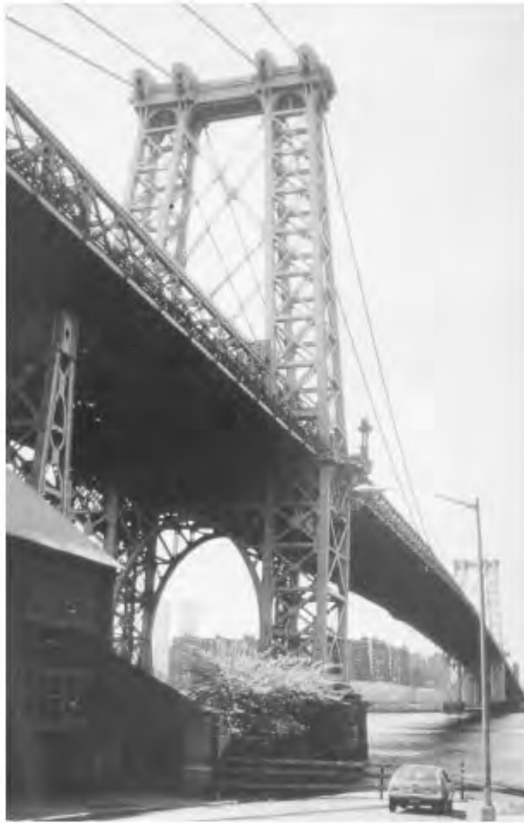
FIGURE 28.4 Williamsburg Bridge, New York. (Courtesy of Charles Seim.)
