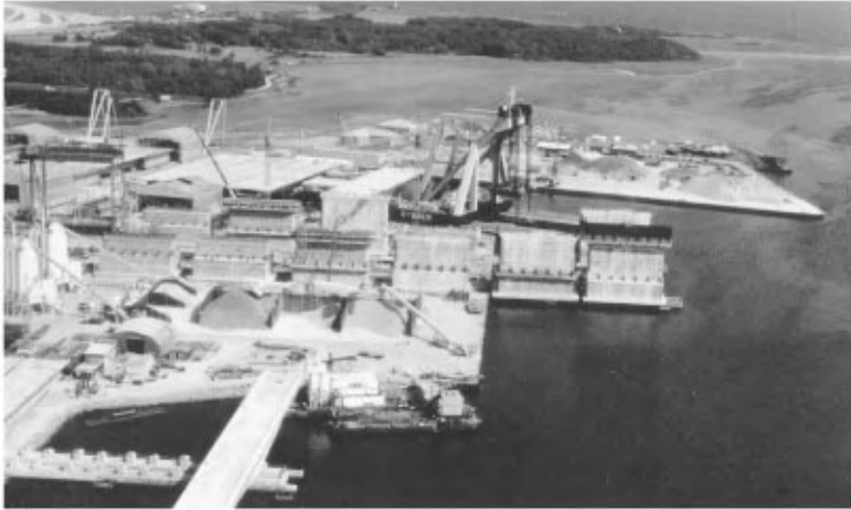
FIGURE 47.21 Prefabrication of box caisson piers for Great Belt Western Bridge, Denmark.
