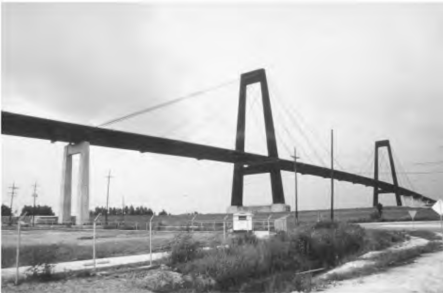
FIGURE 28.6 Luling Bridge, New Orleans, Louisiana. (Courtesy of Charles Seim.)
