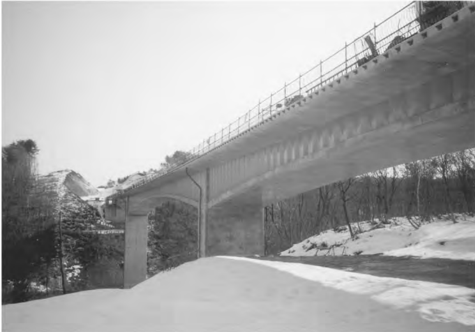
FIGURE 65.27 Hontani Bridge. (Courtesy of Japan Highway Public Corporation.)
