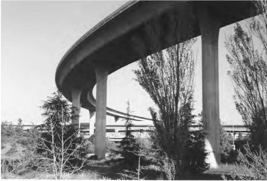
FIGURE 10.4 Prestressed box-girder bridge (I-280/110 Interchange, CA).
