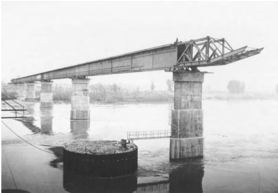
Figure 45.41c Leading end of north girder train is now supported on pier 5.
