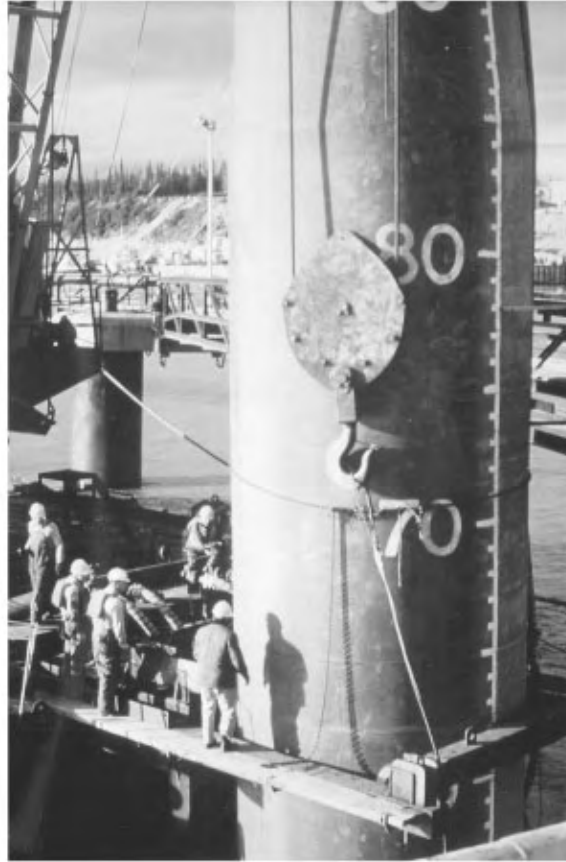
FIGURE 47.4 Large-diameter tubular steel pile being positioned.
