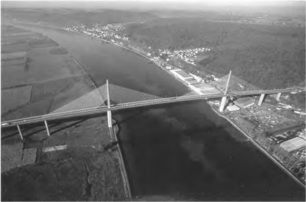
FIGURE 64.28 Brotonne Bridge. (Courtesy of Campenon Bernard.)
