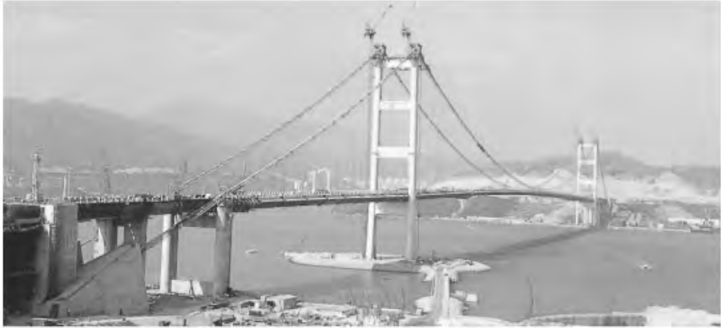
FIGURE 63.31 Hong Kong Tsing Ma Bridge.
