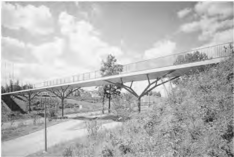
FIGURE 3.4 One of Jorg Schlaich's footbridges.
