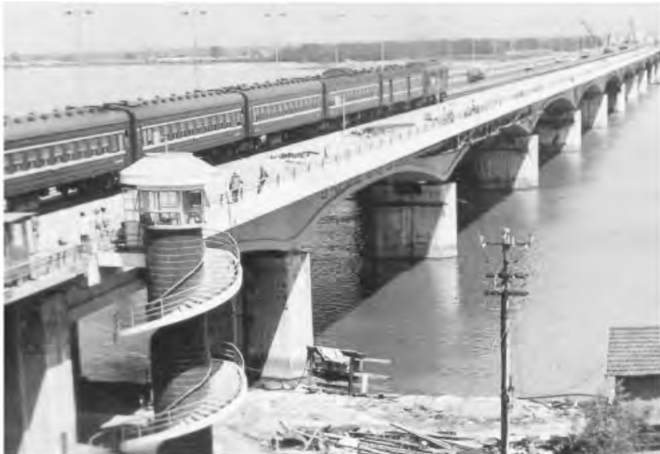
FIGURE 63.7 Second Qiantang River Bridge.
