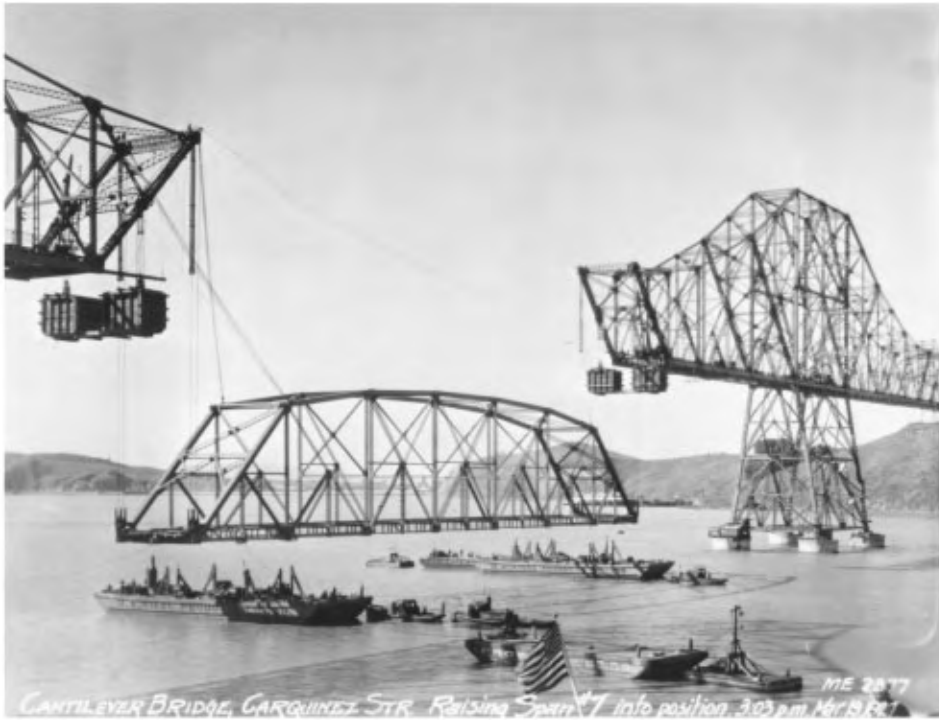
Figure 45.20 Raising of suspended span, Carquinez Strait Bridge, California, 1927. The 433 ft (132 m) suspended span, weighting 650 tons, was raised into position in 35 min., driven by four counterweight boxes having a total weight of 740 tons.
