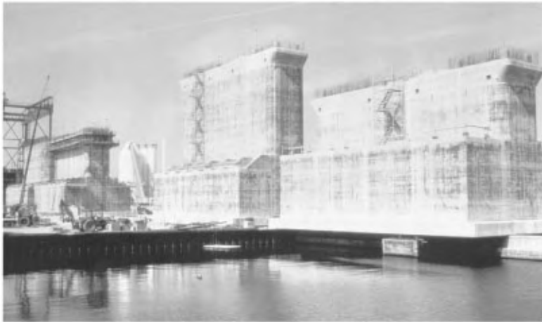
FIGURE 47.22 Prefabricated concrete box caissons are moved by jacks onto pier for load-out.
