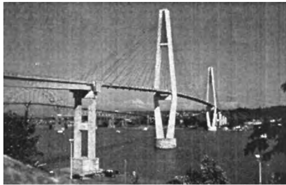
FIGURE 19.6 ALRT Skytrain Bridge.
