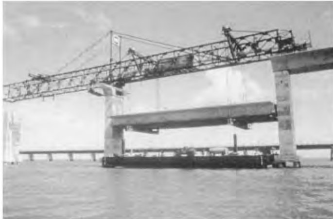
FIGURE 11.10 Lifting completed span of the Seven Mile Bridge, Florida, using an overhead truss .
