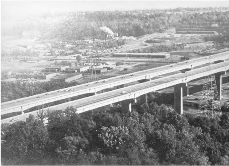
FIGURE 67.44 The Cuyahoga River Valley Bridge built in 1980 for the Ohio Turnpike Authority earned an AISC award that year. It was designed by Howard Needles Tamman Bergendoff. (Courtesy of American Institute of Steel Construction.)
