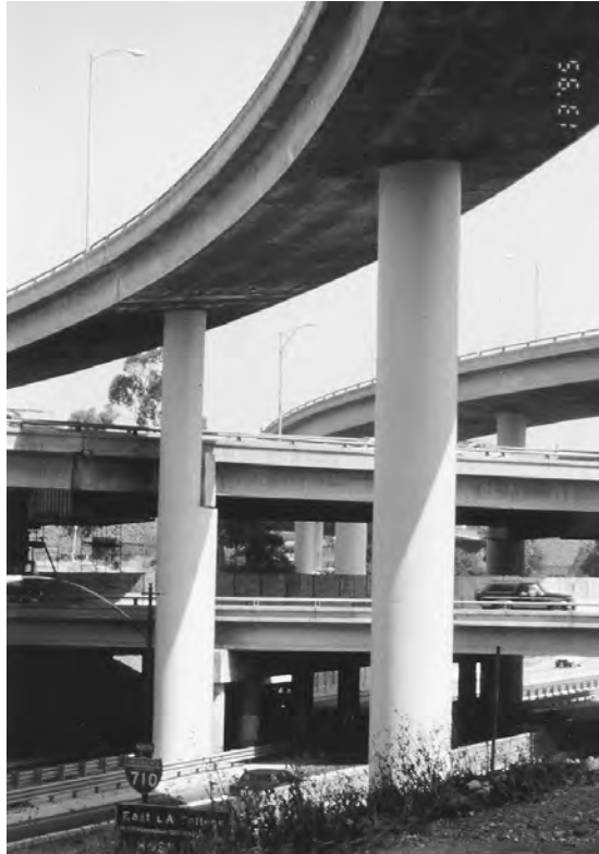
FIGURE 40.17 Completed seismic retrofit of I-5/710 interchange in Los Angeles.
