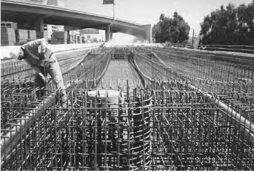
FIGURE 10.2 A post-tensioned box-girder bridge under construction.
