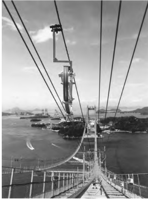
FIGURE 18.30 Aerial spinning for the Shimotsui-Seto bridge. (Courtesy of Honshu-Shikoku Bridge Authority.)
