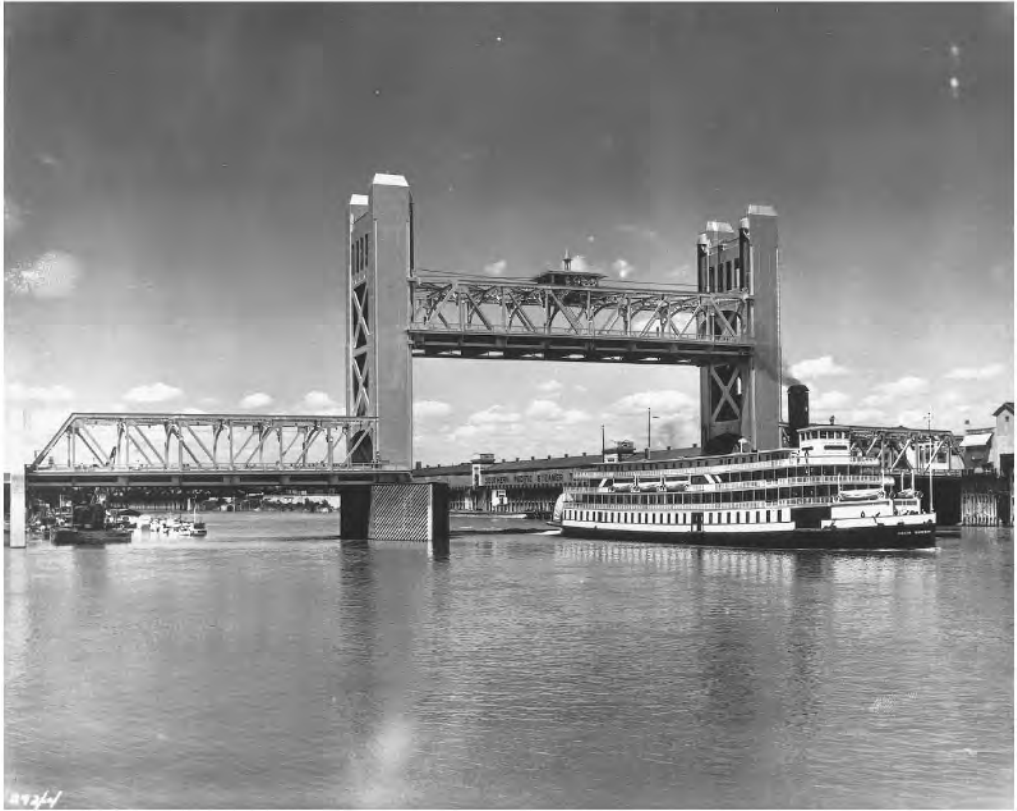
FIGURE 67.36 The Tower Bridge in Sacramento earned an AISC design award in 1936, the year in which it was built. This unique lift span is clad in steel plate to cover the moving parts. It was designed by Leonard Hollister of the California Division of Highways. (Courtesy of California Department of Transportation.)
