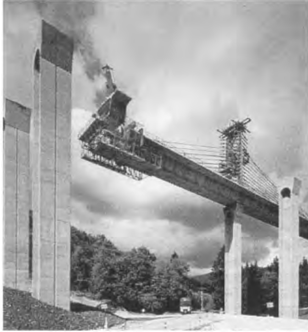
FIGURE 11.7 Fréburge Viaduct, France—erection with movable stay tower.
