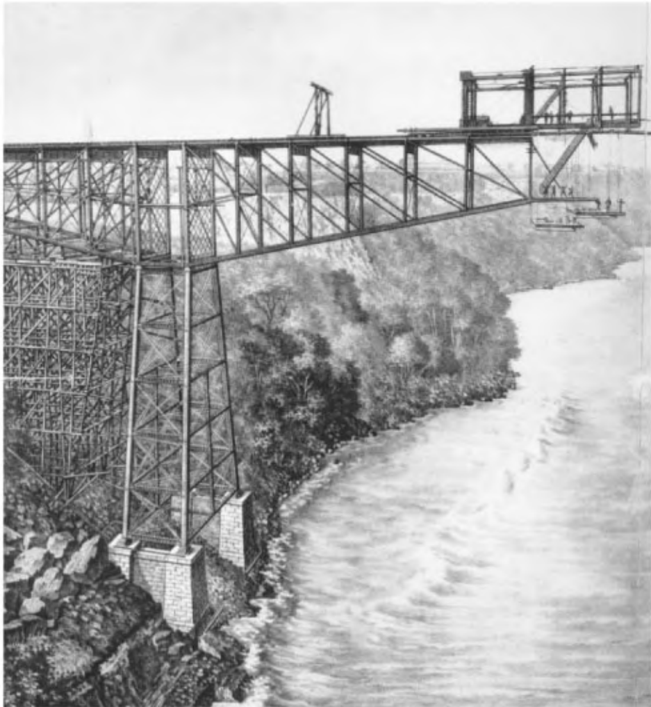
Figure 45.17 Niagara River railway cantilever truss bridge, near Niagara Falls, New York, 1883. Massive wood erection traveler constructed side span on falsework, then cantilevered half of main span to midspan. Erection of other half of bridge was similar. First modern-type cantilever bridge, with 470 ft (143 m) clear main span having a 120 ft (37 m) center suspended span.
