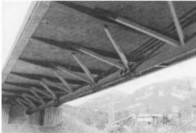
FIGURE 11.22 The Roize Bridge, France — erection of steel bottom chord and webs.
