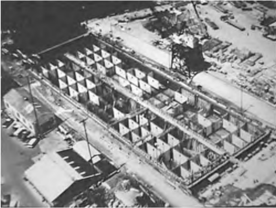
FIGURE 22.16 Construction in a graving dock.
