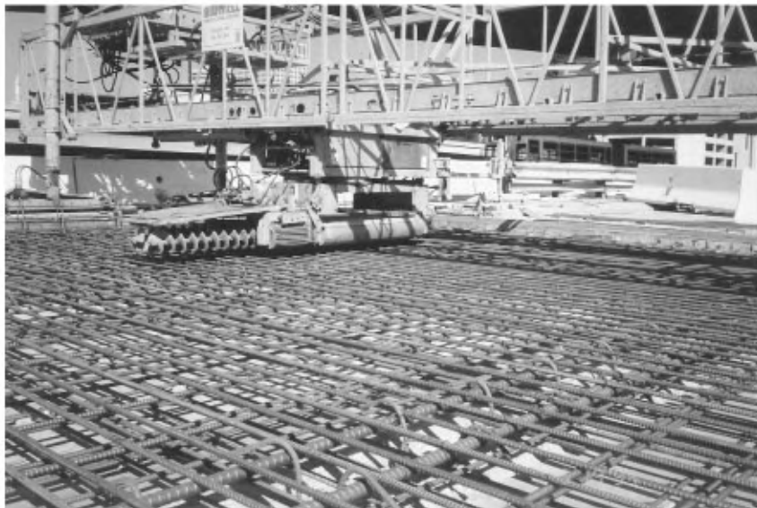
FIGURE 48.5 Bridge deck reinforcement with bidwell finishing machine.
