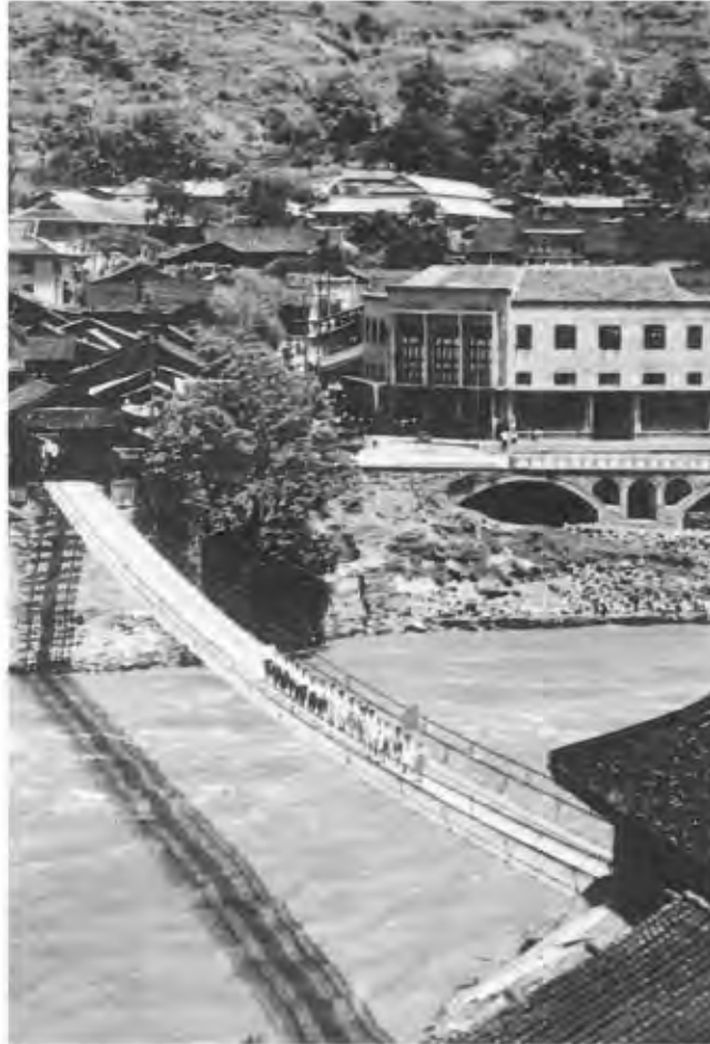
FIGURE 63.3 Luding Iron-Chain Bridge.
