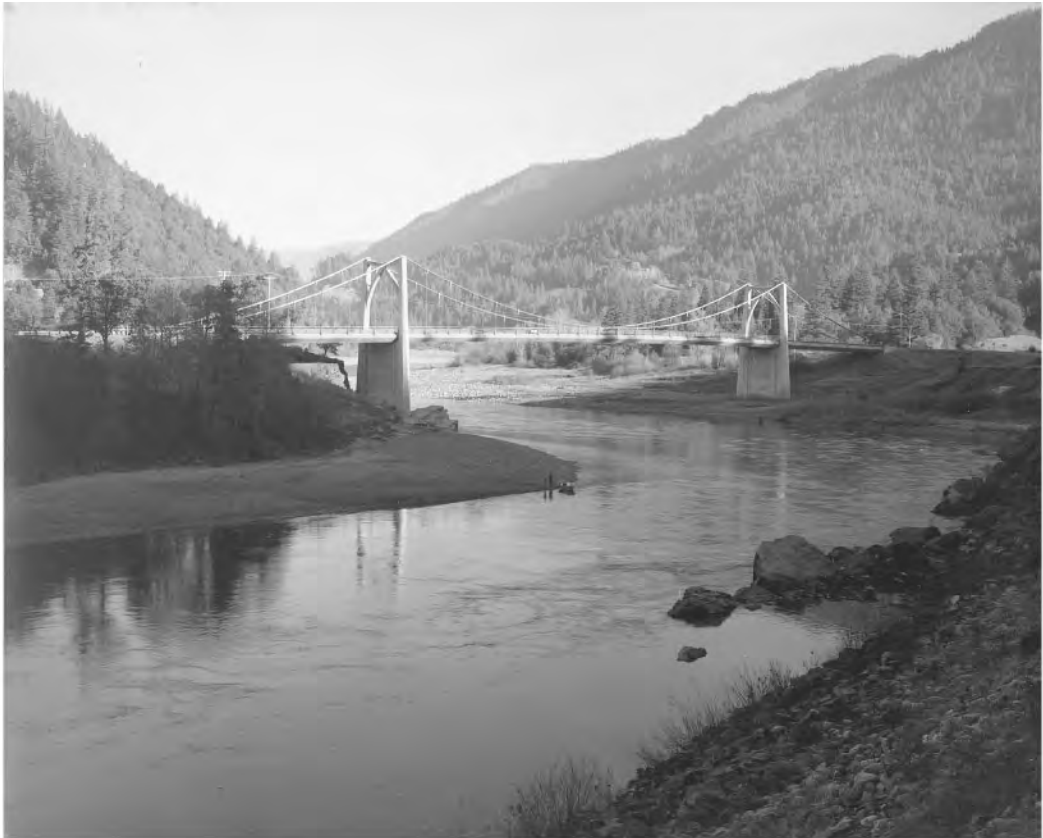
FIGURE 67.47 The Klamath River crossing at Orleans in Northern California is a picturesque setting on a back road. There have been seven structures at this site, one burned and five have been washed away during major floods. The current steel box girder suspension span has lasted longer than any of its predecessors. Built in 1967, it was designed by Bert Bezzone of the California Division of Highways. (Courtesy of California Department of Transportation.)
