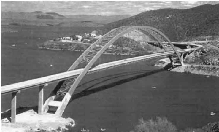
FIGURE 17.10 Roosevelt Lake Bridge, Arizona.
