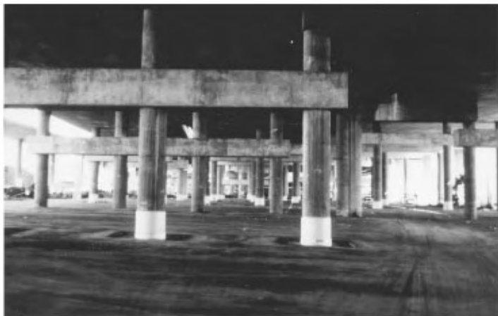
FIGURE 40.10 Steel jackets and bond beam — Santa Monica Freeway.
