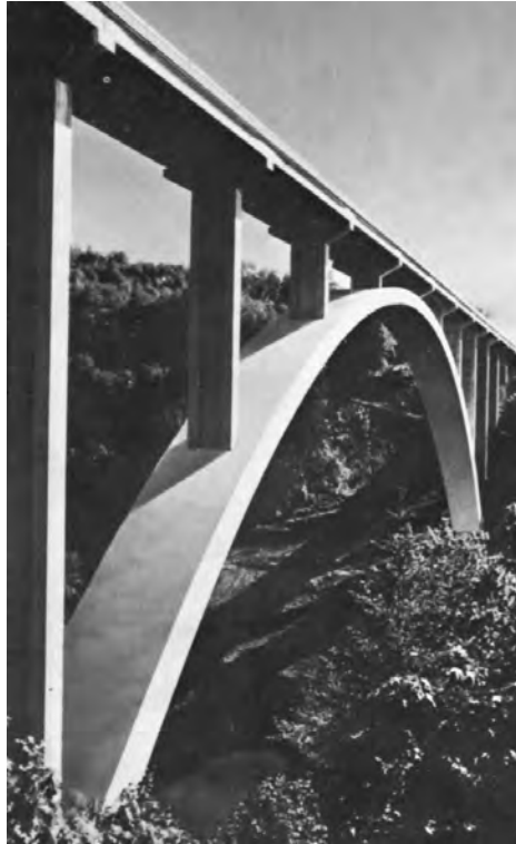
FIGURE 17.5 Cowlitz River concrete arch.
