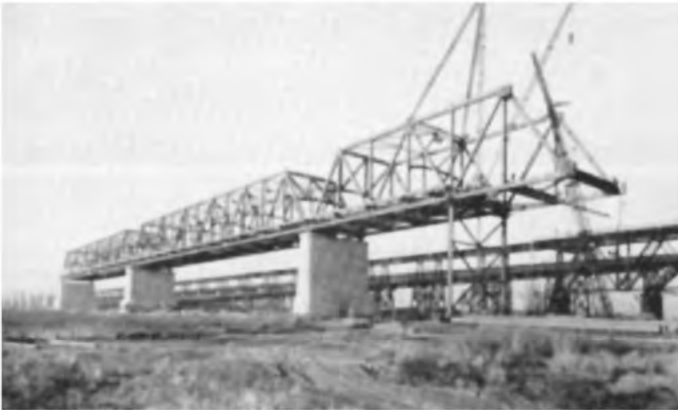
FIGURE 16.25 Use of falsework — 1.
