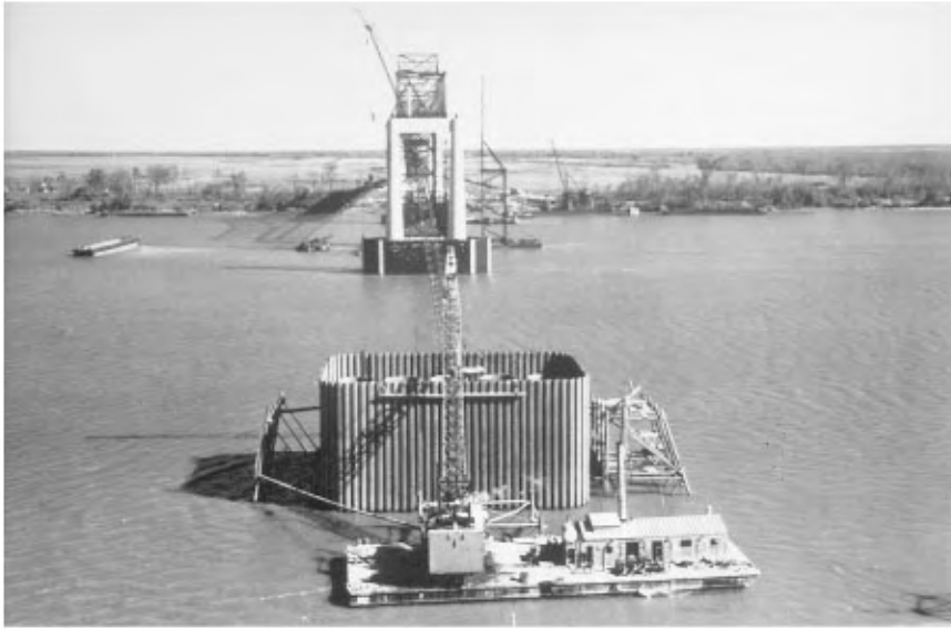
FIGURE 47.15 Open-caisson positioned within steel jackets on “pens.”
