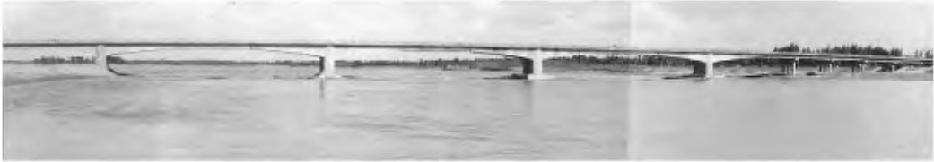
FIGURE 63.15 Qingtongxia Yellow River Highway Bridge.
