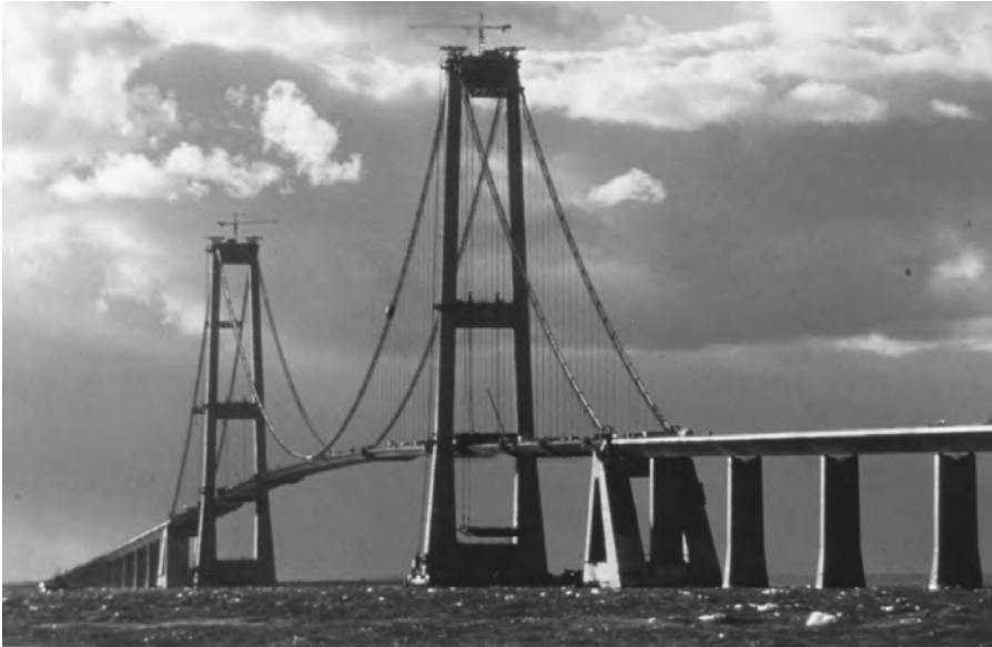
FIGURE 4.4 Storebælt East Bridge.
