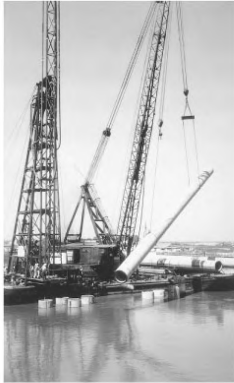
FIGURE 47.6 Large-diameter prestressed concrete pile, Napa River Bridge, California.
