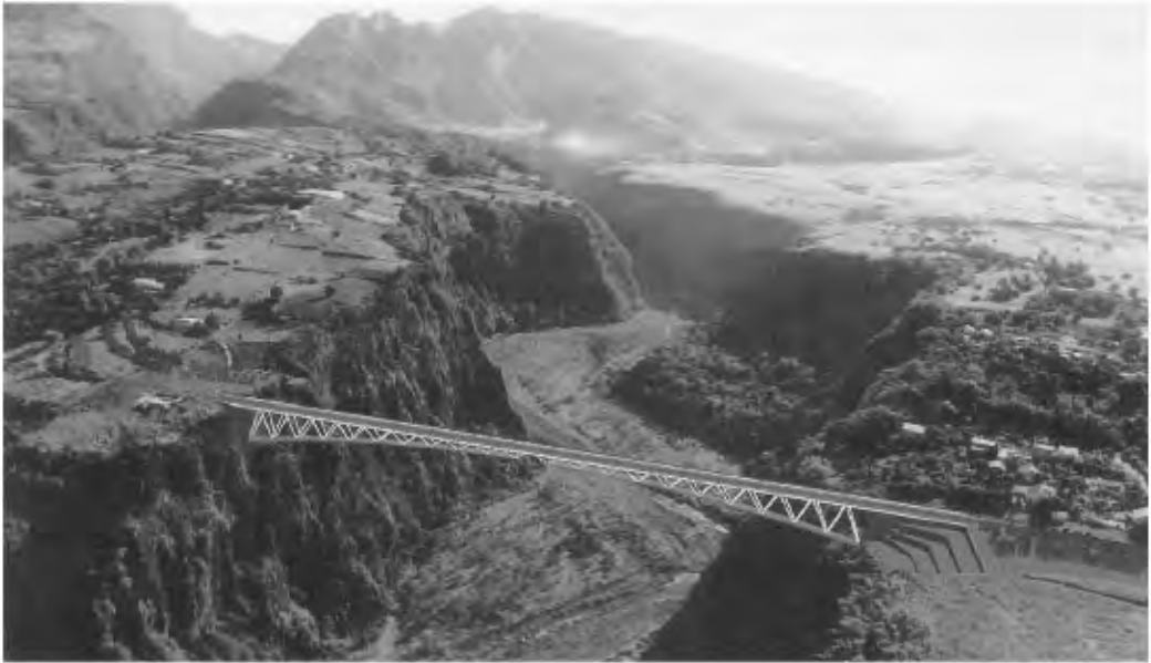
FIGURE 64.25 Bras de la Plaine Bridge. (Courtesy of Jean Muller International.)
