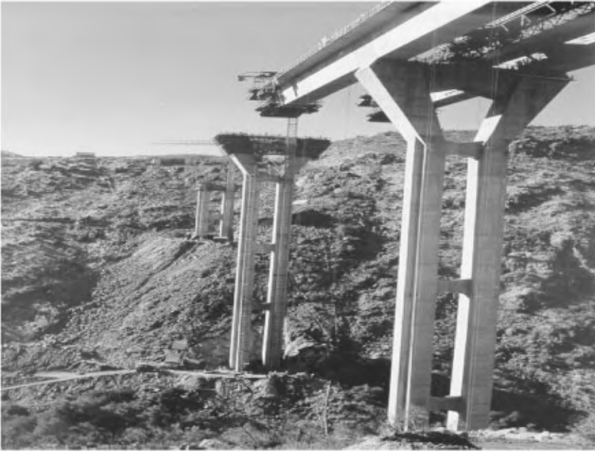
FIGURE 46.3 Pine Valley Creek Bridge — pier construction
