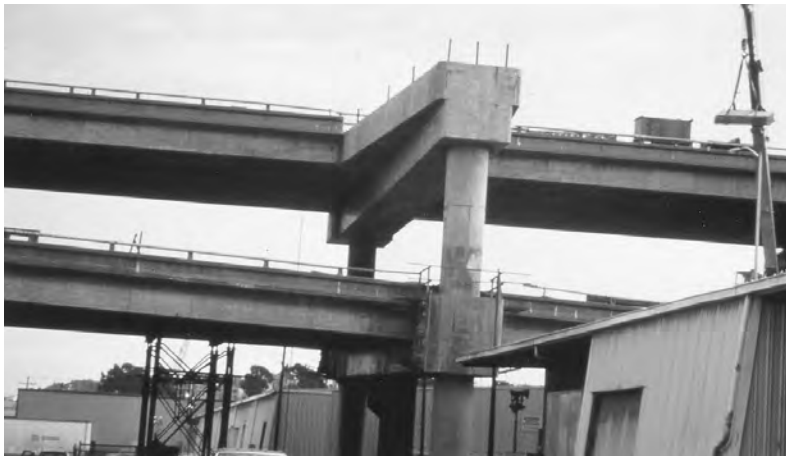
FIGURE 40.14 Completed retrofitted structures.
