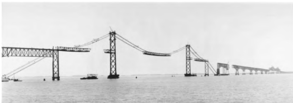
Figure 45.6 Suspension spans of first Chesapeake Bay Bridge, Maryland, 1952. Deck steelwork is under erection and is about 50% complete. A typical four-panel through-truss deck section, weighing about 100 tons, is being picked in west side span, and also in east side span in distance. Main span is 1600 ft (488 m) and side spans are 661 ft (201 m); towers are 324 ft (99 m) high. Cables are 14 in. (356 mm) in diameter and are made up of 61 helical bridge strands each (see Figure 45.8 ).
