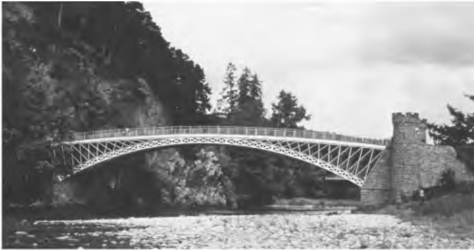
FIGURE 3.1 Thomas Telford's Craigellachie Bridge.
