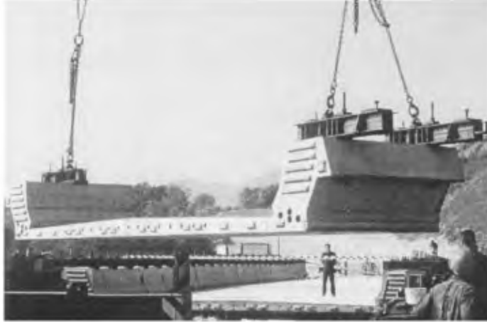
FIGURE 11.13 Channel Bridge, France, under construction.
