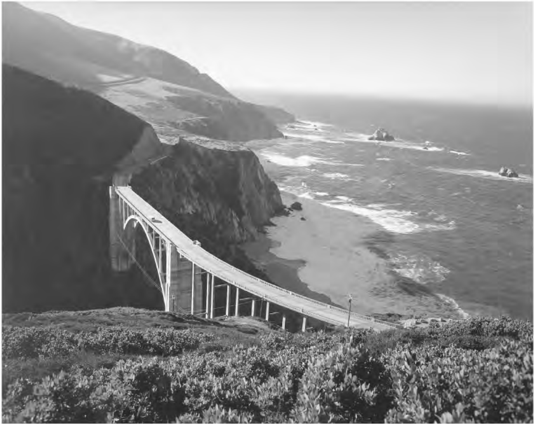
FIGURE 67.24 Bixby Creek Bridge on the Monterey Coast in California is one of the most picturesque and photographed bridges in California. This Monterey Coast Highway was the first designated Scenic Highway in California, in 1961. The route is also the first to be designated an All American Road. Built in 1932, it has a main span of 109.7 m and is 79.2 m above the streambed. Construction required 26 stories of falsework. It was designed by Harvey Stover of the California Division of Highways. Seismic retrofitting is complicated due to aesthetic restrictions established by historical preservation codes. (Courtesy of California Department of Transportation.)
