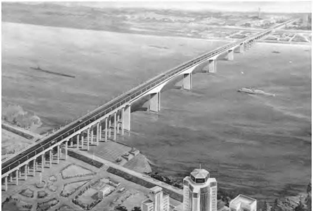
FIGURE 63.19 Huangshi Yangtze River Bridge.
