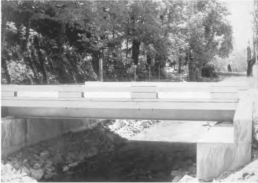
FIGURE 67.54 Laurel Lick Bridge is the second all-composite bridge to be completed. It is owned by the West Virginia Department of Highways and was built experimentally in conjunction with West Virginia University, in 1997. (Courtesy of West Virginia Department of Highways.)
