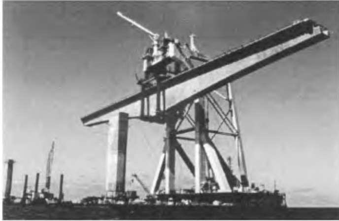
FIGURE 11.52 Confederation Bridge, Canada — floating crane.
