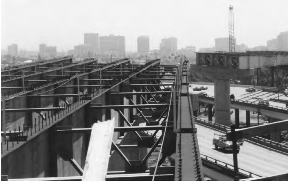
FIGURE 12.1 Steel–concrete composite girder bridge (I-880 Replacement, Oakland, California)
