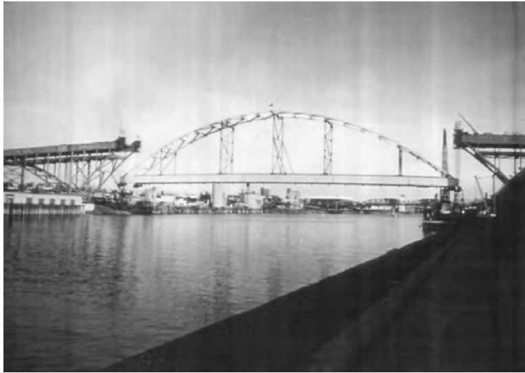
FIGURE 17.15 Fremont tied arch being lifted into place.
