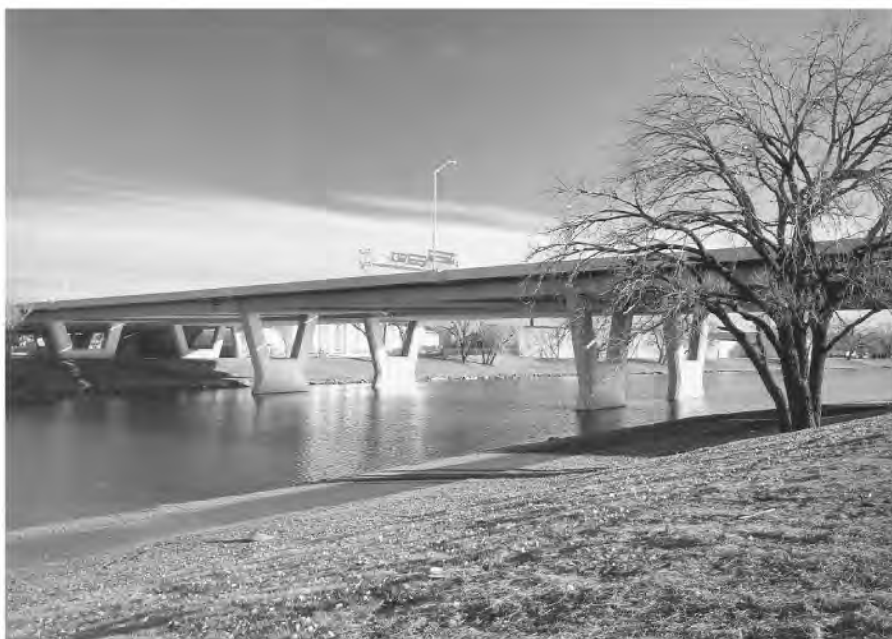
FIGURE 67.42 Kellogg Central Business District Viaduct in Wichita, Kansas, designed by Howard Needles Tamman Bergendoff, won a Portland Cement Association award in 1996. (Courtesy of Howard Needles Tamman Bergendoff.)
