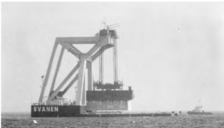
FIGURE 47.31 Setting 7000-ton prefabricated box caisson, Great Belt Western Bridge, Denmark.
