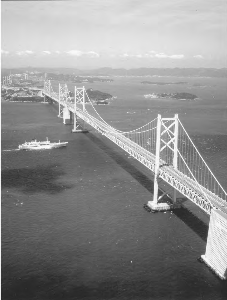
FIGURE 65.39 Kita-Bisan Seto and Minami-Bisan Seto Bridges.
