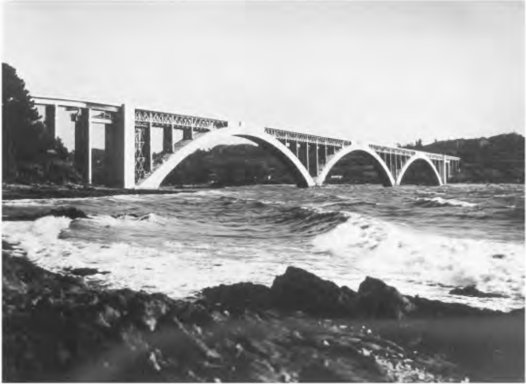
FIGURE 64.4 Albert Louppe Bridge. (Courtesy of Jean Muller International.)
