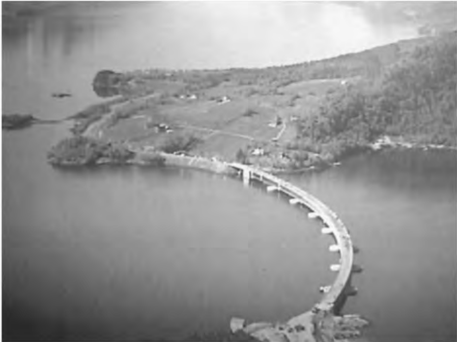
FIGURE 22.2 The Bergsoysund floating bridge.
