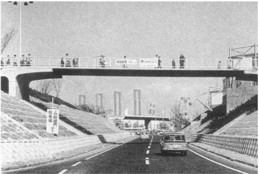
FIGURE 65.23 International Expo No. 9 Bridge.
