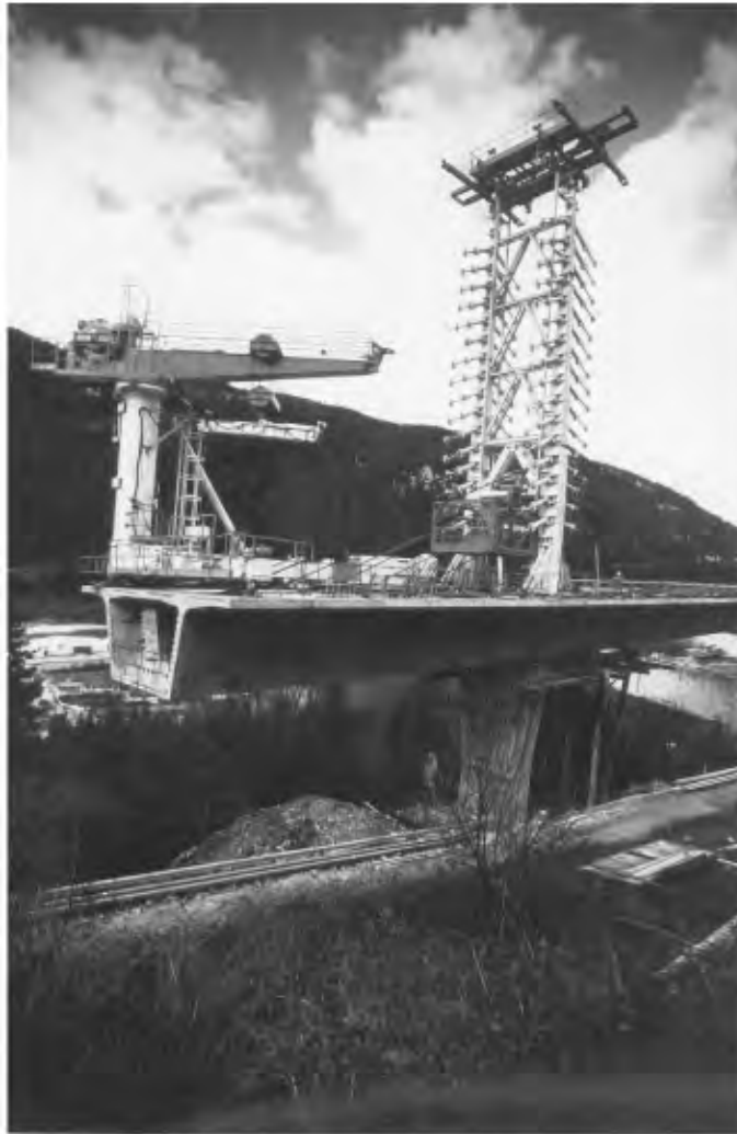
FIGURE 64.14 The second Neyrolles viaduct. (Courtesy of Campenon Bernard.)
