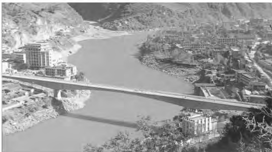
FIGURE 63.6 Liuku Nu River Bridge.
