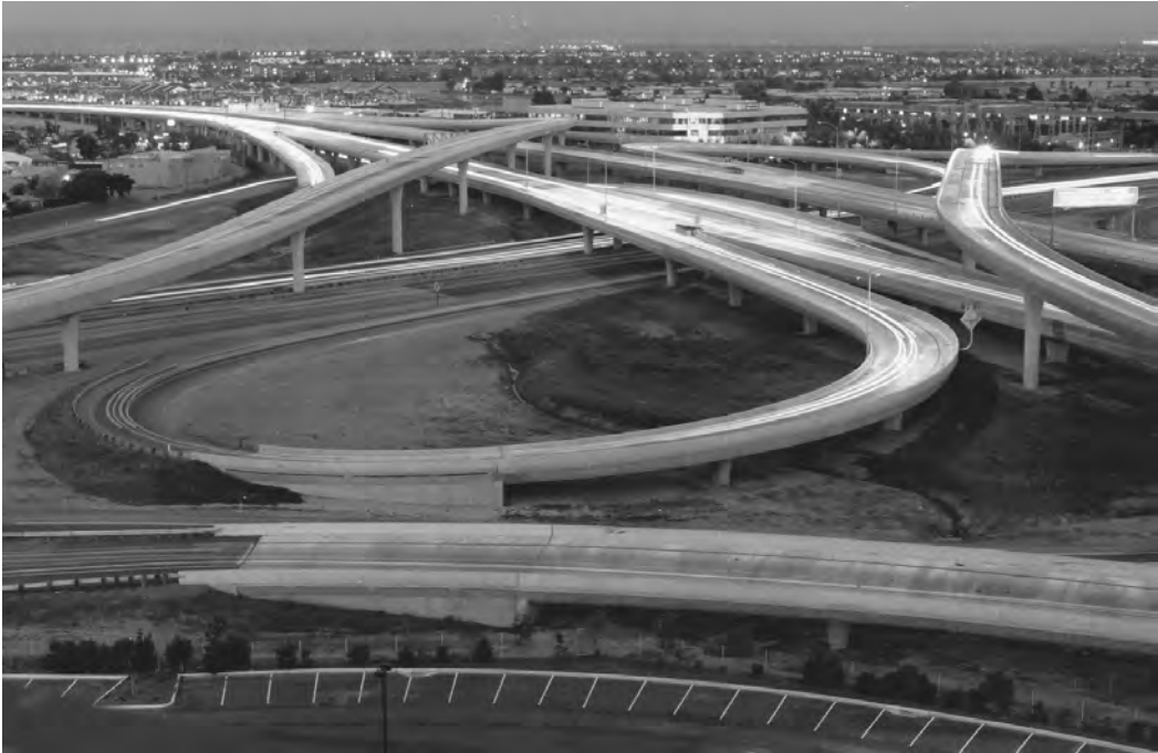
FIGURE 15.6 Curved concrete box-girder bridges — Route 92/101 Interchange, San Mateo, California.
