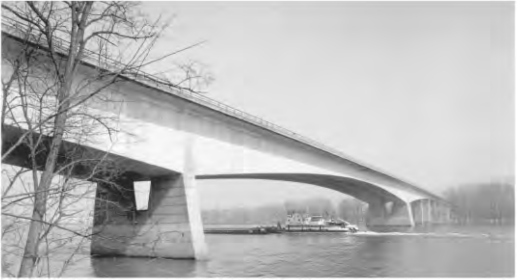
FIGURE 64.5 Bendorf Bridge. ( Source: Leonhardt, F, Ponts/Puentes — 1986 Presses Polytechniques Romandes. With permission.)
