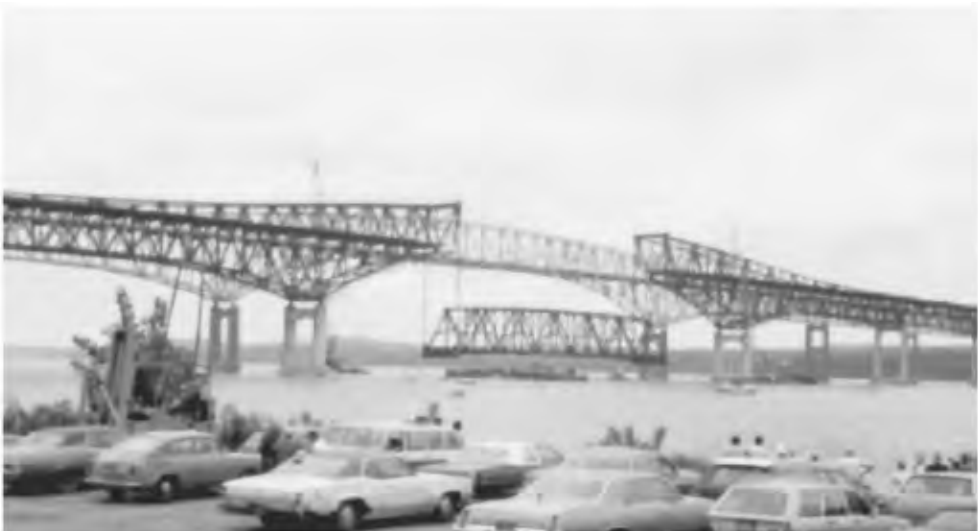
FIGURE 16.31 Lift of suspended span.
