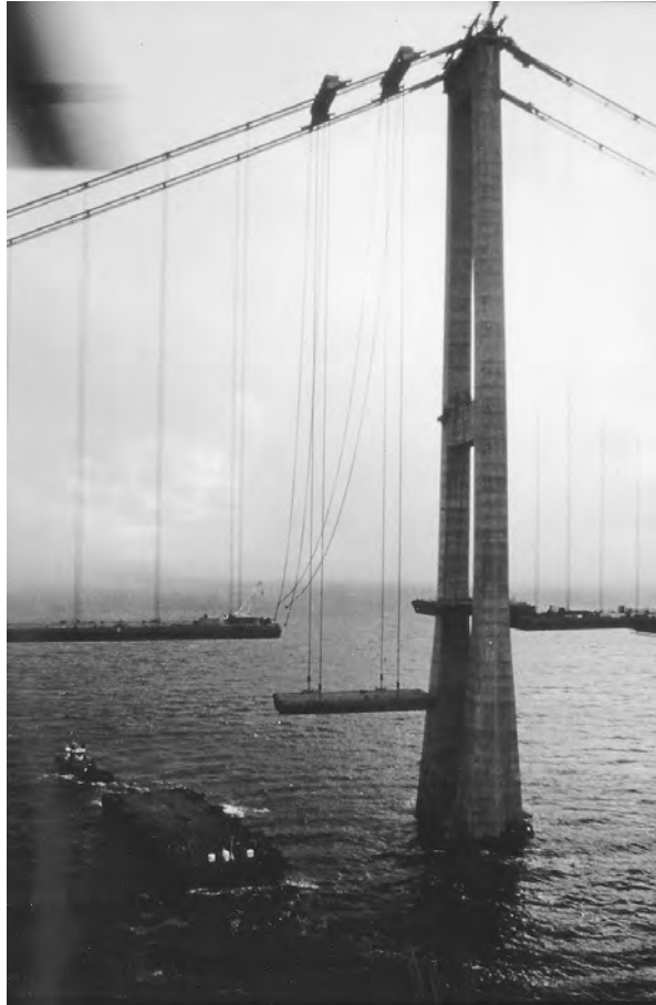
FIGURE 28.13 Great Belt Bridge, Denmark. (Courtesy of Ben C. Gerwick, Inc.)
