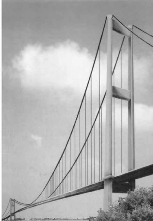
FIGURE 63.32 Jiangyin Yangtze River Bridge.
