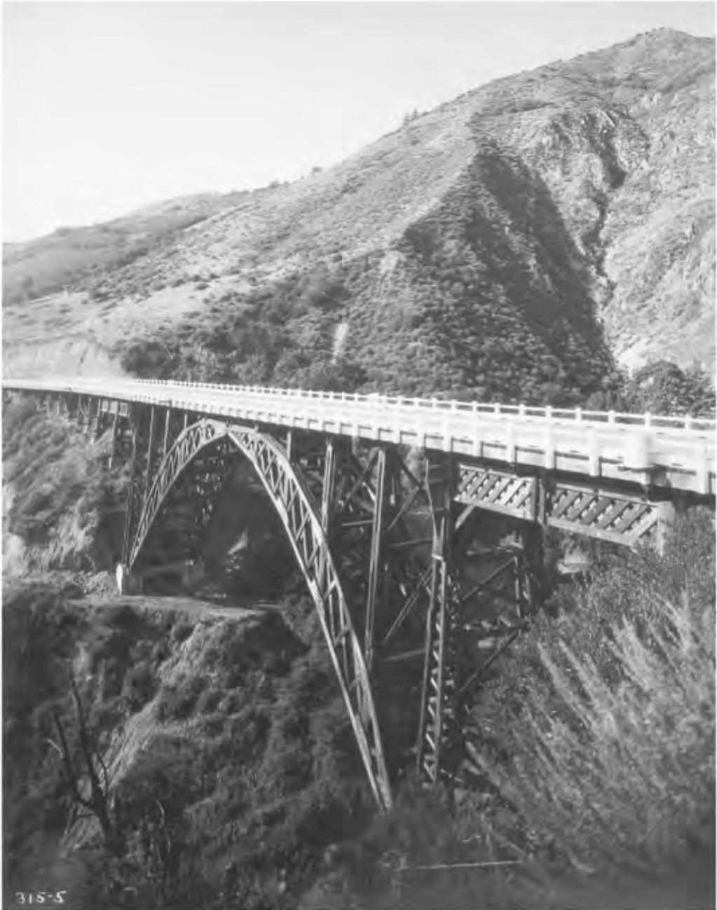
FIGURE 67.3 Dolan Creek Bridge on the Monterey Coast in California was built in 1932. This is one of only two three-pin timber arch bridges ever built on the California State Highway system. It lasted only a few years, and has since been replaced with a concrete bridge in 1961. (Courtesy of California Department of Transportation.)
