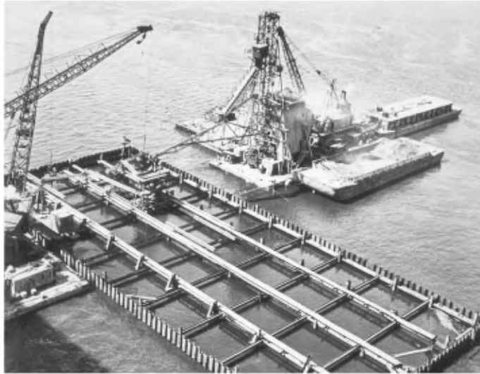
FIGURE 47.9 Large steel sheet pile cofferdam for Second Delaware Memorial Bridge, showing bracing frames.
