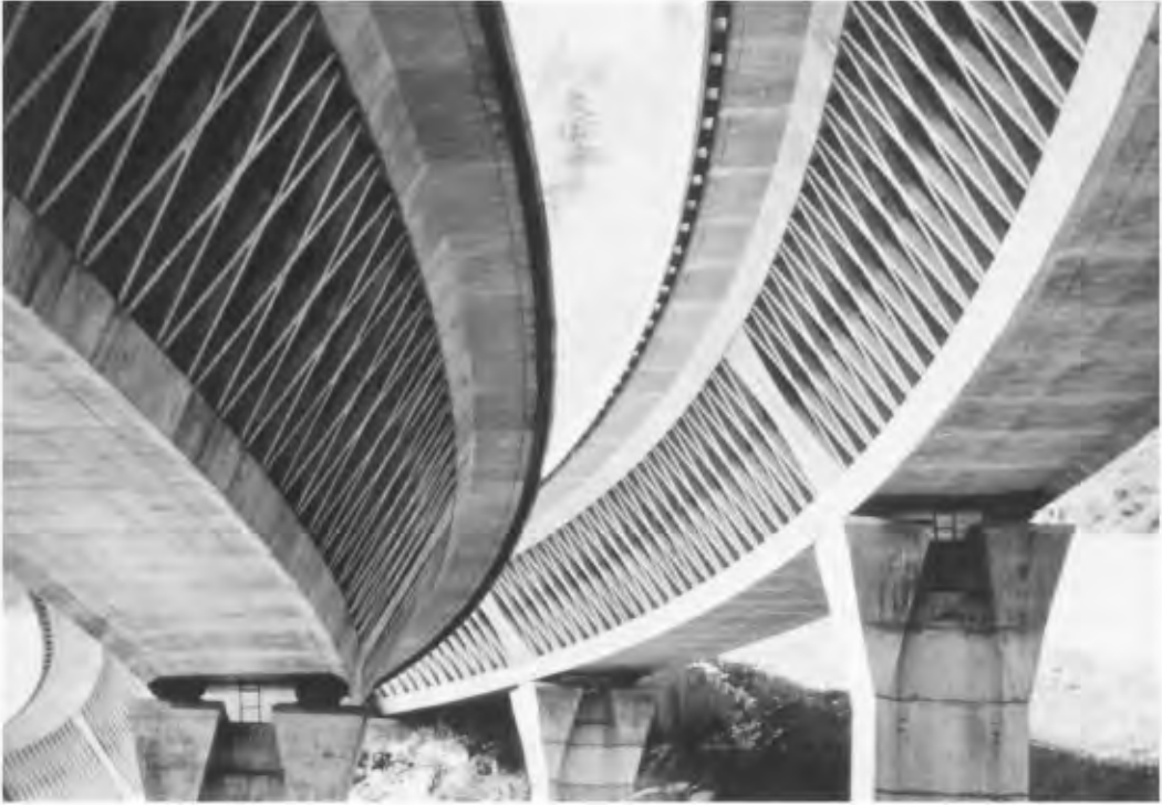
FIGURE 64.18 Sylans Bridge — two parallel decks. (Courtesy of Bouygues.)
