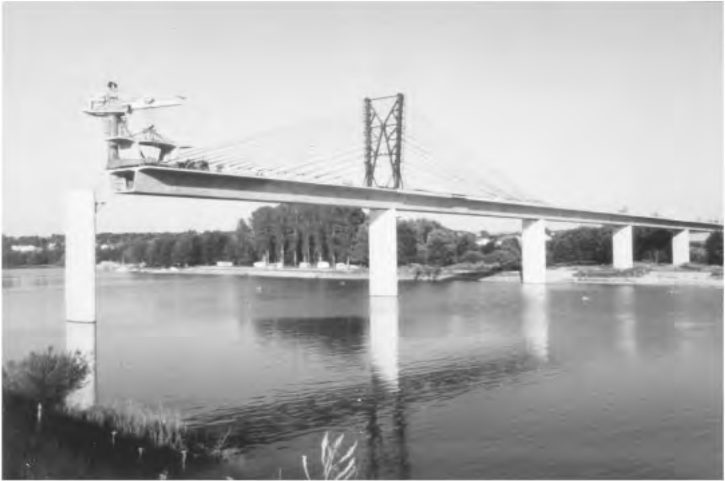
FIGURE 64.13 Fontenoy Bridge. (Courtesy of Campenon Bernard.)
