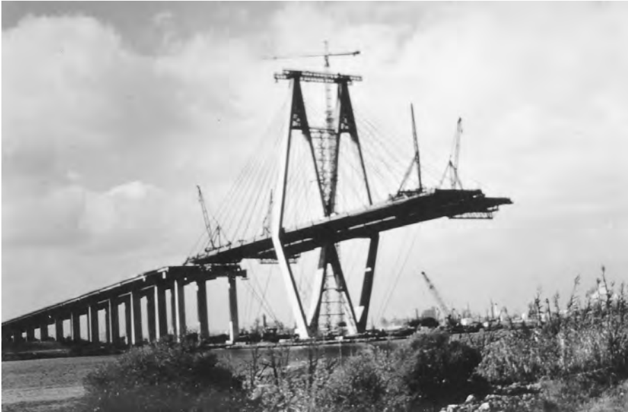
FIGURE 28.10 Baytown Bridge, Texas. (Courtesy of T. Y. Lin International.)
