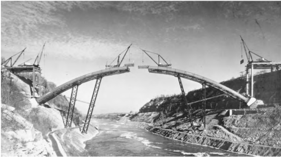
Figure 45.4 Lewiston-Queenston arch bridge, near Niagara Falls, New York, 1962. The longest fixed-arch span in the U.S. at 1000 ft (305 m); rise is 159 ft (48 m). Box arch-rib sections are typically about 3 \times 13\text{-}1/2 ft ( 0.9 \times 4.1 m) in cross-section and about 44\text{-}1/2 ft (13.6 m) long. Job was estimated using erection tiebacks (same as shown in Figure 45.3 ), but subsequent studies showed the long, sloping falsework bents to be more economical (even if less secure looking). Much permanent steelwork was used in the falsework bents. Derricks on approaches load steelwork onto material cars that travel up arch ribs. The 115-ton-capacity travelers are shown erecting the last full-length arch-rib sections, leaving only the short, closing crown sections to be erected. Canada is at left, the U.S. at right. (Courtesy of Bethlehem Steel Corporation.)
