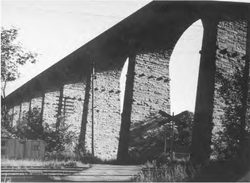
FIGURE 67.8 Starrucca Viaduct, built in the form of the ancient Roman aqueducts, was designed by James Kirkwood for the New York and Erie Rail Road in 1848. It is located over the Starrucca Creek plain at Lanesboro, Pennsylvania. This was the first bridge to use a concrete foundation. This bridge is still in service. (Courtesy of American Society of Civil Engineers.)
