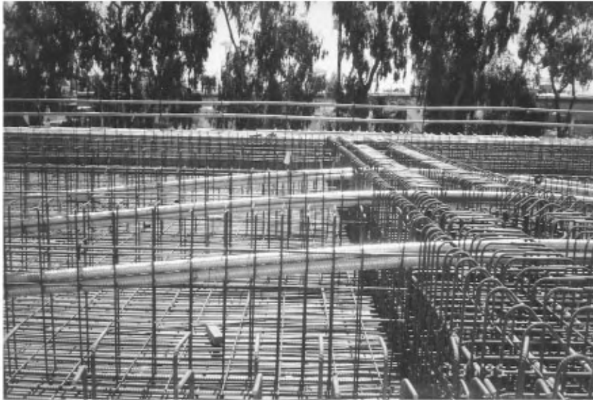
FIGURE 48.6 Bridge soffit and girder reinforcements with prestressing duct profile.
