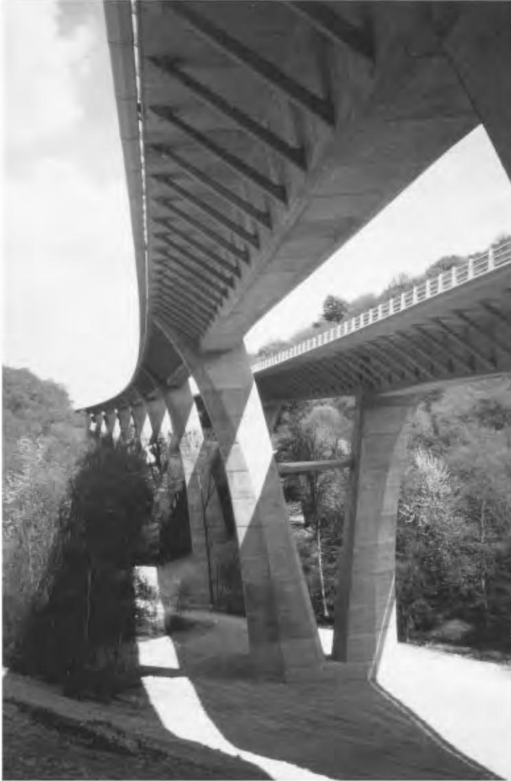
FIGURE 64.39 Rogerville Viaduct. (Courtesy of Jean Muller International.)
