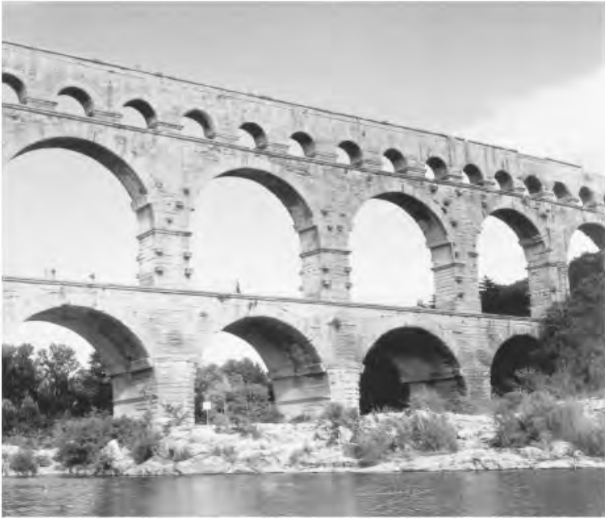
FIGURE 64.1 Gard Bridge over the River Gardon. (Source: Leonhardt, F, Ponts/Puentes — 1986 Presses Polytechniques Romandes. With permission.)
