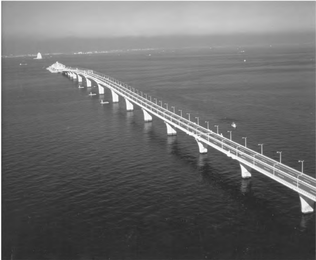
FIGURE 65.46 Steel bridges on Tokyo Wan Aqua-Line. (Courtesy of Trans-Tokyo Bay Highway Corporation.)
