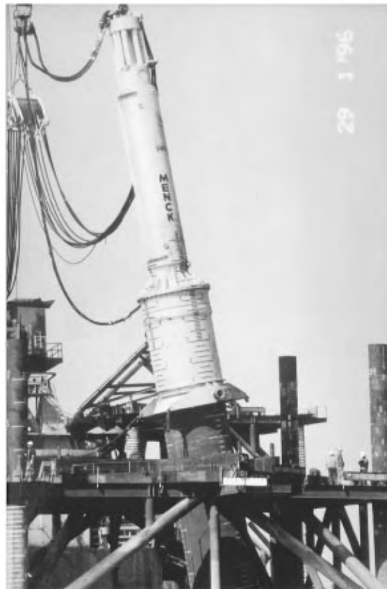
FIGURE 47.2 Driving large-diameter steel tubular pile.
