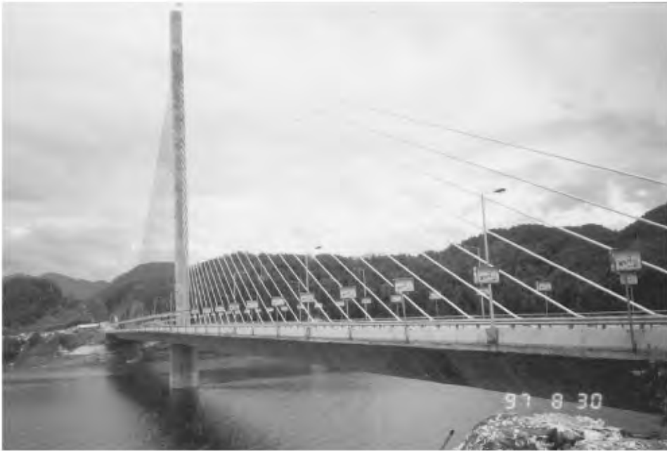
FIGURE 63.27 Huangshan Taiping Lake Bridge.
