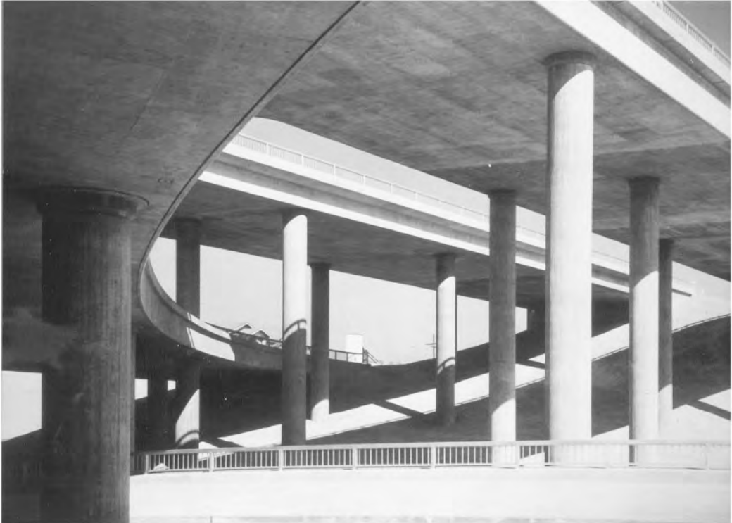
FIGURE 67.39 The Four Level Interchange in downtown Los Angeles, built in 1950, is the first multilevel interchange of two freeways. It is a reinforced concrete box girder, a type developed by, and to become the hallmark of, the California Division of Highways. (Courtesy of California Department of Transportation.)
