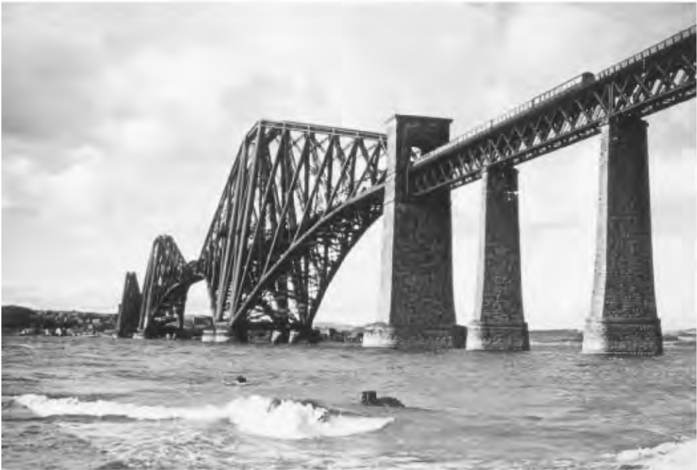
FIGURE 64.2 Firth of Forth Bridge. (Courtesy of J. Arthur Dixon.)
