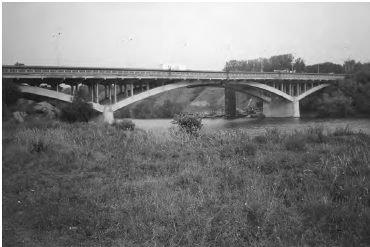
FIGURE 66.35 Moscow Moskva River arch bridge.
