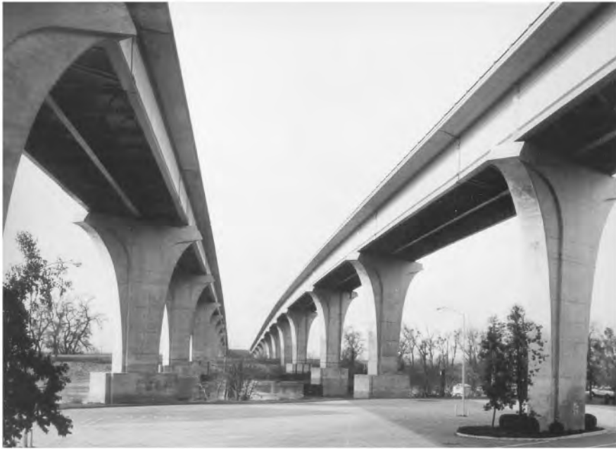
FIGURE 67.46 The Sacramento River Bridge at Elkhorn is a steel girder utilizing high-strength steel. Built in 1970 for Interstate Route 5, the bridge earned an AISC award that year. It was designed by Bert Bezzone of the California Division of Highways. (Courtesy of California Department of Transportation.)
