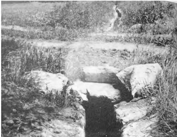
FIGURE 67.1 The aqueduct bridge at La Purisima Mission, Santa Barbara County, California, is an example of a primitive bridge, a short-span stone slab. Built in 1813, it is the oldest bridge in California. (Courtesy of California Department of Transportation.)
