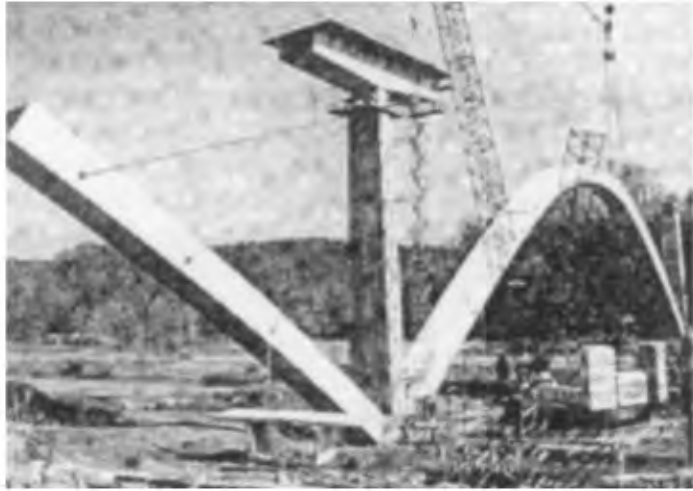
FIGURE 11.18 Natches truss arch—cantilever erection of ribs.
