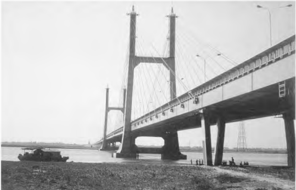
FIGURE 63.24 Dongying Yellow River Bridge.
