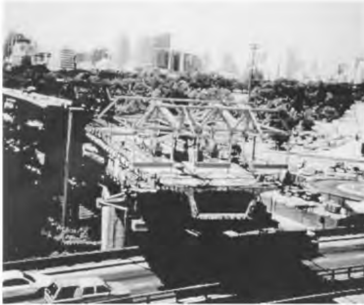
FIGURE 11.3 Construction of the Bangkok Transit System over Rama IV Flyover, Thailand.
