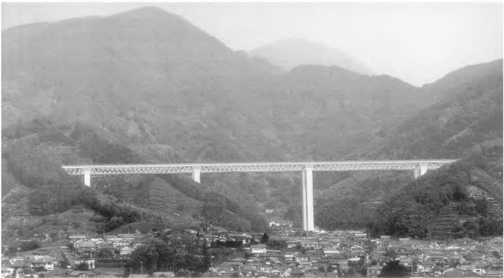
FIGURE 65.28 Tomoegawa Bridge. (Courtesy of Japan Highway Public Corporation.)
