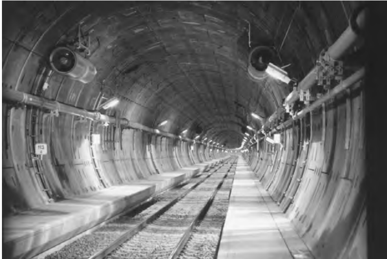
FIGURE 4.6 Storebælt East Tunnel.
