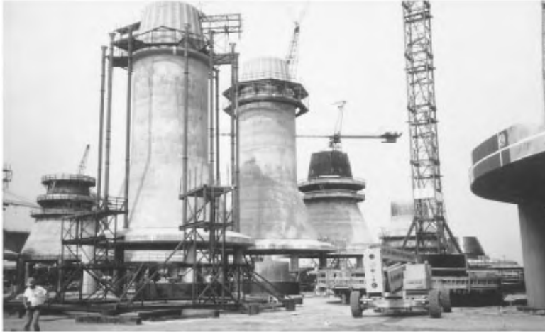
FIGURE 47.25 Prefabrication of pier bases, Prince Edward Island Bridge, Canada.
