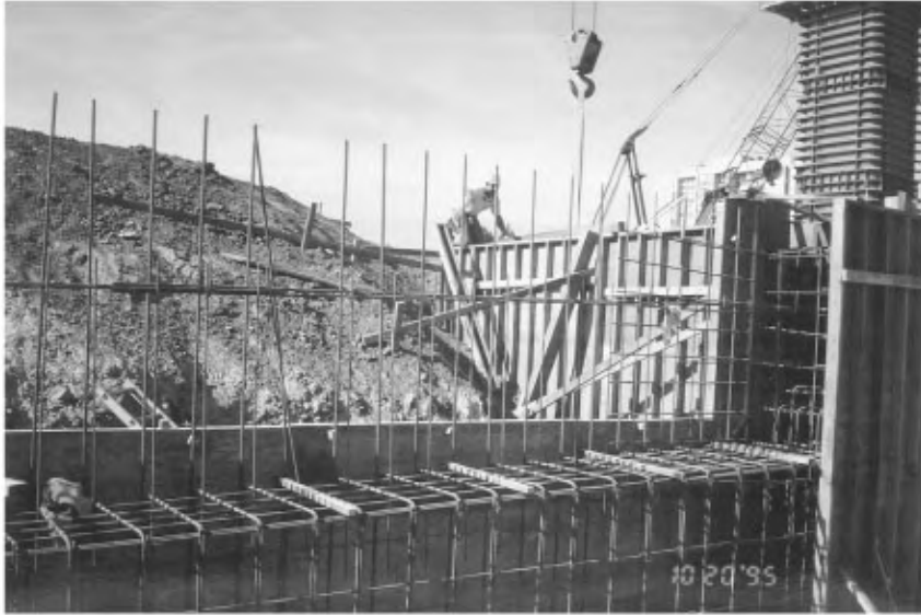
FIGURE 48.3 Wingwall and abutment construction.
