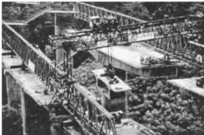
FIGURE 11.51 H-3 Windward Viaduct, Hawaii.
