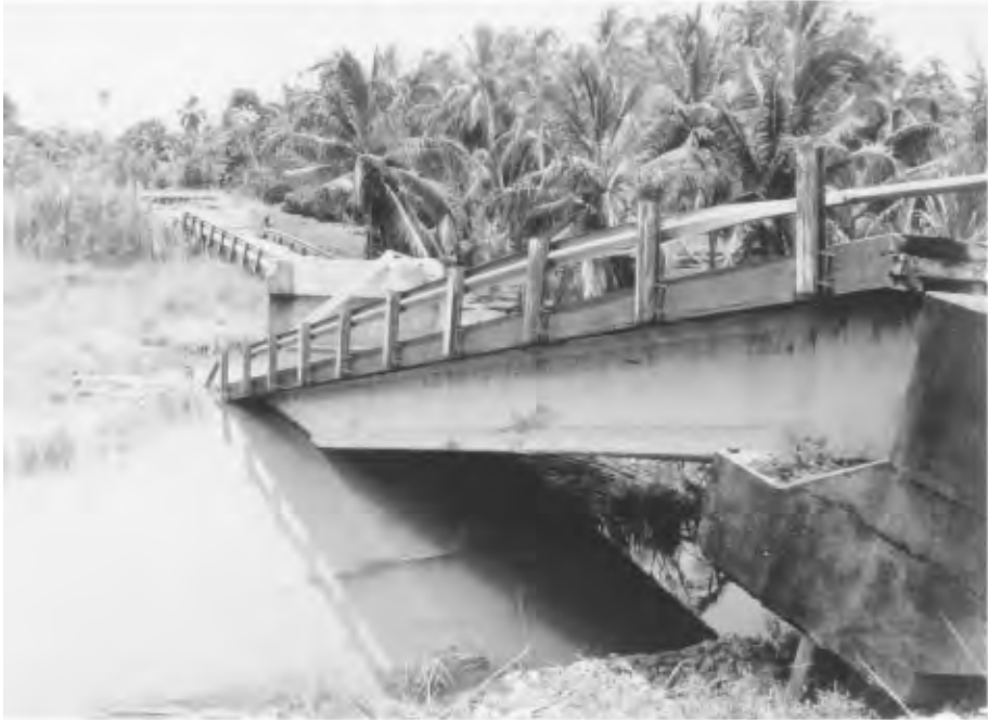
FIGURE 34.9 Rio Bananito Bridge collapse in the 1991 Costa Rica earthquake. (Source: EERI, Earthquake Spectra , Special Suppl. to Vol. 7, 1991.)
