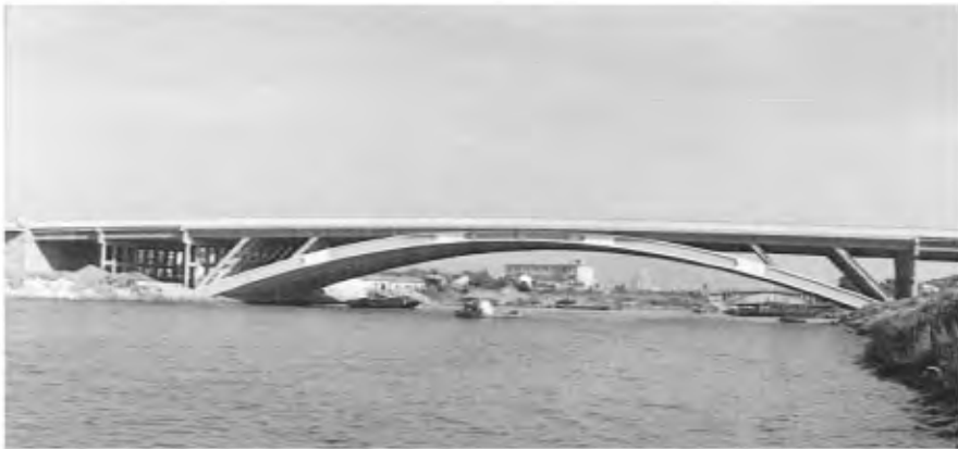
FIGURE 63.12 Jinkui Grand Canal Bridge.
