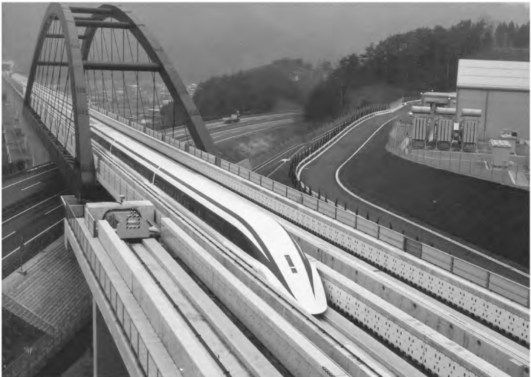
FIGURE 65.50 Maglev car and Ogatayama Bridge. (Courtesy of Japan Railway Corporation.)
