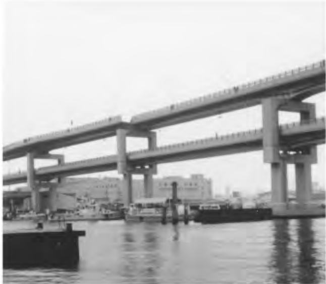
FIGURE 34.15 Hamate Bypass superstructure rotations as a result of bearing failures in the 1995 Hyogo-Ken Nanbu earthquake.
