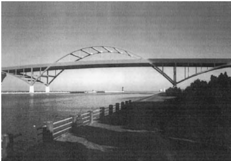
FIGURE 17.8 Milwaukee Harbor half-through arch.
