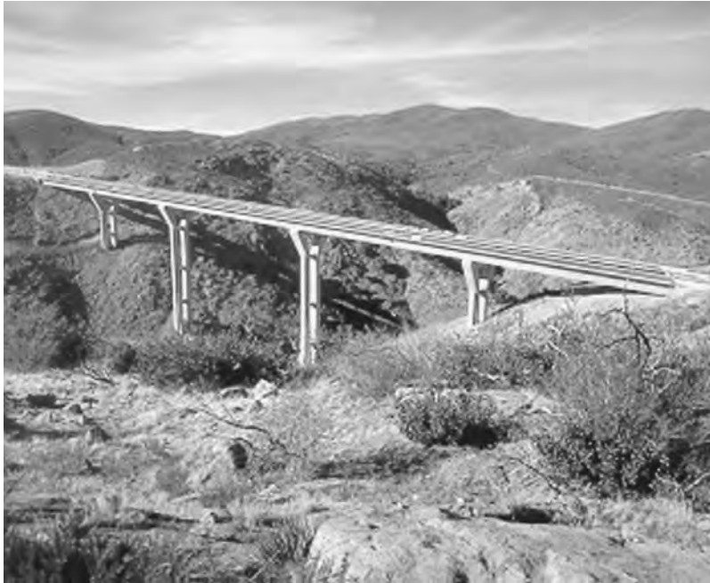
FIGURE 46.5 Pine Valley Creek Bridge — construction completion.
