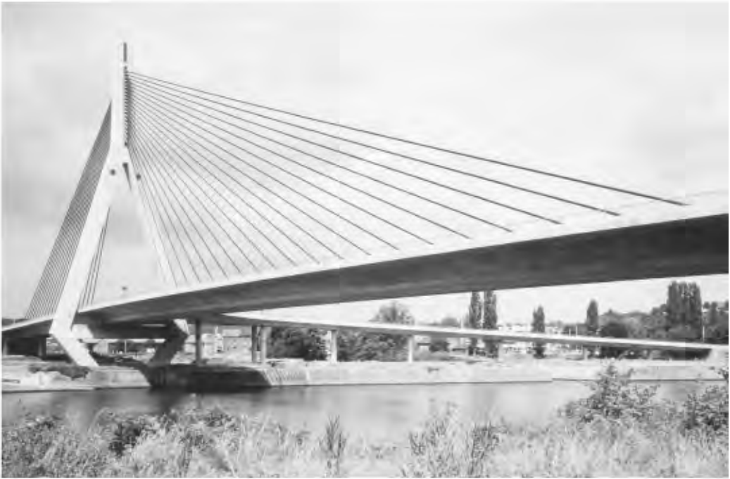
FIGURE 64.16 Ben Ahin Bridge. (Courtesy of Daylight for Greisch.)
