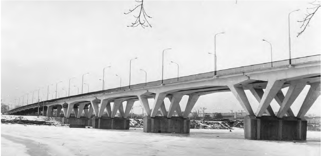
FIGURE 66.32 Penza Sura River Bridge.
