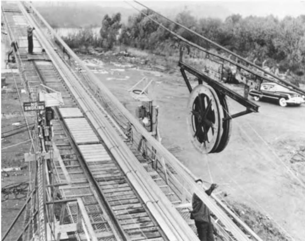
Figure 45.25a Tramway starts across from east anchorage carrying two wire loops. Three 460-wire strands have been spun, with two more under construction. Tramway spinning wheels pull wire loops across the three spans from east anchorage to west anchorage. Suspended footbridges provide access to cables. Spinning goes on 24 hours per day.
