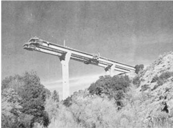
FIGURE 46.2 Pine Valley Creek Bridge — construction at Pier 4.
