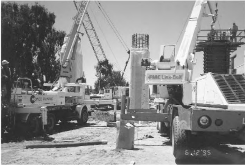
FIGURE 48.2 Crane used to hold the column cage; column is being cured with plastic wrap.
