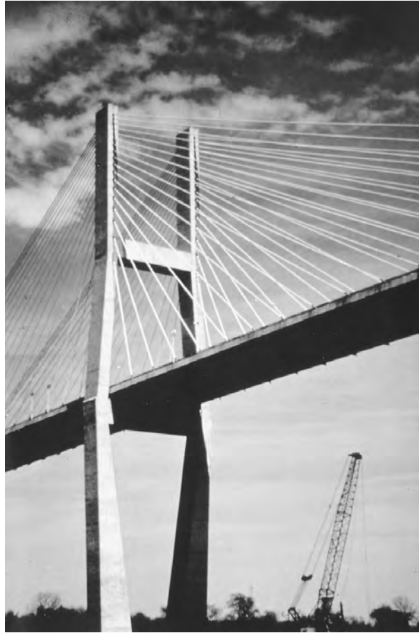
FIGURE 28.8 Talmadge Bridge, Georgia. (Courtesy of T. Y. Lin International.)
