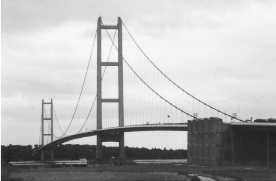
FIGURE 28.12 Humber Bridge, England. (Courtesy of Charles Seim.)
