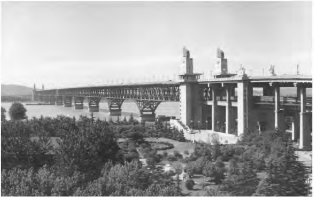
FIGURE 63.21 Nanjing Yangtze River Bridge.
