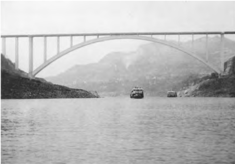
FIGURE 63.14 Wanxian Yangtze River Bridge.
