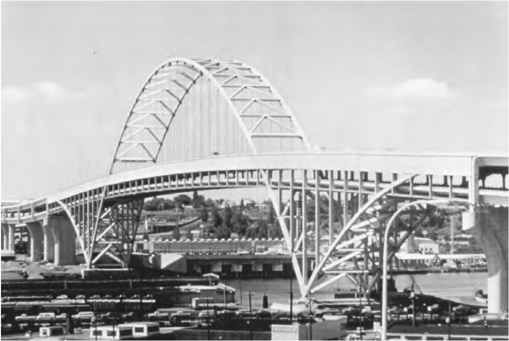
FIGURE 17.9 Fremont Bridge across the Willamette River.
