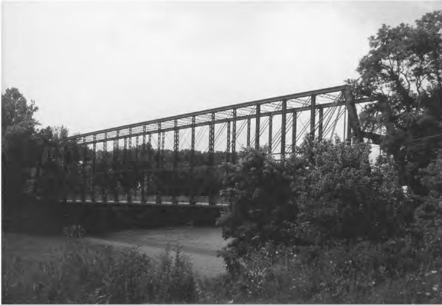
FIGURE 67.15 Laughery Creek Bridge, near Aurora, Indiana, was built by the Wrought Iron Bridge Company of Canton, Ohio, in 1878. Its 92-m span was unprecedented. This bridge appeared on the cover of the company’s catalog in 1893. (Courtesy of American Society of Civil Engineers.)
