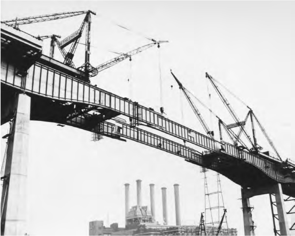
Figure 45.29 Erecting closing girder sections of Passaic River Bridge, New Jersey Turnpike, 1951. Huge double-boom travelers, each weighing 270 tons, erect closing plate girders of the 375 ft (114 m) main span. The closing girders are 14 ft (4.3 m) deep and 115 ft (35 m) long and weigh 146 tons each. Sidewise entry was required (as shown) because of long projecting splice material. Longitudinal motion was provided at one pier, where girders were jacked to effect closure. Closing girders were laterally stable without floor steel fill-in, such that derrick falls could be released immediately. (Courtesy of Bethlehem Steel Corporation.)
