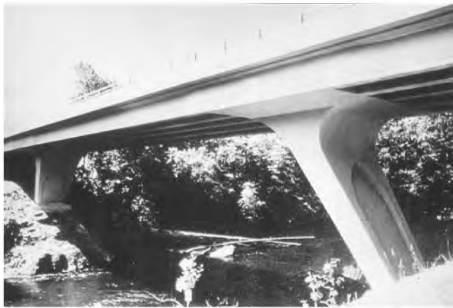
FIGURE 67.29 The North Santiam (Gates) Bridge, in Marion County, Oregon, earned a Portland Cement Association design award in 1997. It was designed by the Oregon Department of Transportation. (Courtesy of Portland Cement Association.)
