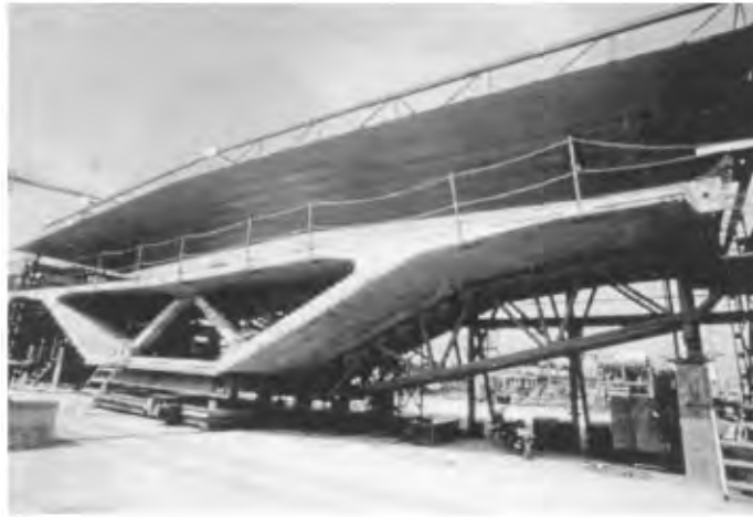
FIGURE 11.54 Bang Na Expressway, Thailand — D6, six-traffic-lane segment at precast yard.
