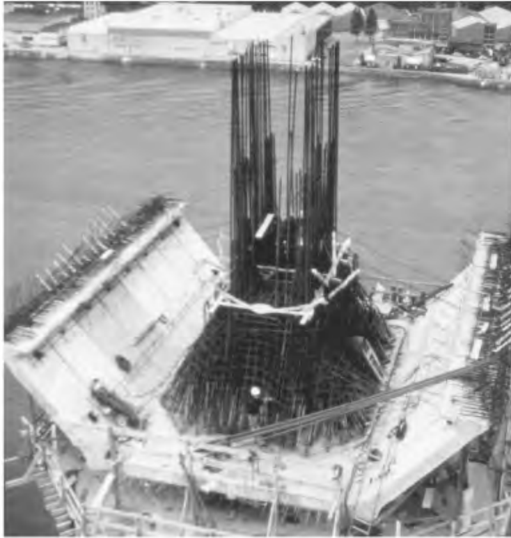
FIGURE 64.30 Brotonne Bridge — pylon base reinforcement. (Courtesy of Campenon Bernard.)
