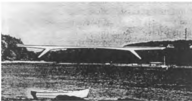
FIGURE 11.19 Bonhomme Bridge in Brittany, France.
