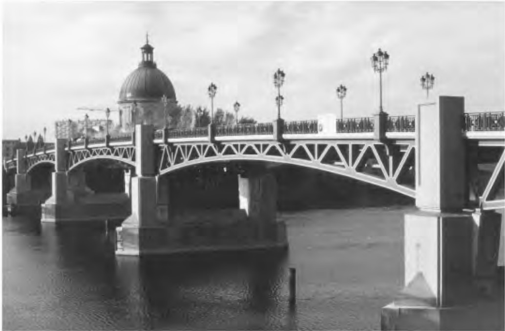
FIGURE 64.11 Saint Pierre Bridge. (Courtesy of Albert Berenguier, Egis Group.)
