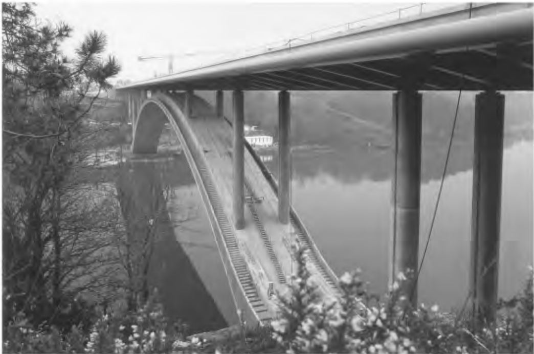
FIGURE 64.23 La Roche Bernard Bridge. (Courtesy of Campenon Bernard.)
