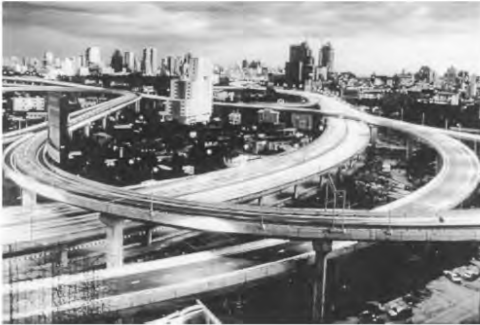
FIGURE 11.56 View of the completed Second Expressway System Project, Thailand.
