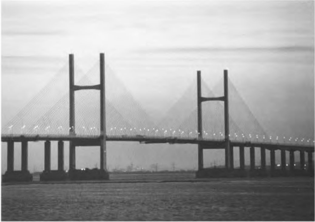
FIGURE 64.33 Second Severn Bridge at twilight time. (Courtesy of G.T.M.)
