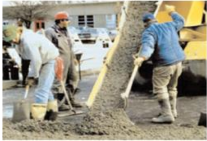
Direct Chute Discharge
