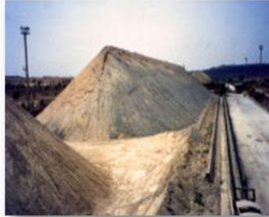
a completed limestone pre-homogenization pile
