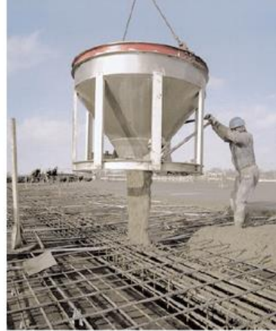
Crane and bucket
