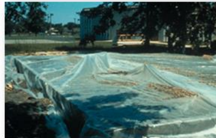
▪ Covering with wet gunny bags or polyethylene
