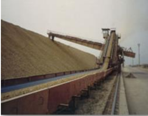
limestone pre-homogenization pile
