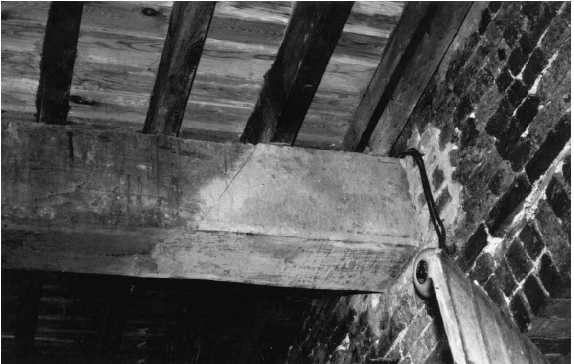
Photograph 8.13 Epoxy resin-based repair to decayed beam end
