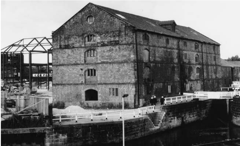
Photograph 10.1 The Granary Building, Leeds: north and east elevations
