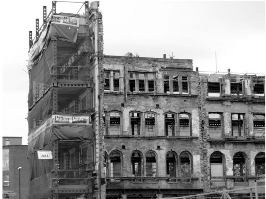
Photograph 13.22 Proprietary external façade support system, Belfast
