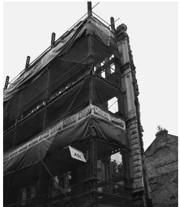
Photograph 13.10 Proprietary façade retention system
