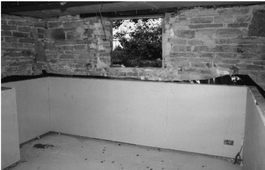
Photograph 6.4 Traditional dense polythene wall-lining with block-work loading wall and thermal-board dry lining. (Note: the untreated section of wall is above ground level)
