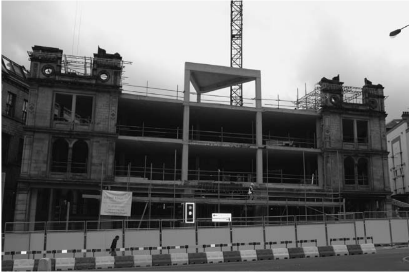
Photograph 13.34 Façade removed brick by brick
