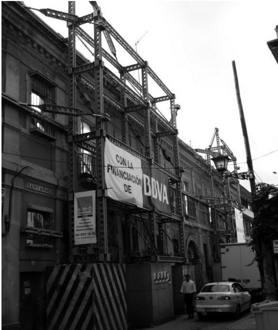
Photograph 13.7 Temporary external façade support – proprietary system
