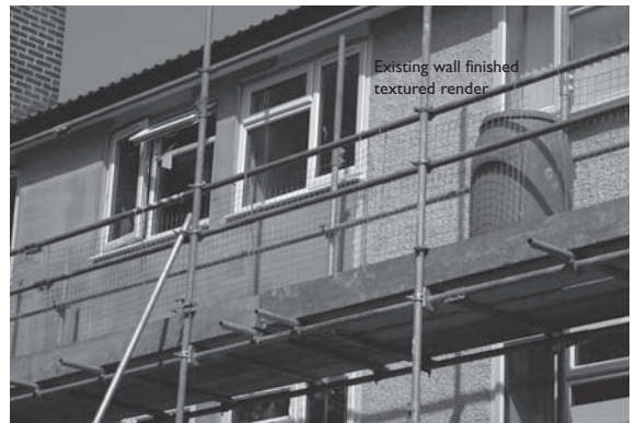
Photograph 4.11 Existing textured render provided a strong substrate with which to bond the insulation
