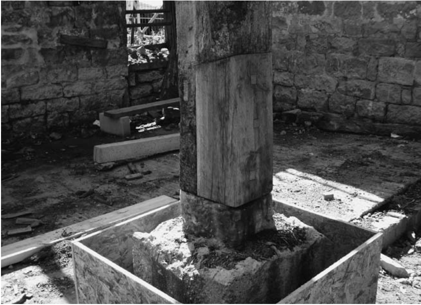
Photograph 8.16 Section of timber cut into existing column and pinned in place
