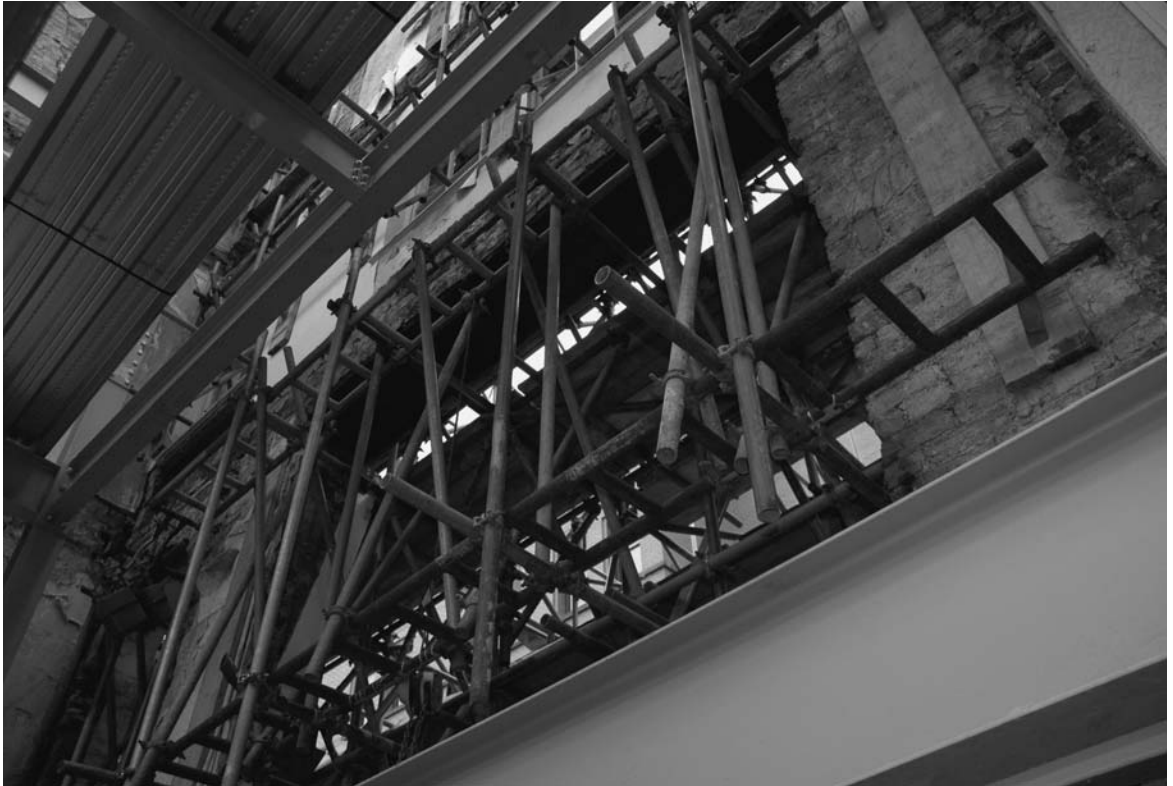
Photograph 13.18 Through-tie and strap using deep steel ladder beams (courtesy of Paul Smith ROK Developments)
