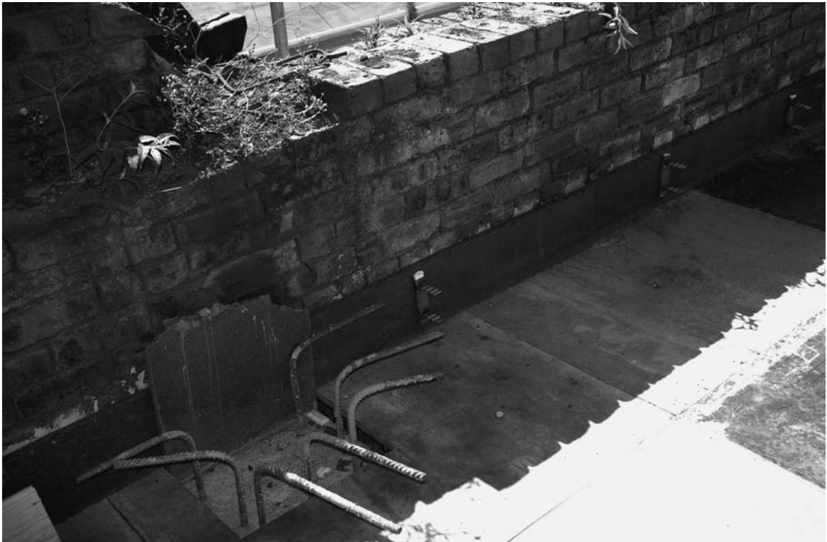
Photograph 13.27 (below) Expansion board and restraint fixings in place prior to concrete floor being cast
