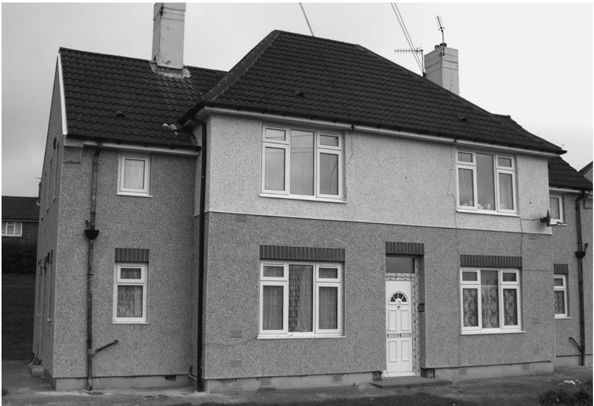
Photograph 4.8 Finished building, fully insulated without major disruption to occupants
