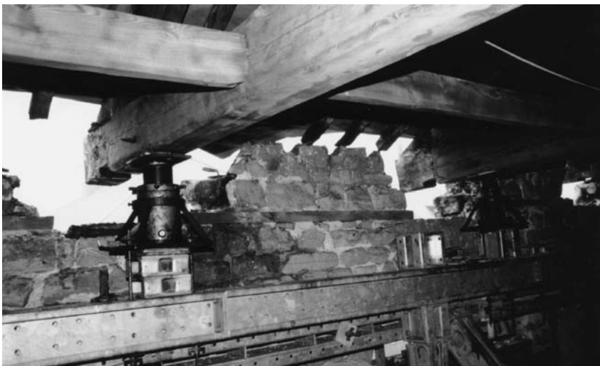
Photograph 10.3 The Granary Building, Leeds: after lifting of roof
