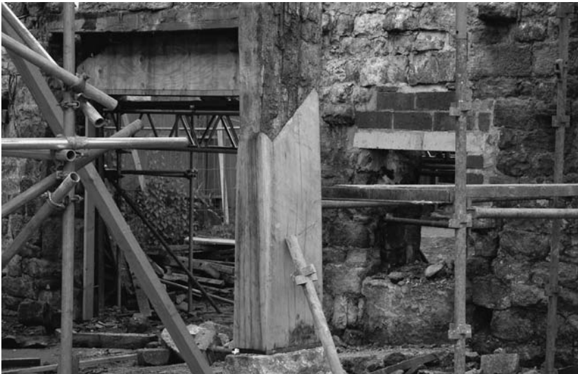
Photograph 8.17 Spliced oak column
