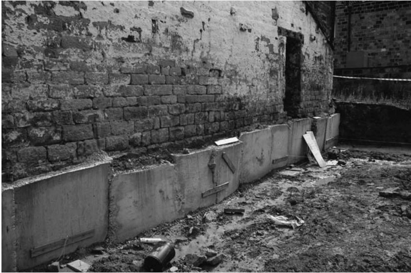
Photograph 11.3 Mass concrete underpinning
