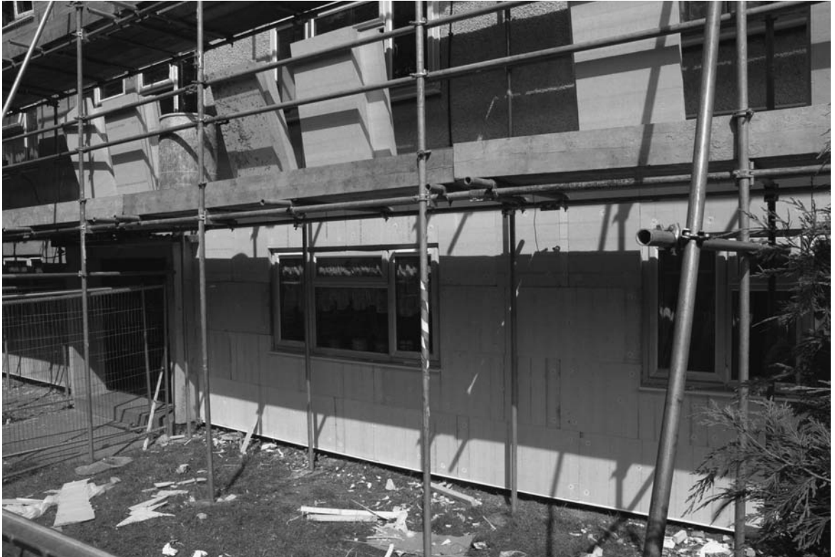
Photograph 4.9 External insulation bonded to existing wall
