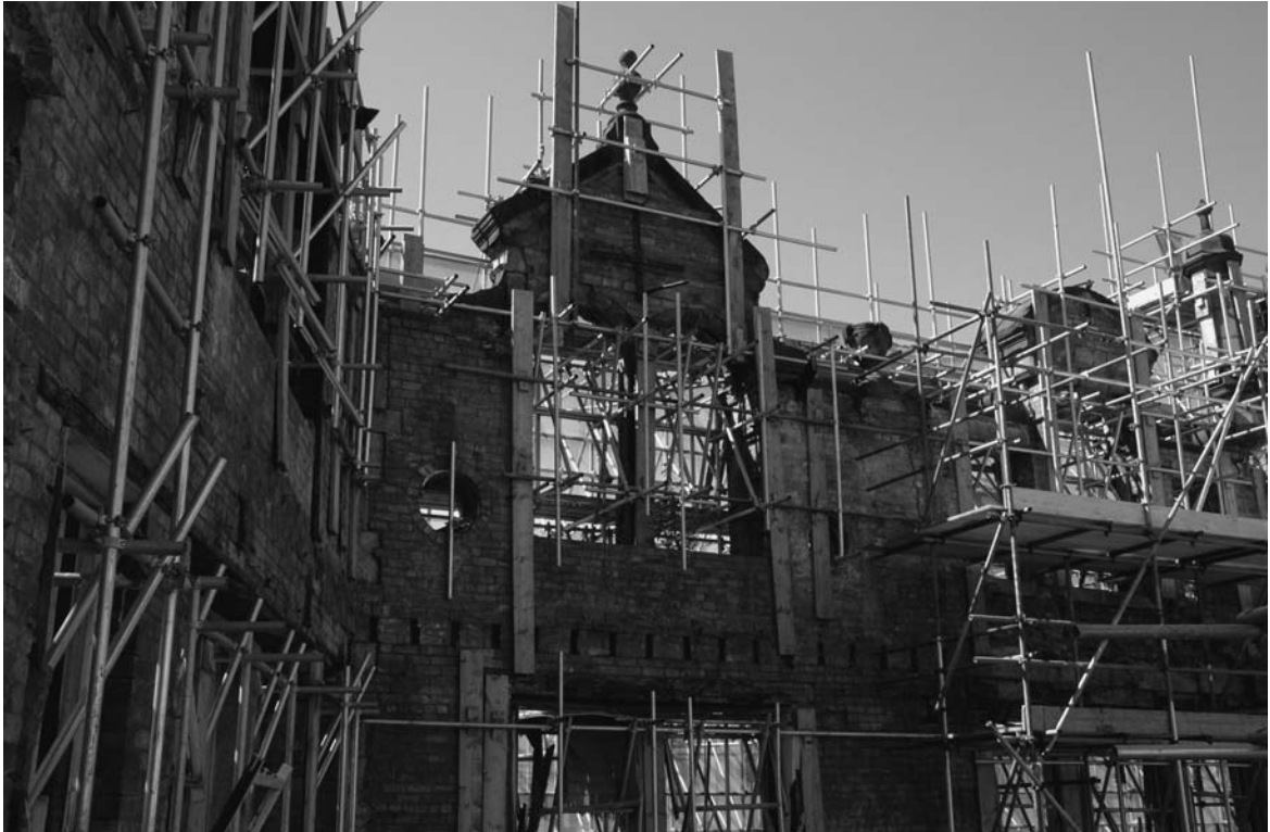
Photograph 13.29 Tubular scaffold system: through-ties and clamps
