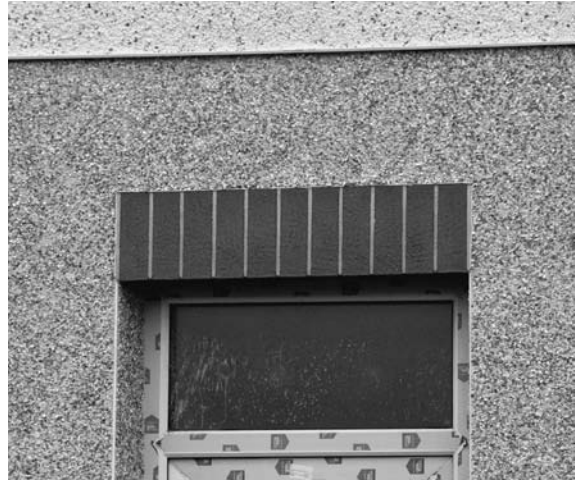
Photograph 4.7 Brick detail formed out of render. It is difficult to recognise the difference between brick render and bricks
