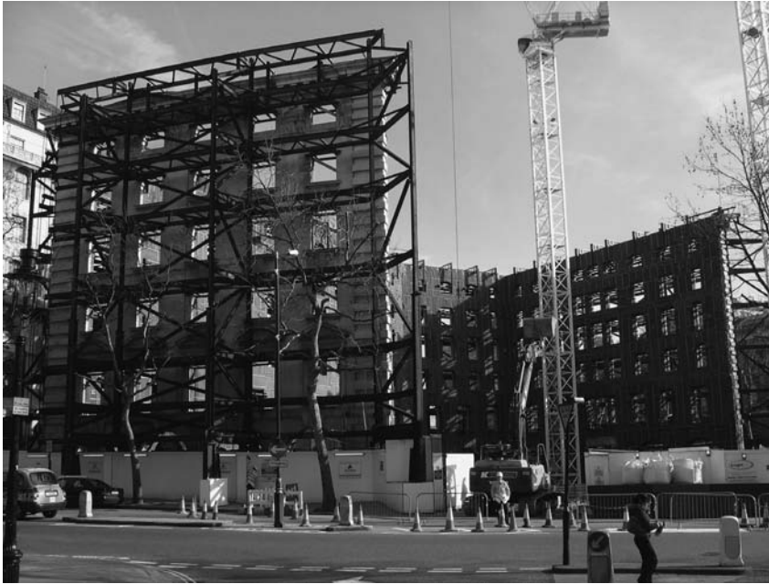
Photograph 13.38 External rolled steel façade retention system
