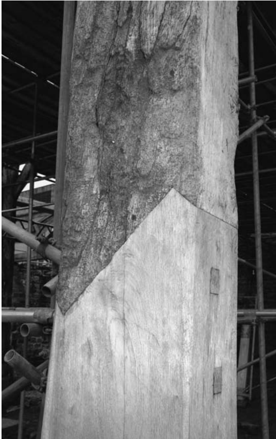
Photograph 8.15 Pinned mortise and tenon joint
