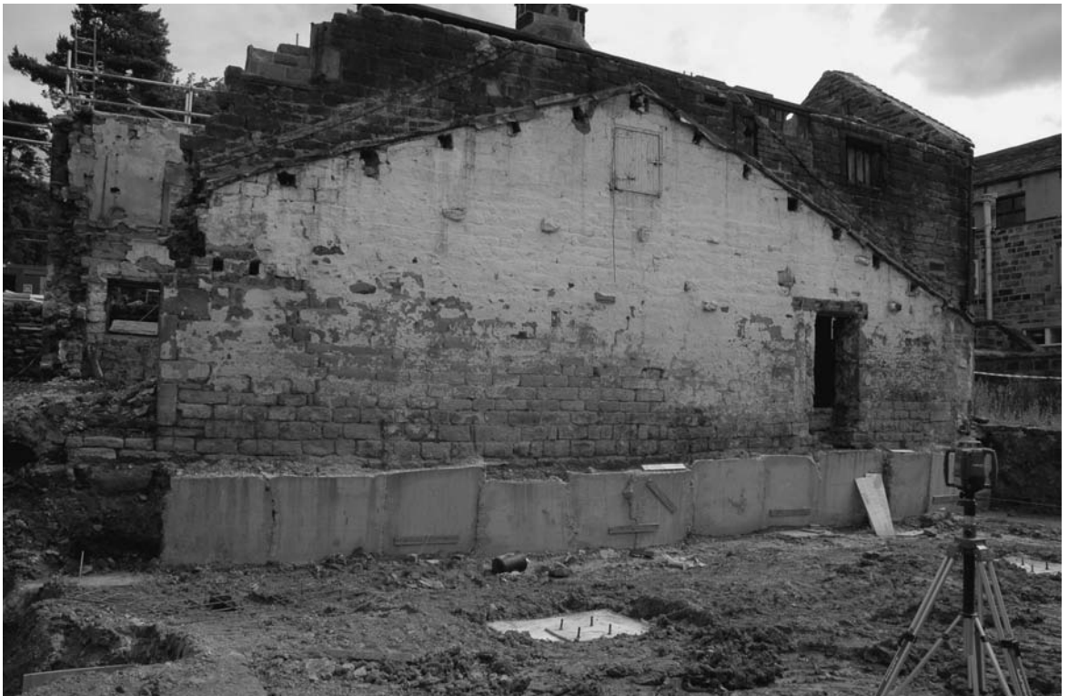
Photograph 11.4 Mass concrete underpinning
