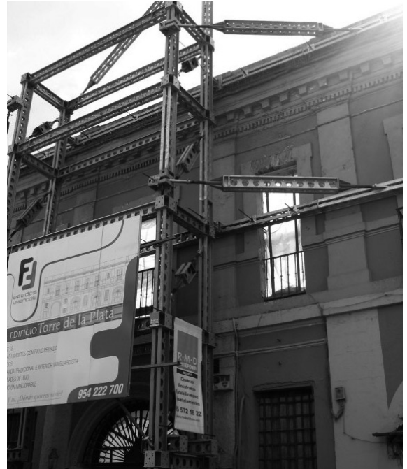
Photograph 13.8 Adjustable façade retention system
