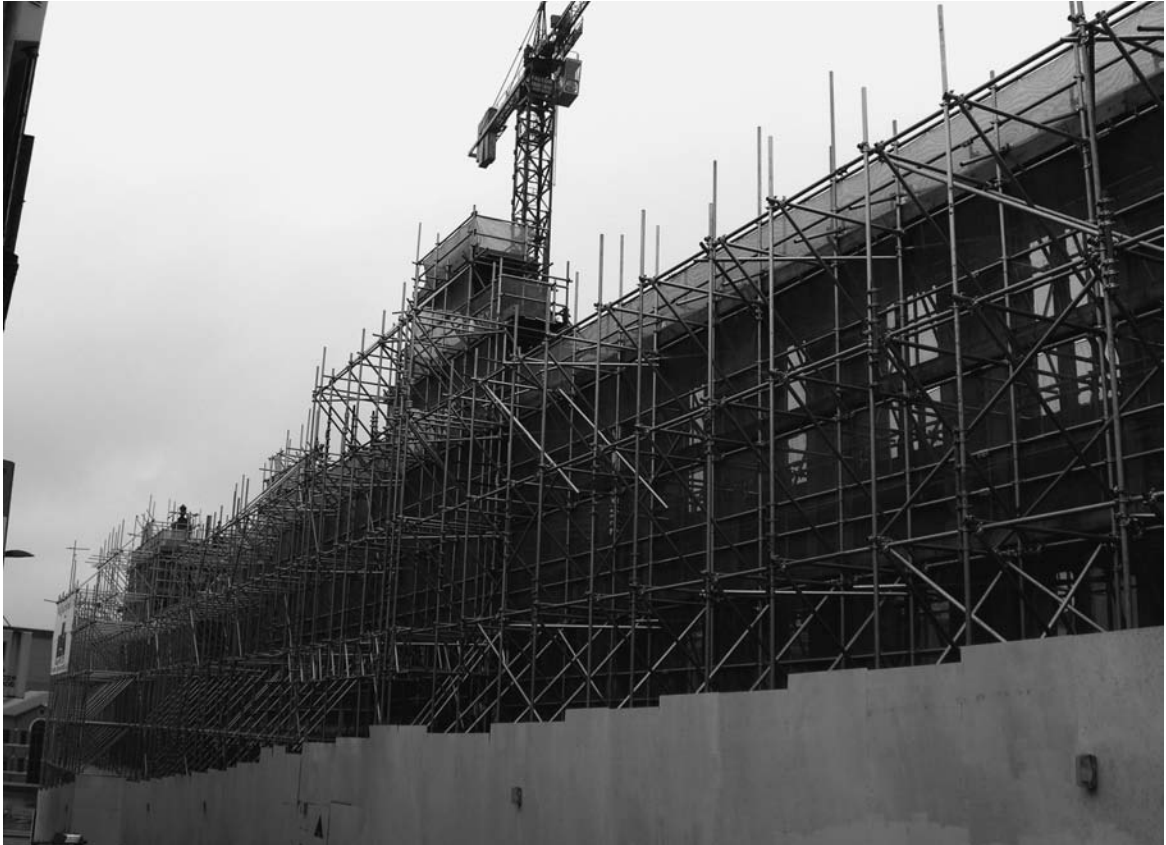
Photograph 13.5 Tubular façade retention scheme, East Brook Hall, Bradford
