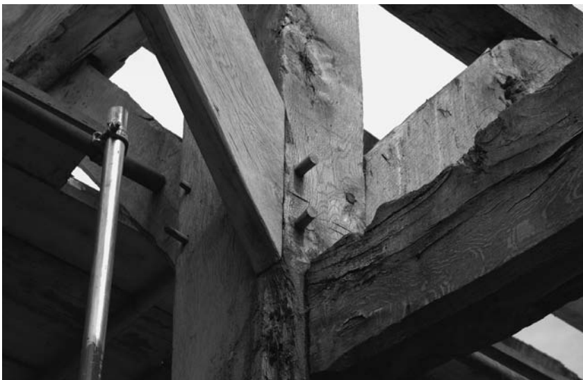
Photograph 8.14 Existing structural timber can be removed and replaced
