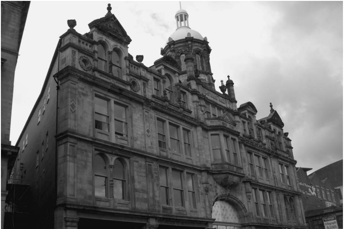
Photograph 13.35 Completed façade after rebuild
