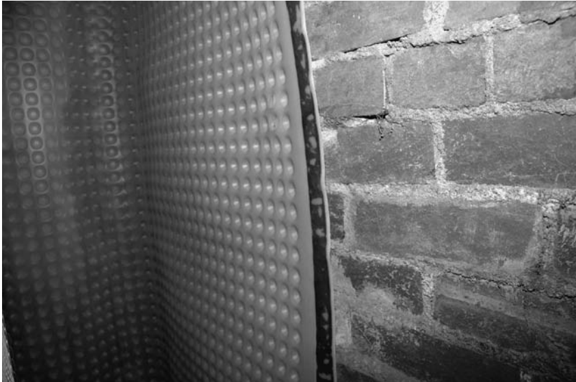
Photograph 6.1 Polypropylene cavity drain ready for fixing to the internal surface of a basement wall
