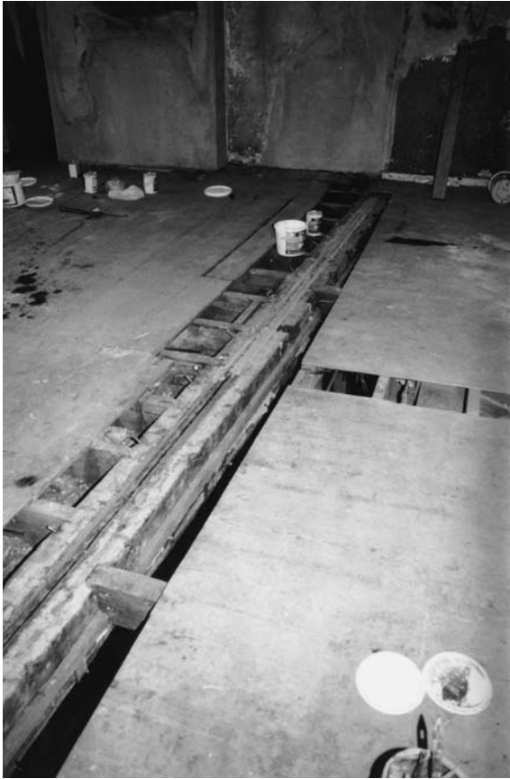
Photograph 9.4 Floor-beam strengthening using steel plate embedded in low-viscosity epoxy
