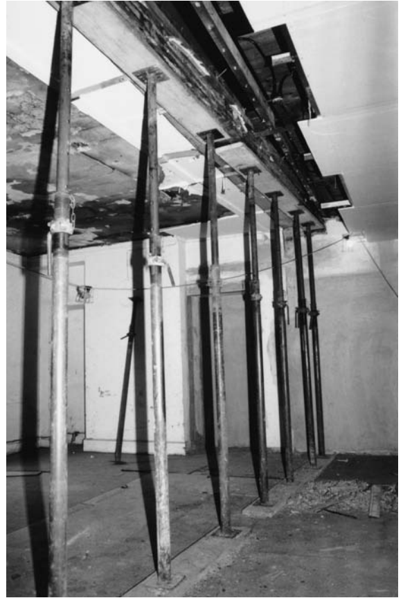
Photograph 9.5 Temporary support to beam during strengthening work
