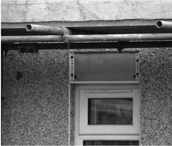
Photograph 4.6 Head of window prepared to provide a render brick finish
