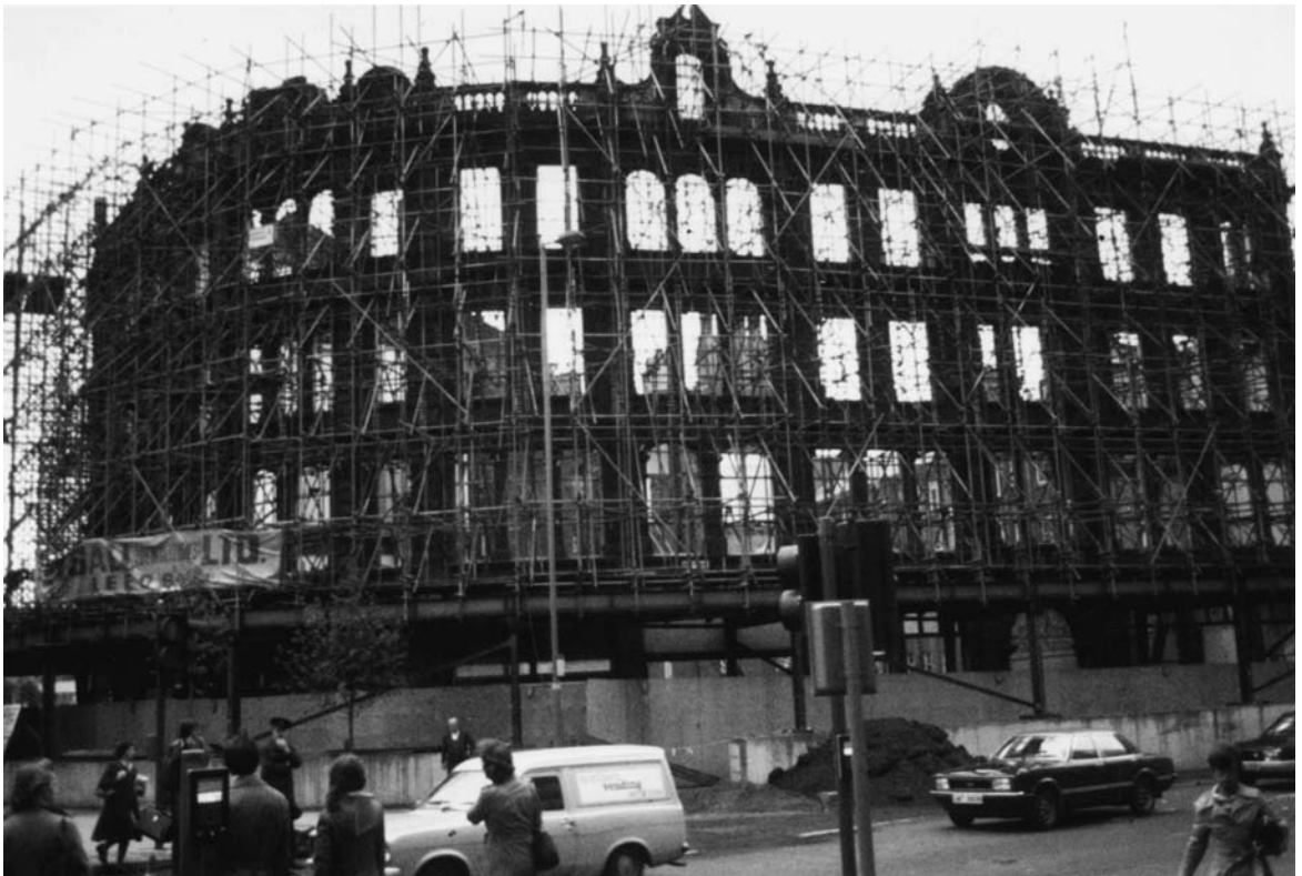
Photograph 13.15 Tubular scaffolding external façade support system, East Parade, Leeds
