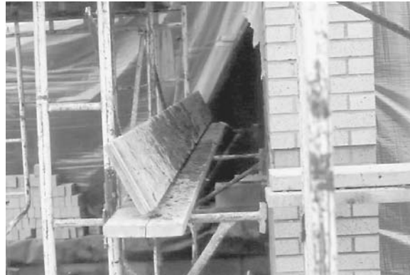
Figure 15-58 Turn scaffold boards on edge at the end of the day to avoid splashing mortar droppings or dirt onto the face of the wall.
