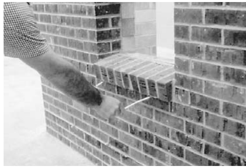
Figure 15-34 Oiled rods, ropes, or pins should be spaced 16 in. on center and removed before final set of mortar. (Photo courtesy BIA.)
