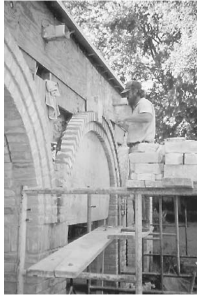
Figure 15-57 Arches require temporary support until the masonry attains strength.
