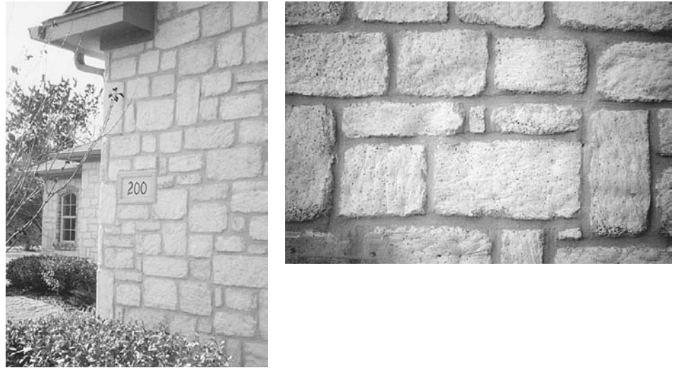
Figure 4-3 Simulated stone made to resemble natural rubble stone is not the same strength and quality as architectural cast stone.
