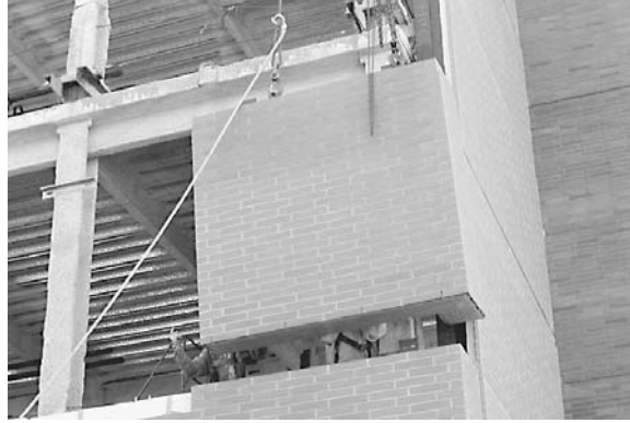
Figure 15-59 Lifting a prefabricated masonry panel into place.
