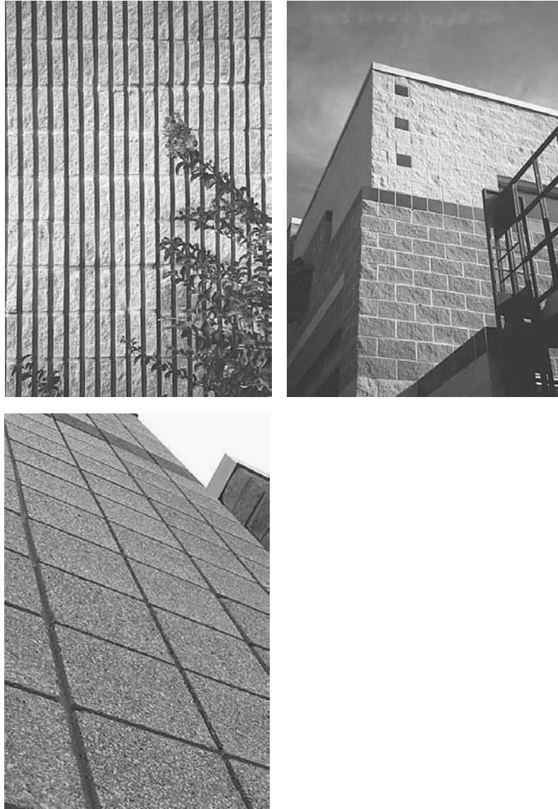
Figure 4-11 Ribbed, split-face, and burnished concrete block.
