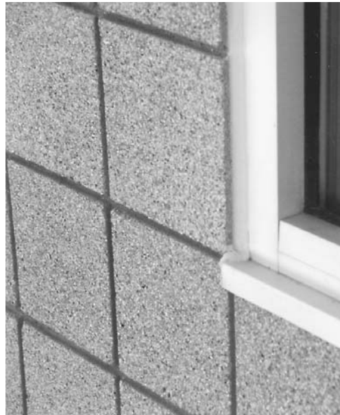
Figure 2-8 Concrete blocks face-ground to expose natural aggregate colors.
