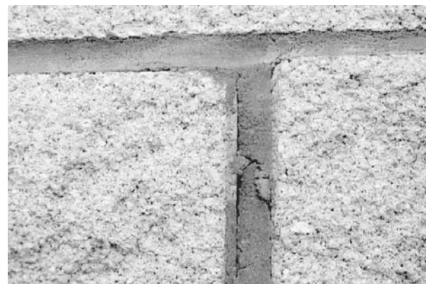
Figure 15-24 Good joint tooling is the first line of defense against water penetration, and is especially critical in single-wythe walls.
