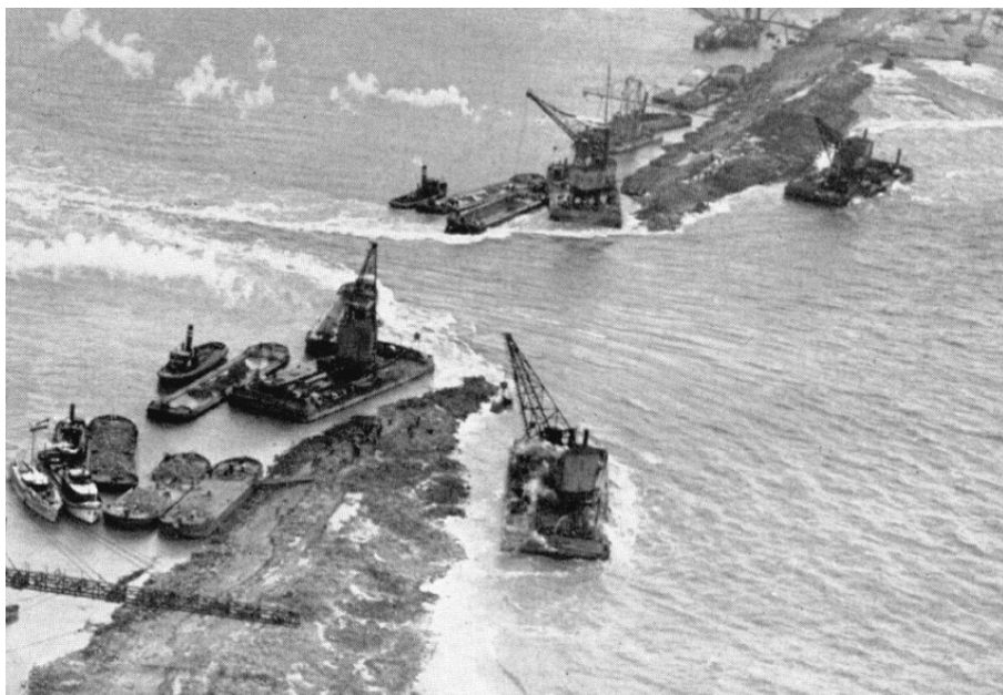
Figure 13-6 Positioning the floating cranes
