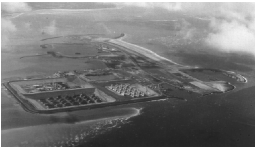
Figure 14-4 Dredged dock for construction of caissons at Neeltje Jans construction island
