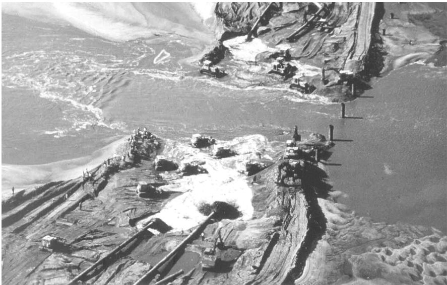
Figure 13-11 Final closure using sand only
