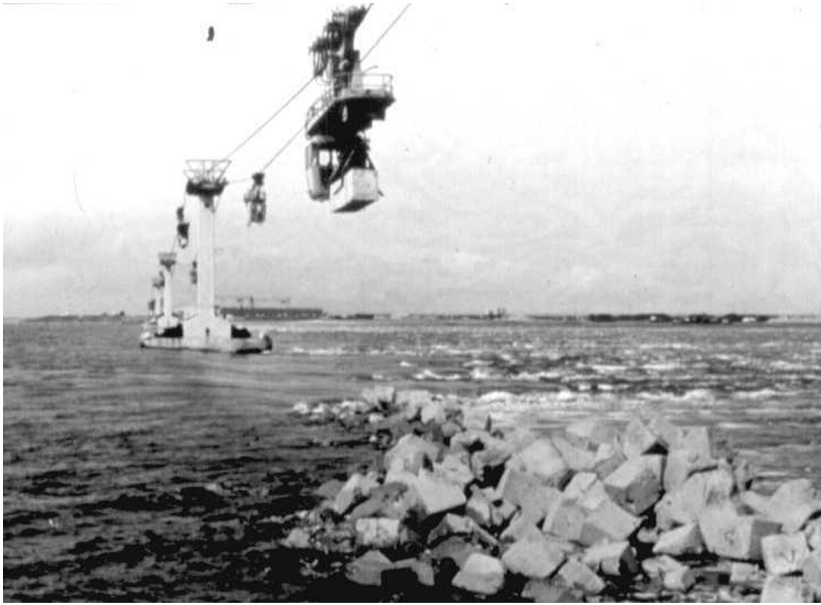
Figure 13-12 Closure with a cable way
