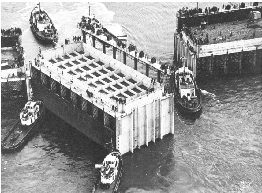
Figure 14-7 Placing the final caisson in “Het Veerse Gat”
