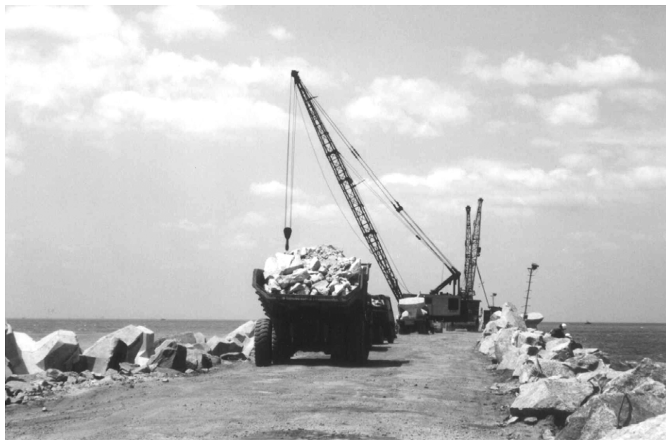
Figure 13-3 A breakwater under construction
