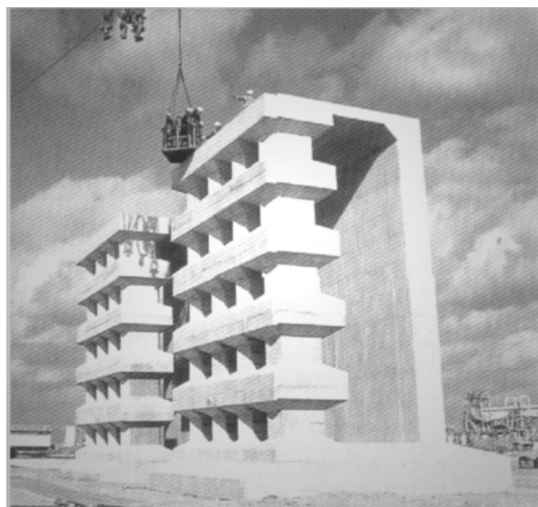
Figure 9-11 Honey wall breakwater
