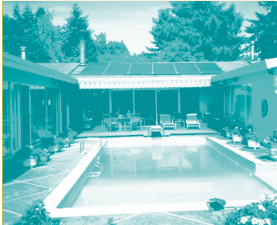
▲ Tsawwassen, British Columbia. This 5-m x 10-m (16-ft. x 32-ft.) in-ground pool has six 4.4-m 2 (4-ft. x 12-ft.) solar collectors. Photo courtesy Taylor Munro Energy Systems.
