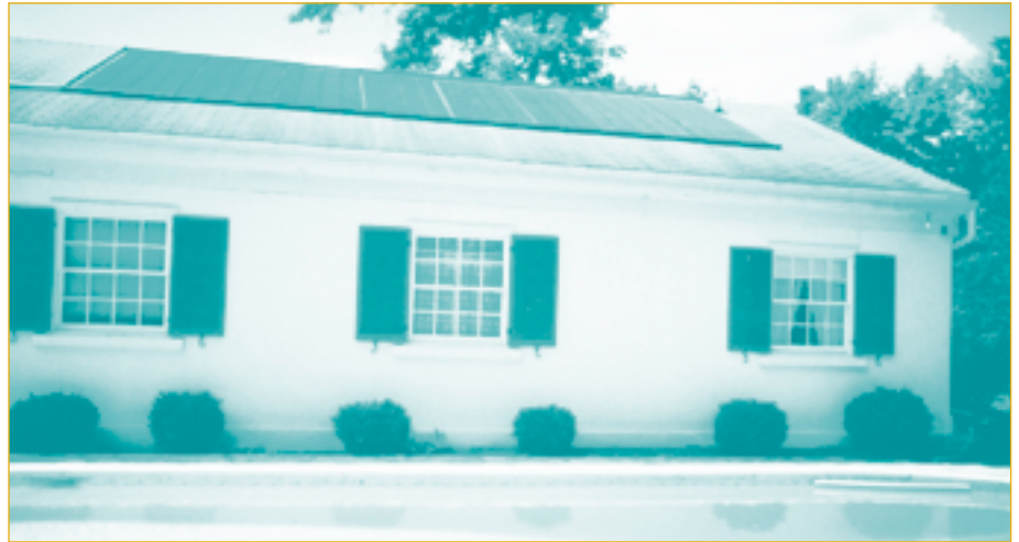
▲ Ottawa, Ontario. 6.1-m x 12.2-m (20-ft. x 40-ft.) in-ground pool, eight 4.4-m 2 (4-ft. x 12-ft.) solar collectors. Photo courtesy of Heliocol Canada.
