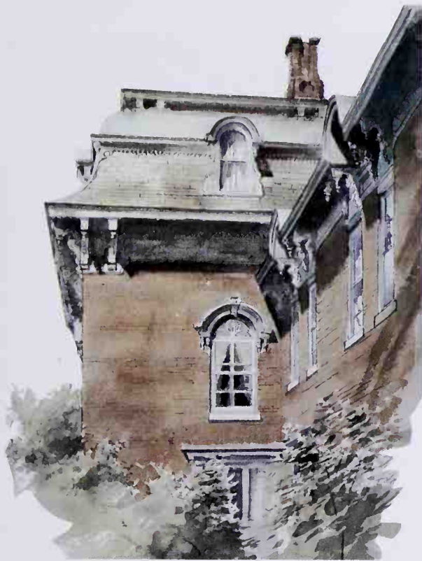
Mansard roof with convex and concave sides, Port Henry, New York
