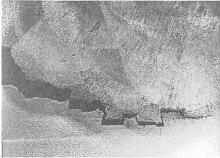
FIG. 4. Typical lamellar tear adjacent to a large fillet weld [39].
