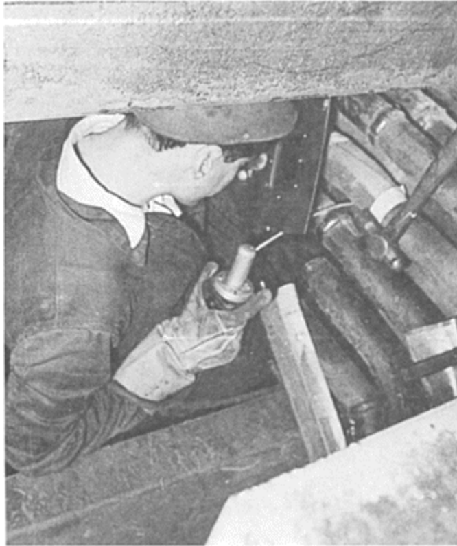
FIG. 7. Illustration of restricted access for welding, typical of the site situation.
