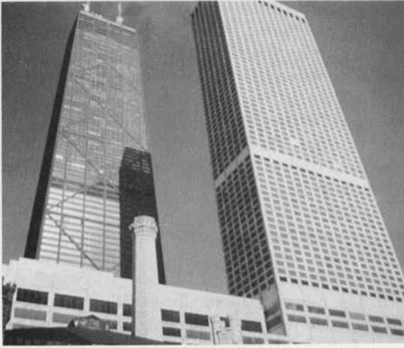
Figure 4.49 The John Hancock Tower in Chicago is an outstanding example of a steel building with exterior braced tube.
