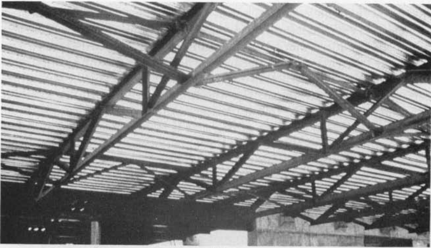
Figure 9.12 (Continued) (d) Photograph of composite truss and metal deck framing.
