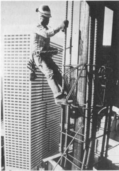
Figure 6.17 (Continued). (e) Reinforcement placement in exterior composite column.
