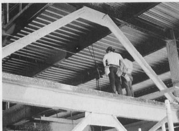
Figure 4.16 Inverted K bracing with double-angle connections.
