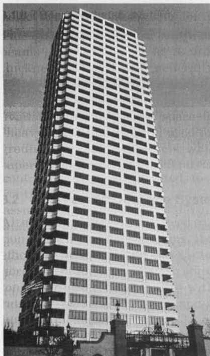
Figure 6.27 The Huntington. (Architects, Talbot Wilson & Associates; structural engineers, Walter P. Moore and Associates; contractor, W. S. Bellows Construction Corp.)
