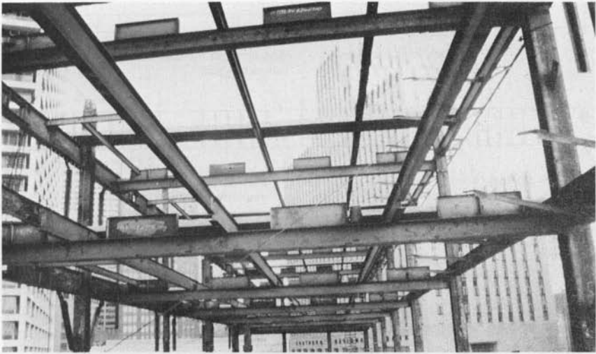
Figure 13 (Continued) (d) Photograph of stub girder framing.
