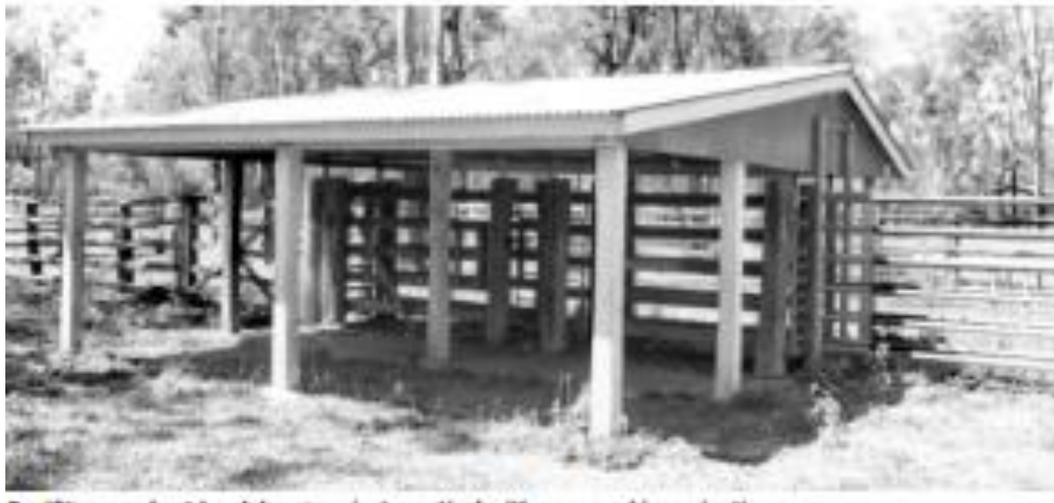
Figure 3. Handling Facilities Covered with roof
