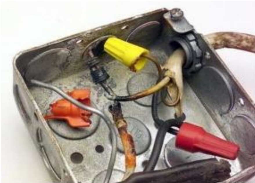
Fig 4.1 heat to burn up the connection wire
