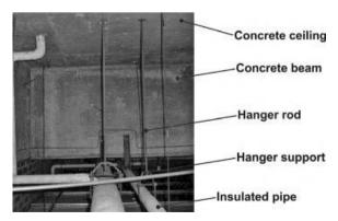
Figure 3.4 Pipes supported on hangers
