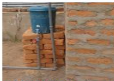
Plate 2: Fertigation chamber and stand
