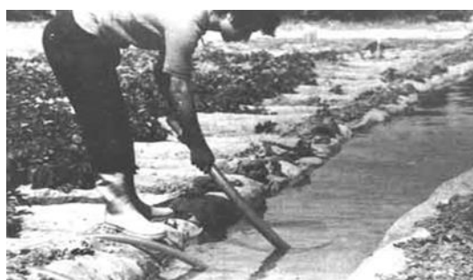
Figure: 1. "Priming" of a siphon
