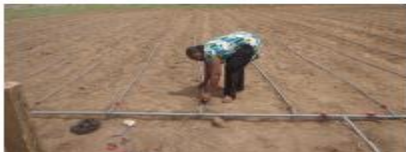
Plate 3: Connecting lateral pipes
