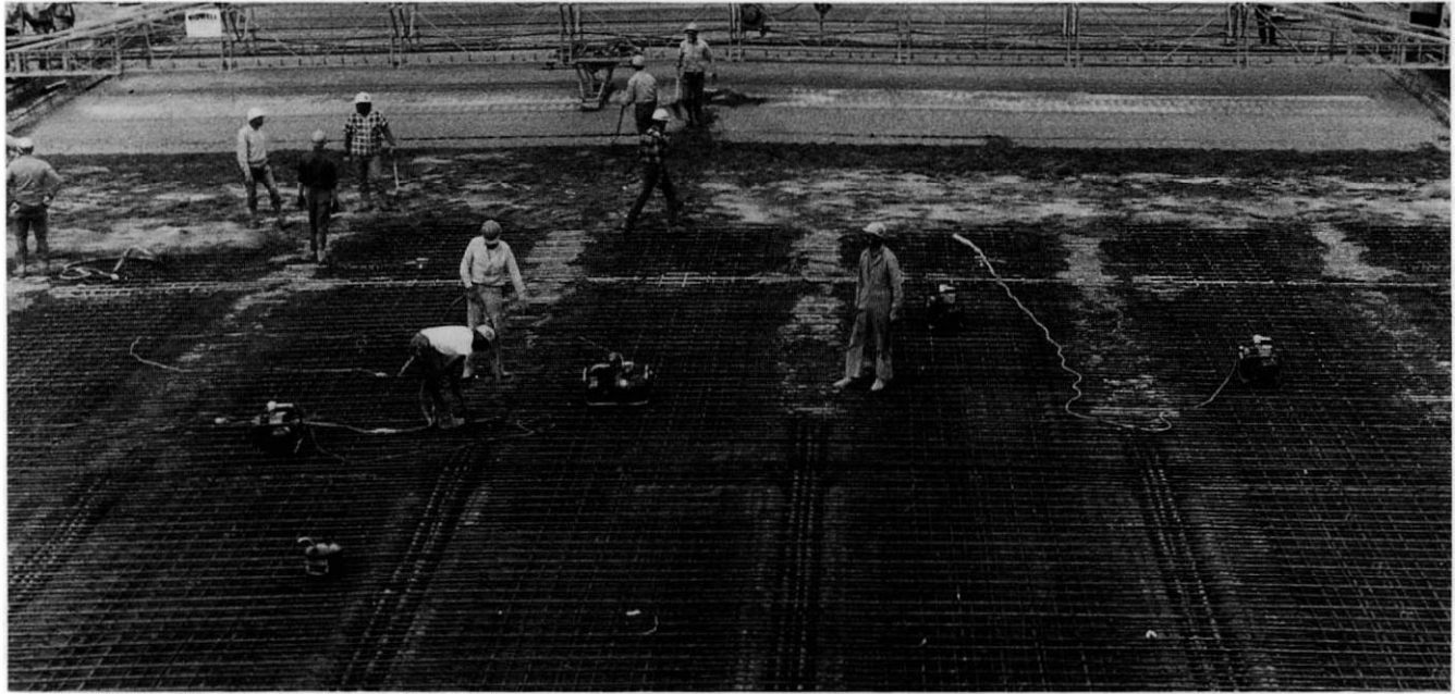
Reinforcing bars in box girder bridge with post-tensioning backs in girders
