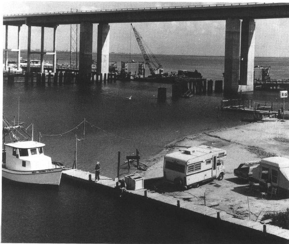
Completed box girder span at Corpus Christi, Texas (photo courtesy of Texas Highway Department)
