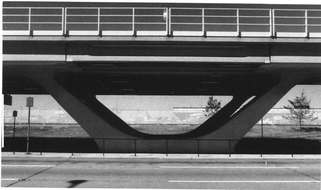
O'Hare Field elevated roadway (photo courtesy of Alfred Benesch and Company)
