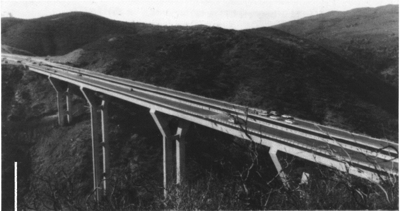
Completed Pine Valley Bridge in California post-tensioned segmental construction
