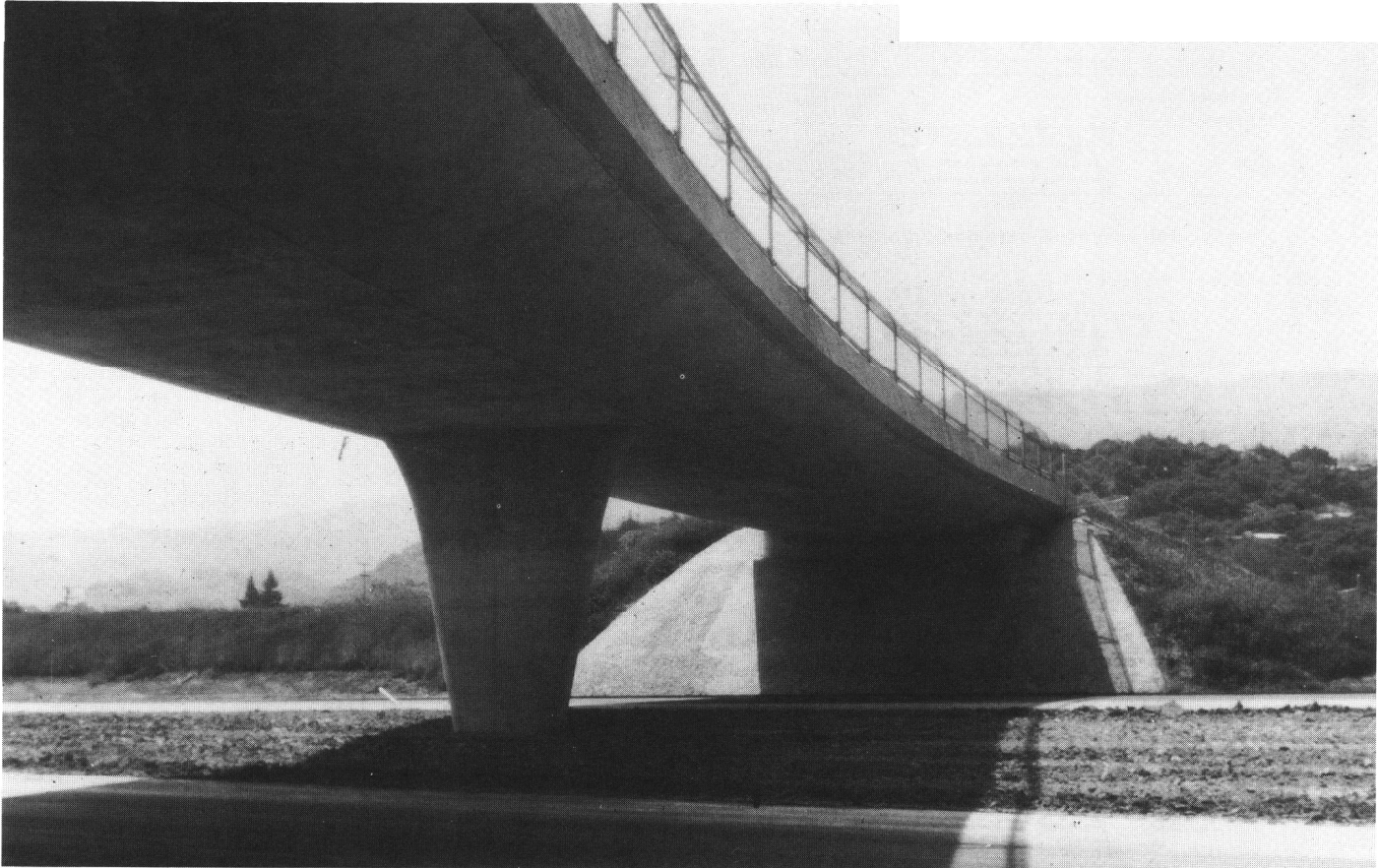
Overcrossing in California with curved alignment and curved soffit (note flared integrated pier and unobtrusive abutments)
