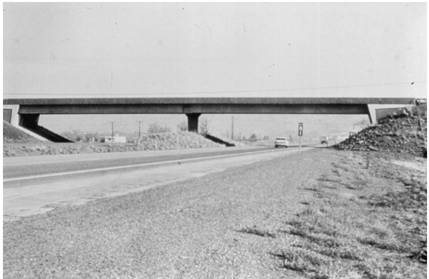
Fig. 2.20 Texture reduces visual mass, I-82 Hinzerling Road undercrossing, Prosser, Washington. (Photo courtesy of Washington State DOT.)
