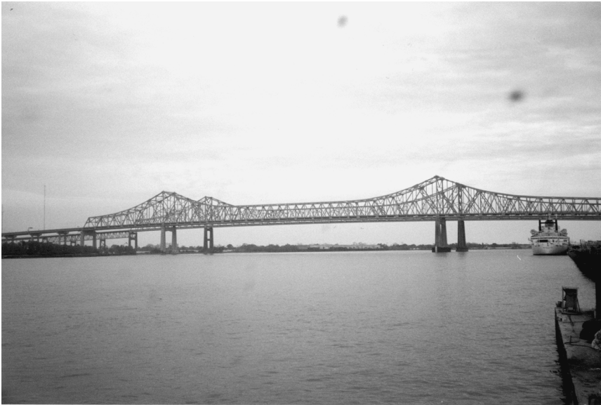
Fig. 2.48 Greater New Orleans Through-Truss Bridge. (Photo courtesy of Amy Kohls, 1996.)
