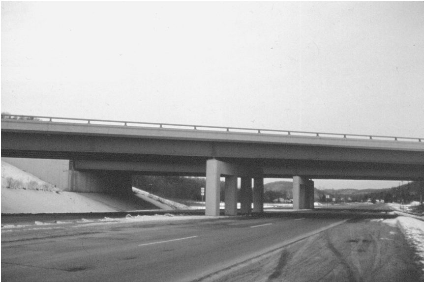
Fig. 2.36 Multiple-column bents. (Photo courtesy of Tennessee DOT—Geo. Hornal, photographer.)
