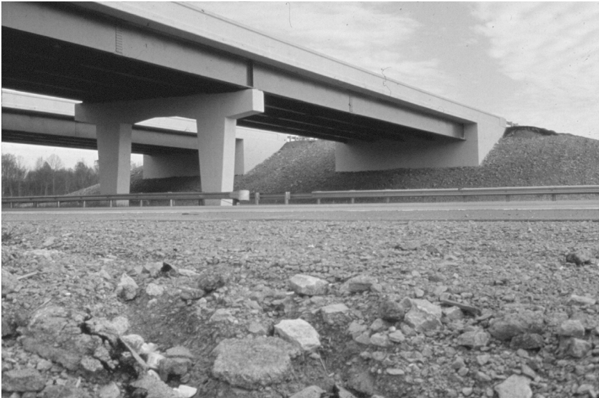
Fig. 2.35 Hammerhead piers. (Photo courtesy of Tennessee DOT—Geo. Hornal, photographer.)
