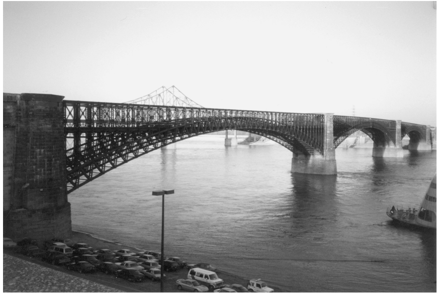
Fig. 1.12 Eads Bridge, St. Louis, Missouri. (Photo courtesy of Kathryn Kontrim, 1996.)
