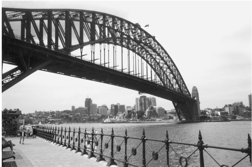
Fig. 2.51 Sydney Harbour Bridge.
