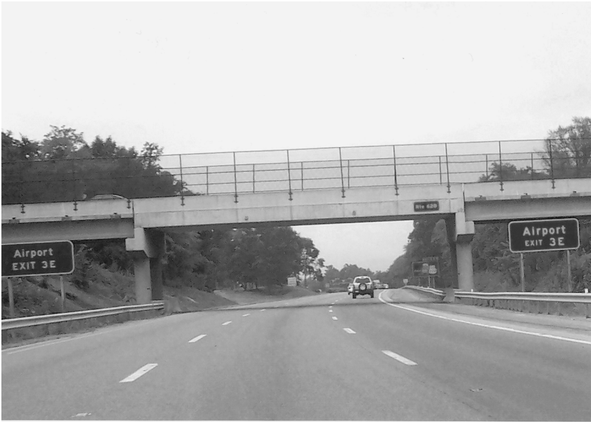
Fig. 2.21 Concrete barrier wall and short-span overpass without shadow: girders look deeper.
