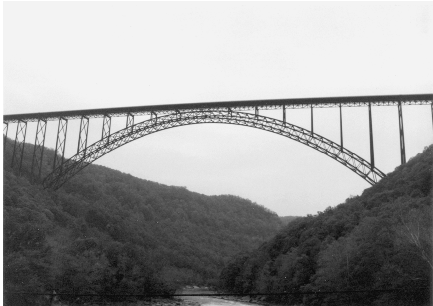
Fig. 2.43 New River Gorge Bridge. (Photo courtesy of Michelle Rambo-Roddenberry, 1996.)
