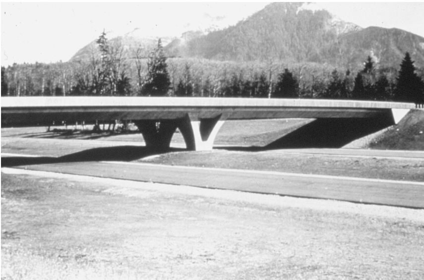
Fig. 2.23 Cedar Falls Road overpass, I-90, King County, Washington. (Photo courtesy of Washington State DOT.)
