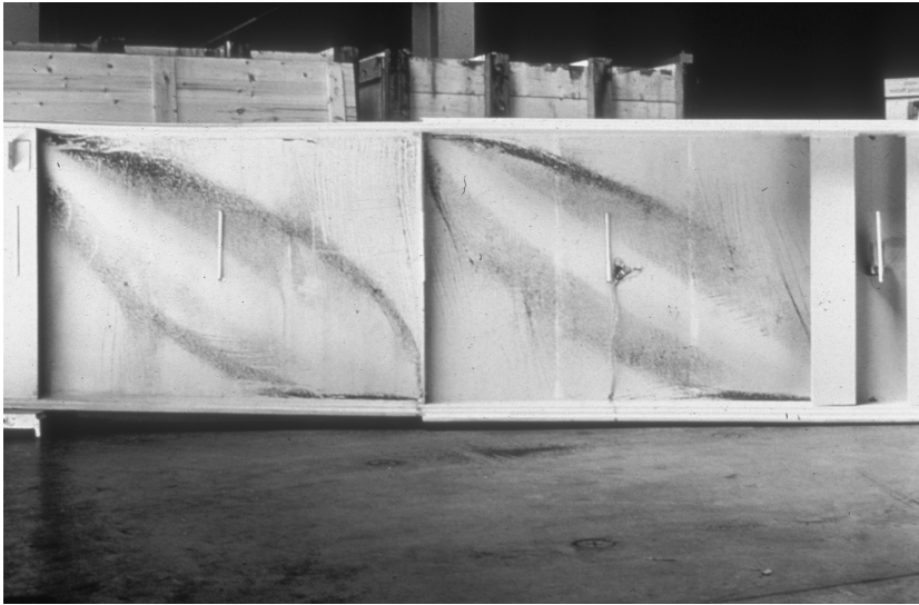
Fig. 8.64 Thin-web girder after testing. (Photo courtesy of John Fisher, ATLSS Engineering Research Center, Lehigh University.)
