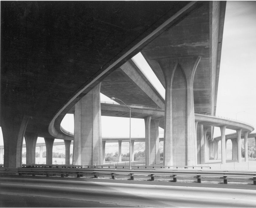
Fig. 2.34 Route 8/805 interchange, San Diego, California. (Permission granted by the California DOT.)
