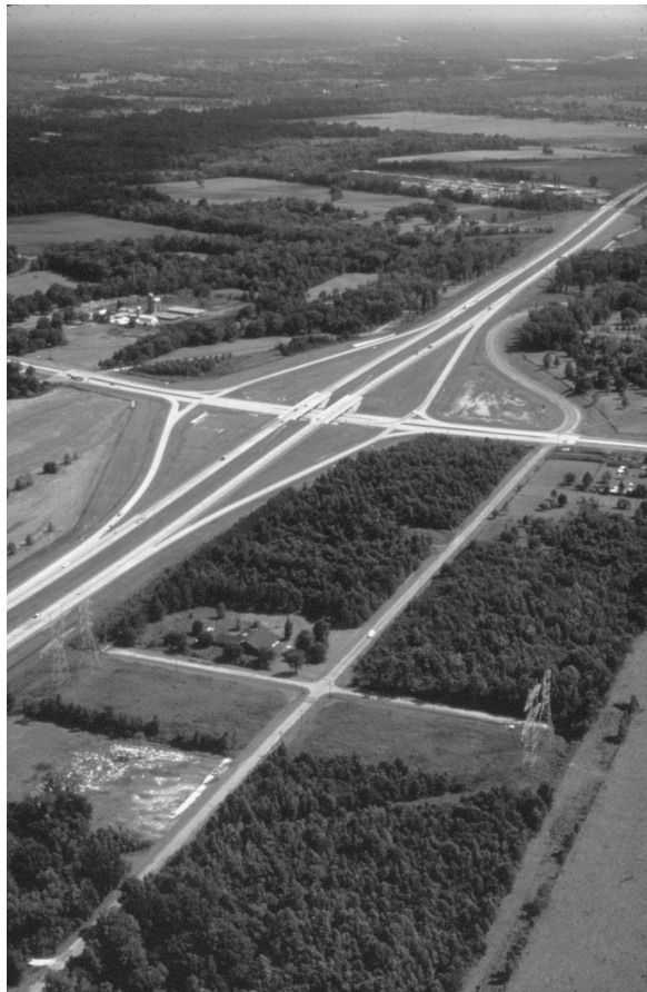
Fig. 3.10 Typical overpass structure. (Courtesy of Modjeski & Masters, Inc.)
