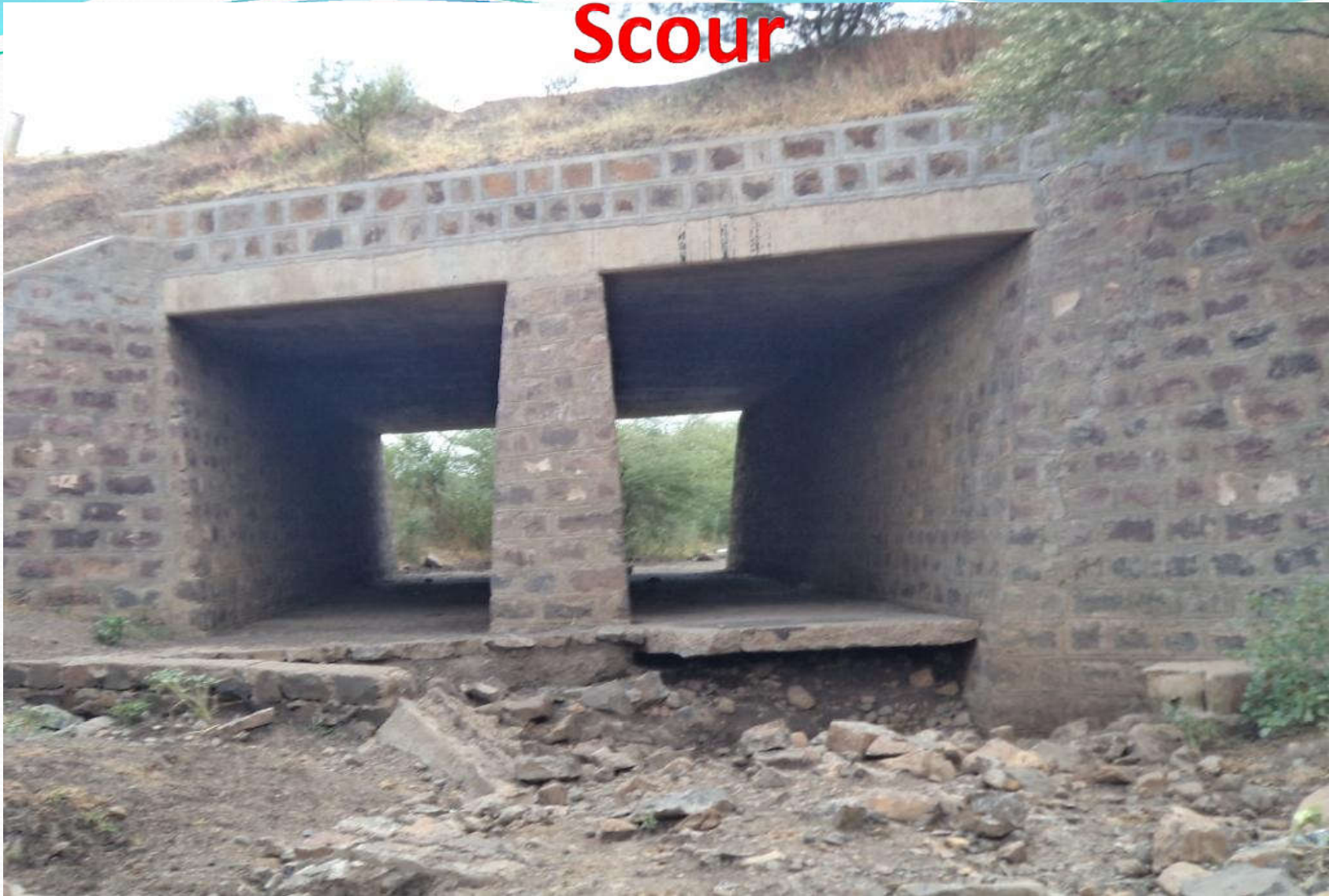
Bridge . No. A1-6-008 along Gewane – Undufo raod segment.
