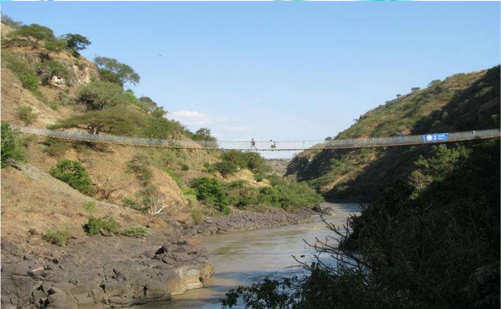
Pedestrian cable bridge over the Blue Nile River in Ethiopia (completed in 2009)
