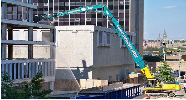
Fig. Long Reach Excavator
