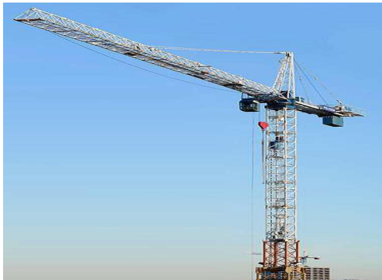
Fig. Tower Crane Rotates on its axis
