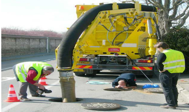
Fig. Cleaning out a sewer manhole
